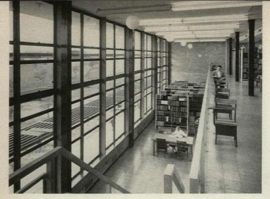
**SOUTH WALL** of library wears three levels of sun shields, braced in place by cables as shown in diagram (below, right).
