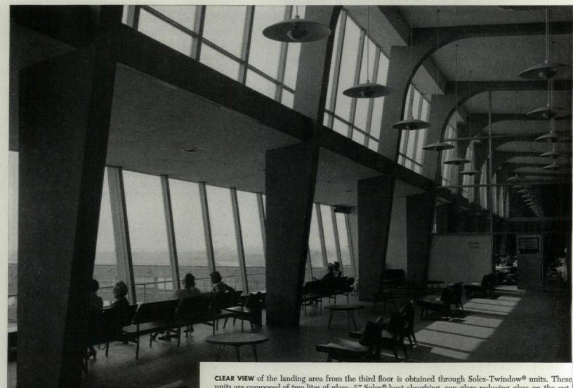
units are composed of two lites of glass-4" Solex® heat-absorbing, sun-glare-reducing glass on the outside, and " polished plate glass on the inside, with a sealed-in air space between them. Solex-Twindow units are noted for their ability to reduce substantially the load on the air-conditioning system; they cut down on room-side condensation, minimize cold air downdrafts.
