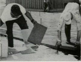
"We also insulated most roofs with FOAMGLAS. Its high strength permits heavy foot traffic, minimizing need for catwalks.
