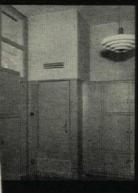
Exterior of corner cabinet containing room conditioner. The two warm air outlets are shown above the woodwork, air return is below access door.
