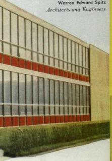
SPEEDS ERECTION. Knapp Unit Wall System is engineered and designed for simple, fast installation. Adjacent units are connected by specially designed sections and hook bolts. Panels are firmly secured to the structural framing with a minimum of time and effort. No construction delays . . . erection can proceed in all kinds of weather. Knapp Wall Panels go up in days instead of months, assuring earlier occupancy of the building.
