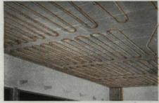
CEILING INSTALLATION ready for plastering. Note tube spacing narrows to  $4\frac{1}{2}$ " c-c nearest the outside walls, and supply lines to panel circuits run next to outside wall.
