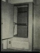
Inside, the compact Janitrol conditioner is completely accessible from the front . . . an outside air inlet supplies combustion air.
