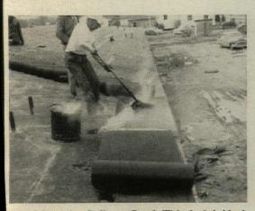
Ideal Base for Built-up Roof. This deck is ideal from two standpoints—a good deck for the roofer to work on—more important, throughout the life of the building, it is an inorganic permanent base for the built-up roof.
