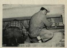
Installing Monel Gutter under expansion bands at the north abutment of the overpass. Monel is easy to bend, cut and weld. Although relatively thin gauge sheet is used (in this case .062"), Monel gutters have ample strength to withstand deformation during installation . . . and abrasion and flexure after installation. Consulting engineers: Brown & Blauvelt, New York.
