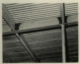
An Economical, Fire-Safe Roof. Finished roof offers maximum in permanence, fire safety. Bright galvanized surface gives lasting protection; affords light reflection when left exposed. However, any normal ceiling treatment may be applied.
