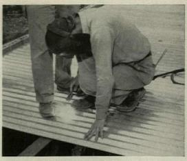
Lightweight High-strength Steel Deck is welded to purlins. Deep-corrugated Granco toughtemper steel has high load carrying capacity. permits wider joist spacing, reduces framing costs.
