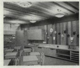
Auditorium, like lunchroom, can be easily shut off from rest of school for public use. Strips of galvanized decking, 16" wide, attach to flat bars imbedded in top face of prestressed beams. Decking is perforated and has sound-absorbent filler.
