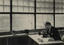
Thermocouples applied to the face of the 80-F block during hot weather (outside temperature 90°) showed that the roomside surface temperature was 14 degrees less than a conventional type light-directing block.
