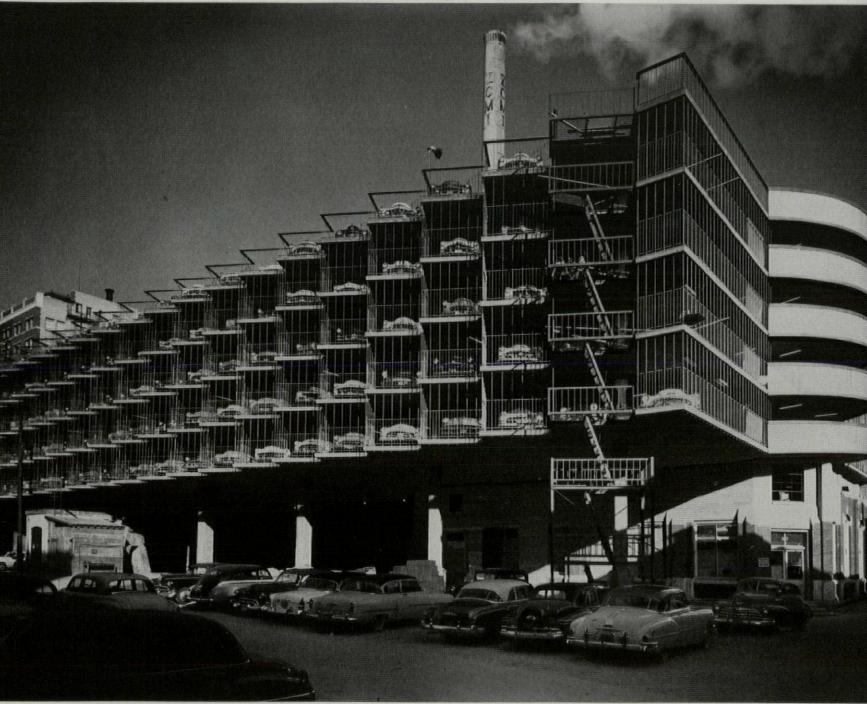
Zigzag floor slabs outline car stalls and cut dead load of parking decks. Railings of continuous 1" rods 12" o.c. will stop a 4,000-lb. car traveling 20 mph; ½" rods 4" o.c. and 4' high are to restrain small children.
