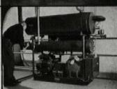
Convectors replace bulky radiators when it is desired to leave existing heating system intact and use transom model UniTrane units for cooling only.
