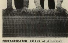
PREFABRICATED ROLLS of American Welded Wire Fabric wound on large mandrels can be unrolled continuously from beam to beam, making installation easy and assuring continuous reinforcing.
