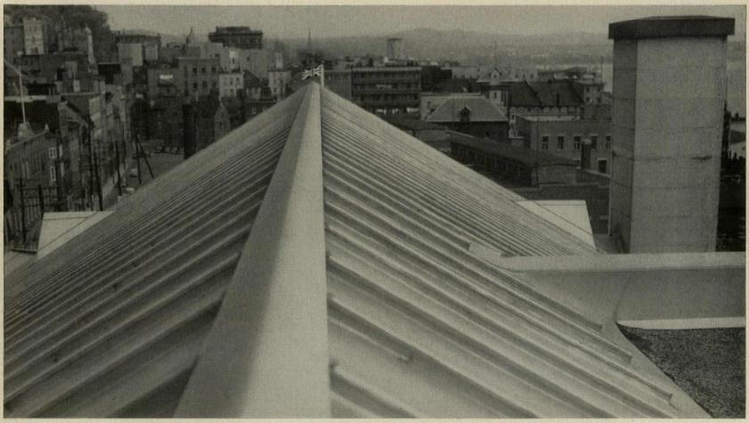
On the waterfront. Over 22,000 pounds of Monel went into construction of the batten seam roof, flashings and 60-inch-wide gutters of the new
