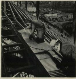
Corruform between Risers. The 100,000 psi steel, pre-sized and stacked, made both concrete base and working platform, kept laying crews well ahead of concreting. Hot-dip galvanized Corruform was vinyl primed for finish paint.
