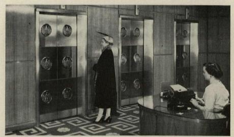
STAINLESS STEEL BECOMES A DECORATIVE TOOL in the reception room, Home Federal Savings and Loan Association. Doors and trim are stainless. The texture effect on the door panels is the result of turning the direction of the polish lines on the middle panels 90 degrees to those on top and bottom panels.
