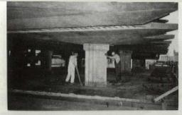
Movable formwork panel, 54' x 60', is lowered 8' to next floor level by . . .
