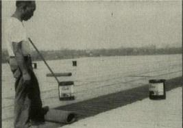
Apply a full 36" wide sheet of Fire-Chex Vapor Barrier, sanded side to deck. Allow 3" side lap, 6" end lap.
