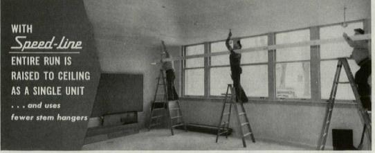
No straining at top of ladders. Simply hook Garcy Stem Hangers into hickeys and then connect house wiring.
