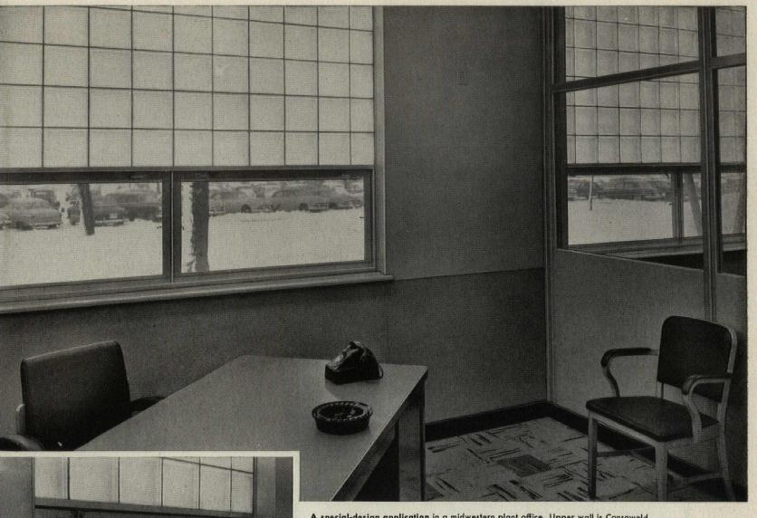
A special-design application in a midwestern plant office. Upper wall is Consoweld 10 in Dusty Green Echo. Wainscoting is Gray Holiday, with Twin-Trim moulding. Movable partitions are faced with Consoweld wood grain in Harvest Brown Birch. Baseboard is a ¾" thick strip of Consoweld, available on special order. Desk top is Consoweld Gray Echo. Wall materials are applied directly over cement block.
