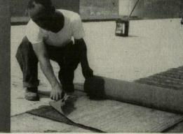
Seal both ends securely with Fire-Chex Adhesive. Continue application, lapping each sheet 3". Now apply insulation and built-up roofing.
