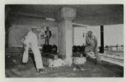
. . . manually operated winches, two to each of panel's four columns.
