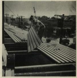
Granco Steel Roof Deck formed concourse roof and decorative curtain wall behind upper-deck rear seats. Wide sheets meant fewer laps, greater roof strength and safety, big time-saving in placing and welding.
