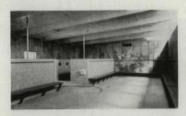
Dressing rooms have high strip windows, washable tile, concrete surfaces. Below: tanks and filters in mechanical building.
