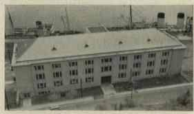
The full picture. Here is an over-all view of the huge Marine Storage Building. For the batten seam roof—and for all flashings—.018" Monel was used. The gutters took .031" Monel—still a comparatively light gauge considering the rigidity required in 60-inch gutters. The sheet metal contractor, Alelard Laberge, Ltd., used Monel cleats and Monel "Anchorfast" nails throughout.
