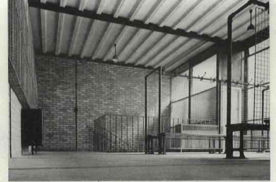
Rawness is typified in ceiling of bare precast channels. Steel beams were sprung for these to be let in, slid to position. All equipment is prefabricated, US style.
