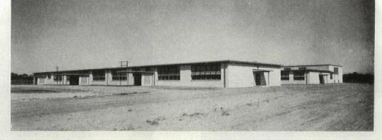
Separate classroom wings of spacious suburban school are heated by small residential boilers, permitting use of short, inexpensive chimneys that do not mar roof lines.
