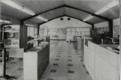
**Spacious clear-span** interior of Butler steel building, handsomely and economically modified, provides post-free space for greatest usability, convenient arrangement of office equipment.
