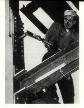
SPOT CHECK is made with manual torque wrench. Only every tenth bolt is checked.
