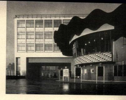
Low wing. Cantilevered canopy, in corrugated outline, has an overhang of 20'. Underside of canopy is painted dark blue-gray and the glass mosaic panel below the control room window is four shades of blue-green.
