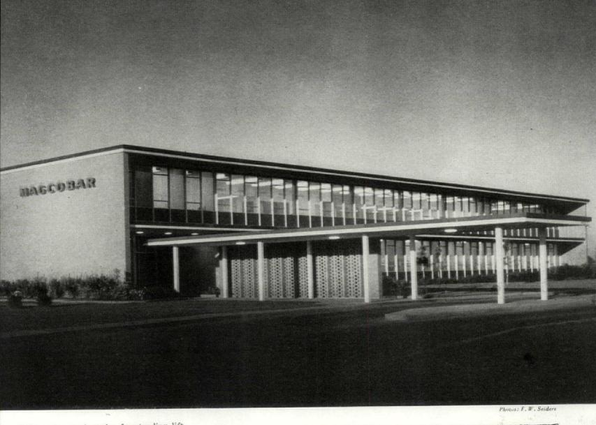
Main entrance is under freestanding liftslab canopy, in front of "corrugated" screen wall of pierced brick. South-facing offices are shaded by 7' overhangs.
