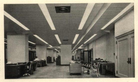
UNION CENTRAL Annex Building, Cincinnati, utilizes some 200 Kno-Draft High Pressure Air Diffusers for quiet, draftless, comfortable air distribution.
