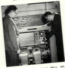
MOTOR-GENERATOR produces 600-v. 400-cycle power. Wiring diagram shows how lines are grounded for 300-v. line-to-ground limit.
