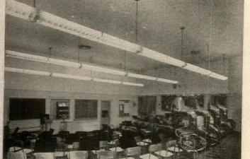
The handsome, Full Random pattern of perforations gives this Cushiontone ceiling an unbroken, monolithic appearance. Armstrong Cushiontone in the music room reduces the reverberation of sound and assures proper acoustics for band practice. Cushiontone can be washed or repainted whenever necessary without losing its high noise-absorbing efficiency.
