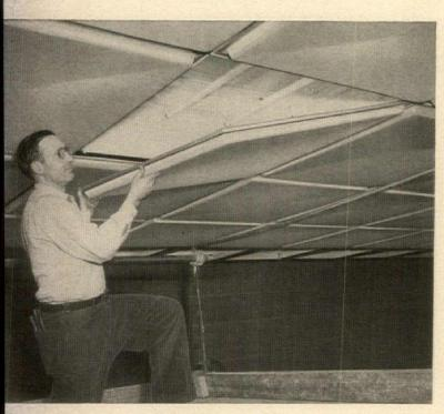
"LUCITE" is readily and economically fabricated to precise tolerances — even broad sections like this 4' x 4' panel. Fixtures of "Lucite" are lightweight for easy assembly, resist discoloration, are durable.
