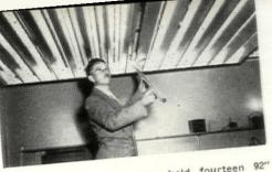
FIXTURES are 8' square, hold fourteen 92" lamps (above) which will be changed every two years under group replacement program. Right above: 400 cycle ballasts are 3-oz. capacitor and 2-lb. choke coil units, both much smaller than the 8-lb., 60-cycle ballasts. Below: only 14 circuits (vs. 84 for conventional lighting system) and two panel boards are used for 198' x 209' area.
