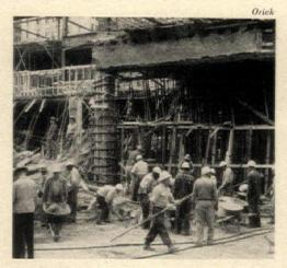
COLOSSAL MESS of reinforcing mesh, duckboards and supporting timbers immediately after Coliseum formwork collapse. Form supports (above), under slab adjacent to collapsed area, indicate how wave of failure spread through falsework. Workers are drilling through fallen slab in their search for body of cement finisher.
