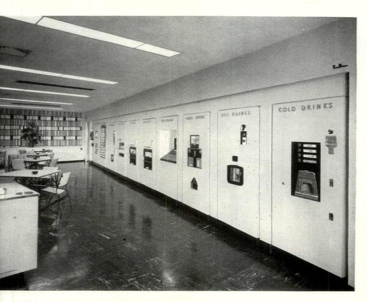
Cafeteria is entirely serviced by vending machines. Service wall is of gypsum block and plaster, with recess left for machines. After installation, machines got 20-mm-thick coat of white plastic spray. Recessed toe space got asphalt tile "baseboard." Two vending machine employees—a manager and a matron—take care of lunch and coffee breaks for close to 1,000 employees. Photo (below) is from curtained "stage" end of room, which can also be shut off with folding wood wall.
