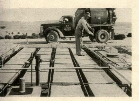
CARDBOARD BOXES are set upside down to raise slab above fill. Cardboard ribs inside boxes maintain shape during pouring.
