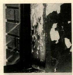
Here's the kind of damage to interiors that driving rain, soaking right through the wall, can cause inside of six months.
