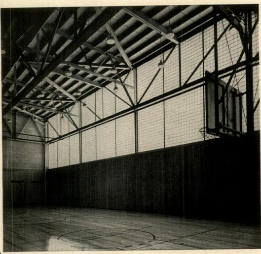
Because Owens-Illinois Glass Block insulate as effectively as an 8" thick brick wall, huge expanses of glass block are practical even in a cold climate.
