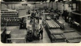
Panels are completely prefabricated in the Rippel company's modern, well-equipped Chicago plant and are installed by Rippel's own expert construction crews.
