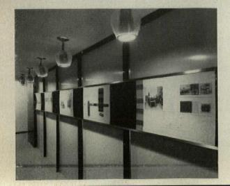
Executive corridor is formed by glass partition set in black wood frame on one side (above) and on other (left) by partition of gray and white panels of plastic-coated plywood set between 2' x 4' walnut posts. Flexible displays are carried by brass brackets. Brass and amber glass lighting fixtures of special design are swivel aimed at display. Carpet is gray. Ceiling is striated acoustic tile.
