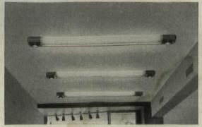
Neat Plaster Ceiling over Fire-Safe Tutcor. Any normal ceiling treatment is easily applied to Tufcor. Its attractive galvanized surface is sometimes left unfinished when light reflection is wanted.
