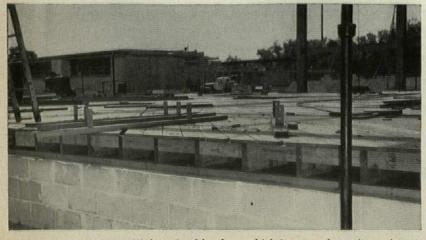
IN THE GYMNASIUM: Wolmanized lumber, which is rot and termite resistant, was specified exclusively for the Gymnasium sub-flooring, furring and joists.
