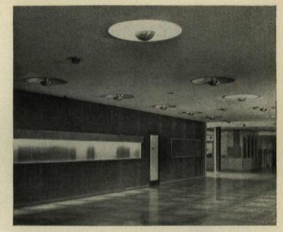
Easily cut and fitted to any shape, Armstrong Travertone is readily installed with lighting and ventilating fixtures. In this school lobby, the Travertone ceiling soaks up the sounds of footsteps and voices, prevents them from bouncing off the many hard surfaces and building to disturbing noise levels.
