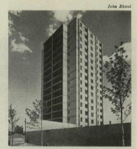
High-rise building in public housing project is one of three nearing completion, along with surrounding two- and three-story buildings. Balconies double as windbracing for structural concrete T's. Louis I. Kahn, Louis E. McAllister and Kenneth Day, associated architects.
