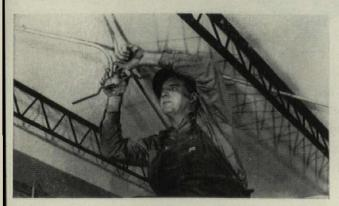
REPUBLIC ELECTRUNITE® ELECTRICAL METALLIC TUBING passes easily through the open web of steel joists. Every coupling is a union—no lines to turn. ELECTRUNITE E.M.T. is Republic's lightweight rigid steel raceway that protects wiring circuits against fire, moisture and mechanical injury. It's inspected by Underwriters' Laboratories, and approved by the National Electrical Code for exposed, concealed and concrete slab construction.
