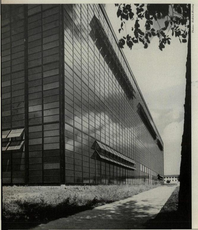
Awning sash at two levels opens up, and blowers atop the roof pull fresh air through the building, helping to counter a heavy sun load. Translucent heat-absorbing glass is frosted inside to diffuse light, maintain security, blank out distractions.
