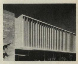
Vertical metal louvers, available in a number of widths and designs, are now made on West Coast. Fins are adjustable to various angles, provide best protection on east and west sides of building. Architect: Richard J. Neutra.
