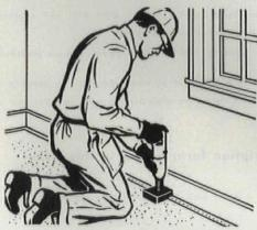
Carpet gripper anchored to concrete
