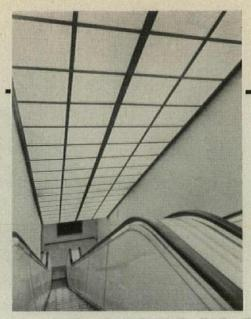
Hutzler Bros. Dept. Store, Baltimore, Md. Photo shows use of Alumiline Framing Sections in pre-fabricated ceiling panels. James R. Edmunds, Jr., Architect. Consolidated Engineering Co., Inc., Contractor. Furnished and installed by Southern Plate Glass Co., Balto, Md.
