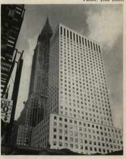
Chrysler building annex, has solar load pattern similar to that shown above, modified by rectangular shape. White brick walls help reduce air-conditioning peak load and operating cost to what is probably record low for a postwar Manhattan office building.
