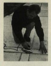
Joints were closed with metal batten, adhesive and plastic cloth. Joint seems to be good where ironed but adhesive is messy, gathers soot during preliminary drying, so better methods are being developed.
