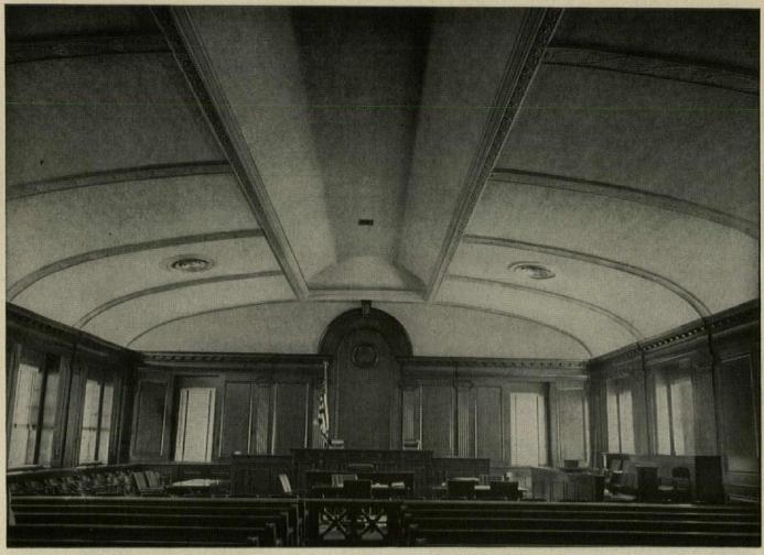
FOLLOWS CEILING CONTOUR. Because this material is sprayed on, original ceiling designs are retained without change, as the courtroom shown above demonstrates.
