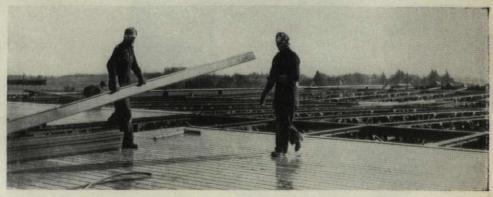
ROOF THE JOB WITH TRUSCON FERROBORD® STEELDECK. Clip or weld Ferrobord directly to Truscon Steel Joists. It comes in lengths long enough to span three or more purlins, roofs large areas quickly . . . flat, pitched, or curved. Exclusive Truscon design allows full-length interlocking, gives greater strength. Installs from the top; no scaffolding required. Write for specifications.
