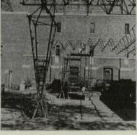
site, was swung onto pedestal with ropes and pulleys, then anchored to roof framing.
