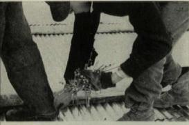
Steel Sheets Are Quickly Clipped to the steel framing. Welding is equally fast. Positive attachment of tough-temper sheets adds rigidity to roof framework.
