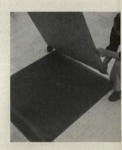
Sub and finish flooring are both installed as panels. Asphalt-felt (automobile body sound deadener) goes over bottom asbestos cement panel. Finish tiling is cemented to thin upper asbestos cement panel, screwed down at corners.
