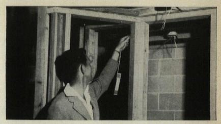
IN DRESSING ROOMS: Architectural Inspector checking an effective use of Wolmanized lumber in framing for a three-way mirror.
