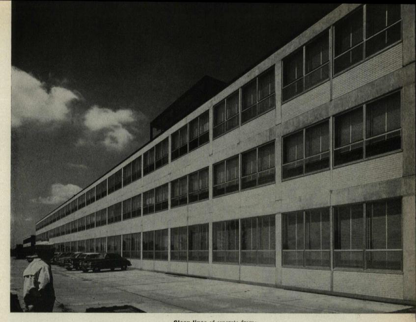
Clean lines of concrete frame are expressed on exterior, filled with brick panels, precast concrete mullions, aluminum window sash.
