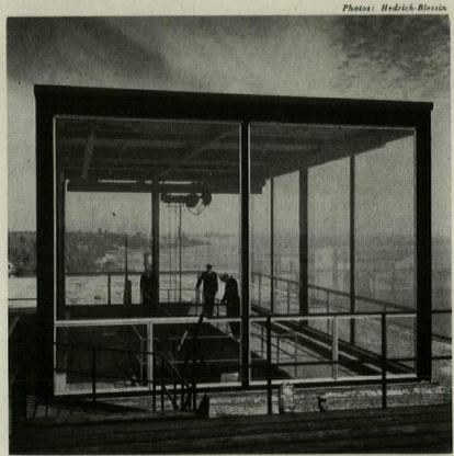
Periscopes are assembled on ground floor, hoisted through three floors to this cleanly detailed observatory for testing. Tops of scopes are guided through slots into collars.
