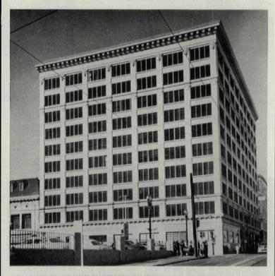
LOS ANGELES COUNTY ENGINEERS BUILDING. The KoolShade Sunscreen installed on this building reduced, by 79 percent, the solar heat gained through glass . . . cut air conditioning requirements by 72 tons.
