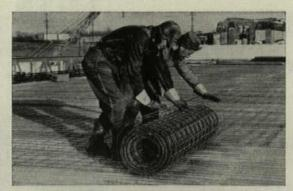
An Immediate Safe Working Deck is obtained as soon as Tufcor is attached, Light mesh is added for shrinkage control of the lightweight insulating concrete.
