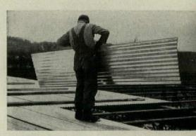
Handles Easily, Places Fast. Tufcor arrives pre-cut to building size. Measuring and cutting is eliminated. Two or three men can place up to 10,000 sq. ft. a day.
