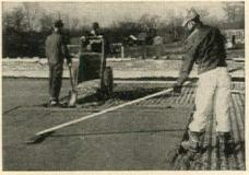
Permanent, Fire-Resistant Roof Deck is formed by cast-in-place slab. A strong bond forms between galvanized steel sheet and lightweight concrete fill giving high-strength rigidity to finished deck.
