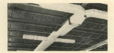
A large section of heating and cooling ducts insulated with L·O·F Super·Fine. Ducts were coated with adhesive, then wrapped around with Super·Fine and secured with light-gauge wire.
