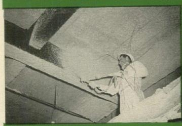
Membrane fireproofing of beams and girders is machine applied. Modern plastering machines move lightweight-aggregate plaster up to a distance of 75 feet for fast, uniform application.
