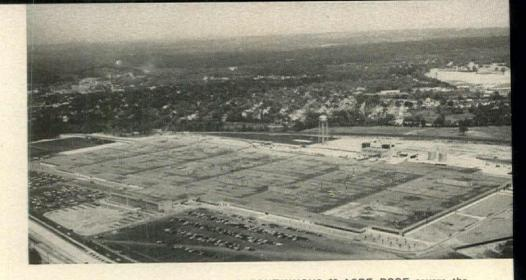
A CONTINUOUS 39-ACRE ROOF covers the 1,700,000 sq. ft. Ford assembly plant at Mahwah, NJ., believed to be the biggest roof area ever built. Architect: L. Rosetti; engineers: R. F. Giffels & V. E. Vallet.
