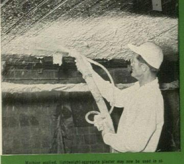
Machine applied, lightweight-aggregate plaster may now be used in almost any type of building, bringing costs of the finest interior surfacing well within those of lesser materials.
