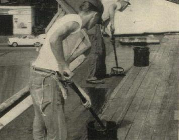
Perma-Topp being applied over wood deck after removal of old roofing. The 1st ply has been applied and 2nd ply is being started.
