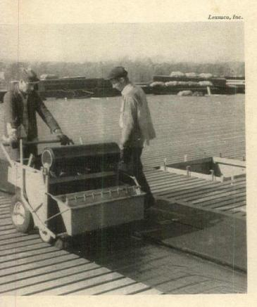
PLASTIC VAPOR BARRIER used atop a metal roof deck at this new General Electric plant does not add fuel to a fire breaking out in the building below.
