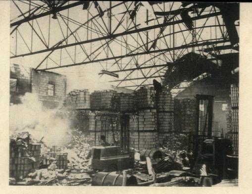
EXCESSIVELY HIGH STACKING rendered the sprinkler protection inadequate in this warehouse fire.
