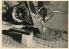
Insulating Concrete Placed on Tufcor is fast operation. On an average roof construction, this material weighs less than 6 pounds per square foot.
