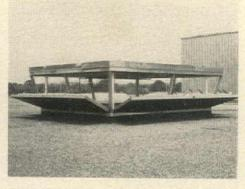
SNAPPED OPEN, side panels fall to end of wires, giving a 41/2'-high vent opening.
