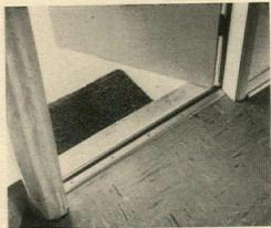
FLEXIBLE THRESHOLD hugs floor and door for air-tight seal
