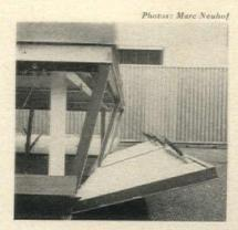
SIDE PANELS ARE INSULATED, are fitted with springs to absorb shock of opening.
