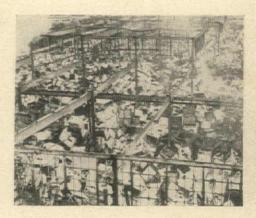
EXCESSIVELY DENSE STORAGE of valuable kitchen appliances caused a total loss of this unsprinklered "noncombustible" building.
