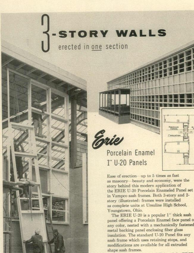
panel offering a Porcelain Enamel face panel of any color, nested with a mechanically fastened
