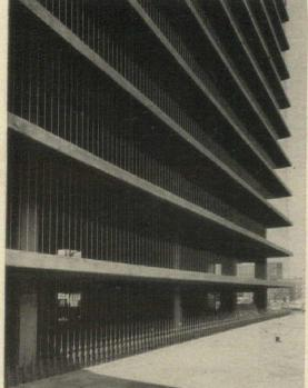
FUNCTIONAL yet strikingly good looking, this new Municipal Parking Garage in downtown Chicago, features pan and slab roof construction with American Welded Wire Fabric Reinforcement. All floors which must withstand heavy loads are also reinforced with American Fabric. Specify American Welded Wire Fabric for all your concrete.
