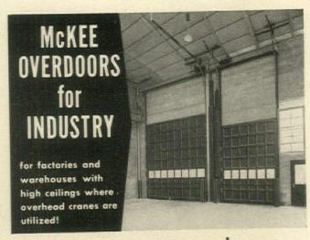
Shown above is an installation of two McKee Vertical Lift Overdoors. These doors required special engineering to follow the contour of the roof, and still give clearance for the overhead crane rails.
