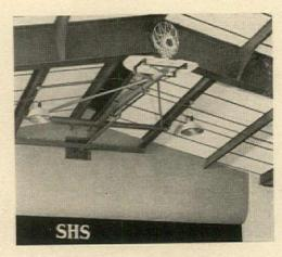
fold backward and the two backstop units, forward, raising up in about 40 seconds and coming down just as fast. One ¼-hp motor wired to a reversing switch operates all four. The forward-folding goal's lifting cable is 10′ above the basket, and cannot interfere with play when in use. Prices on the backstops (based on 16′ truss spacing) including winch and cable start at \$65 a unit and go up to \$467, depending on beam height and type of suspension.
