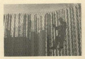
Wall area using a combination of STEELCRETE and bars to obtain desired reinforcements. Produced in  $3'' \propto 8''$  diamond shape, STEEL-CRETE offers up to  $1\frac{1}{2}$  sq. in. of area to the foot of width.
