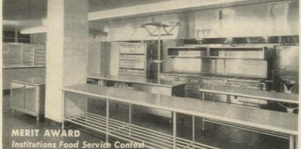
COOKING SECTION, MAIN KITCHEN: Food conveyor traffic flows rapidly around this section in a counter-clockwise direction. Ample work surfaces are provided by the generously-proportioned cooks' tables. Note seamless work tops, rounded corners, welded tubular undershelves.
