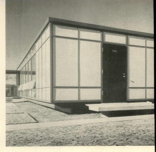
**Exterior wall** combines steel sash with intermediate projected windows. Opaque panels are abestos-cement board.
