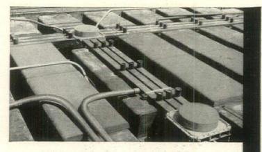
Here's a partially completed 3-duct system. The electrical ducts are installed on top of Ceco-Meyer Removable Steelforms. Concrete is poured over and around ducts. Result is monolithic floor system—no fill needed.
