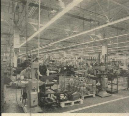
Day-Brite CFI-10 (Comfort For Industry) with 10% upward lighting. Ceiling contrasts are washed out and greater visual comfort assured.
