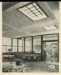
The combination of light-directing glass block and vision strip keep brightness at comfortable levels, provide vision and ventilation.
