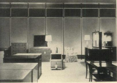
In this department store it was desirable to partition off the furniture section. The high ceilings posed a problem easily solved by UNISTRUT Partitions. Standard panels of wallboard were used with additional panels at the top. Should change in the department be necessary, the partitioning may be easily moved.
