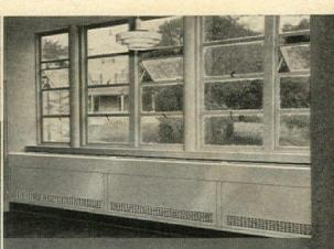
This Milcor multiple Wall Unit enclosure has a flat, perforated stool and perforated front panel.
