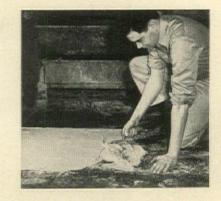
job and handled like regular concrete or mortar. It may be troweled or buffed to a smooth finish. Its rubber content makes the cured composition so flexible that a long thin strip can be bent by hand into a hoop. The surfacing's special cement gives it excellent bonding to almost any clean hard surface: *Laticrete's* grip on masonry is 300 lb. psi. It will also adhere to metal, and to glass for a pull of 100 lb. psi.
