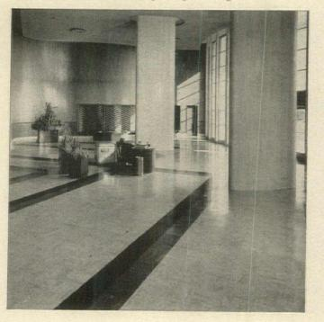
Elaborate custom styling such as in this floor of Armstrong Linoleum requires intricate cutting and fitting. The labor involved can add considerably to the cost of the installation.
