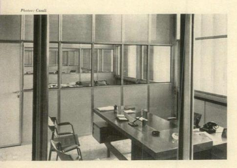
Interior partitioning, all demountable, is made of aluminum sheets, connected to each other and to ceiling with rubber joints, under pressure. These partitions are of three types: opaque panel, glass panel in center; glass panel near ceiling. Special study was made of acoustical problems. Decibel losses were figured at standard room noise level of 70 db., for three partition types are, respectively, 18 db. absorption, 20 db. and 18 db.
