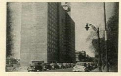
Midway Gardens Apts., Chicago. One of hundreds of successful Plaster-Weld installations. In this case, Plaster-Weld was used to permanently band lime-putty coat directly to all concrete ceilings and columns, Archts.: Holabaird, Root & Burgee & Associates; Genl. Contr.: S. N. Nielsen Co.: Plstg. Contr.: McNulty Brothers Company. Many other examples of Plaster-Weld applications gladly sent on request.
