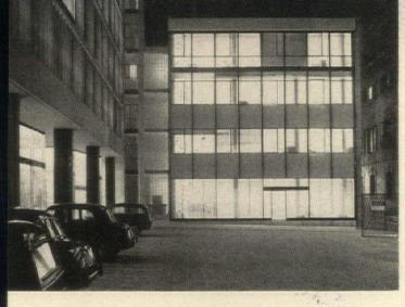
Low office wing by side of piazza. Except for lower floor of main building, left, and double basement, entire structure is offices. Piazza paving is underlaid with network of pipes through which heated antifreeze is circulated in winter to melt snow.
