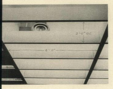
components and can be moved overnight by the insurance company's own maintenance staff. It consists of aluminum posts mounted 6' o.c. in sockets in the open ceiling and in the floor, and carries 6'  $\propto$  7' translucent glass or core filled plastic.
