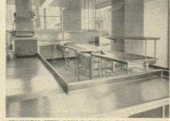
STAINLESS STEEL DISH TABLES in dish pantry. Work top and raised rolled edges form a continuous, crevice-free surface to assure maximum cleanliness.
