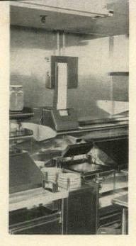
2. Order, transmitted by wire, appears simultaneously on roll of paper in kitchen. Grille below is for hot snacks; full hot meals are elevatored up from another cafeteria kitchen.
