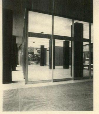
**Exhibition space** on first floor is flooded with light from egg-crate ceiling. Columns are sheathed in black and white anodized aluminum.
