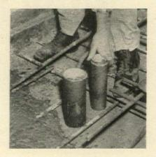
closure. The other metal end is then inserted in the top of the sleeve and anchored to the form to hold it straight. After the concrete sets, closures are knocked out leaving a neat opening for pipe or conduit. Where sound insulation is important, the sleeve itself can be left in. Sonopipe in the 4" size runs about  $18\phi$ per ft., FOB factory, and metal ends to fit that size are  $6\phi$  apiece.
