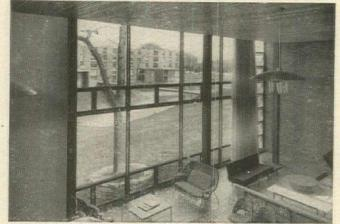
CONTEMPORARY DESIGN AND TRUSCON STEEL WINDOWS work hand in hand to allow skillful use of wide, sweeping expanses of glass. These windows made by Republic's Truscon Steel Division, also help provide controlled ventilation and seal weather out or heat in. Here is how Saarinen & Saarinen & Saarinen, Architects, Detroit, Mich., used Truscon Intermediate Projected and Donovan Steel Windows at Drake University, Des Moines, Iowa.
