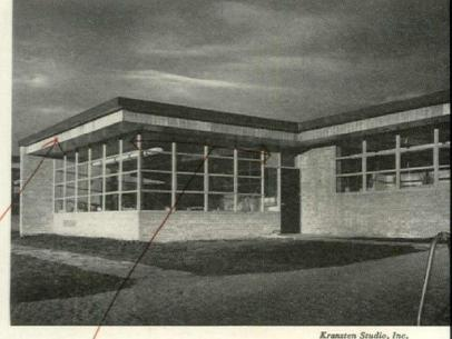
and south. /Even though overhangs do not interrupt sun, especially on west, they do cut sky glare. Alternative suggested by hindsight (which can be another job's foresight) is eliminating top panes. Empirical support: Where Venetian blinds are used in old wing they are usually kept to this point anyway (see opposite page, bottom), and in some cases upper panes have been painted.
