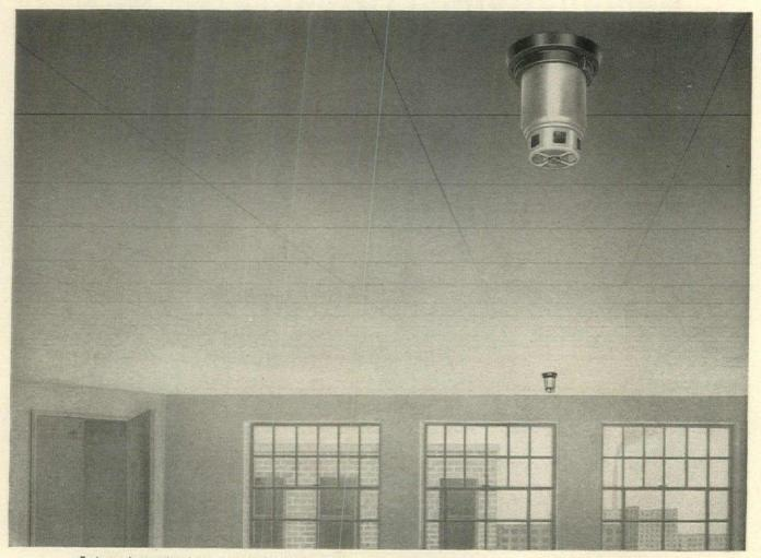
Each pre-detector head protects up to 3,600 square feet of area...harmless radio-active element utilizing ionization chamber principle quickly detects all forms of fire...requires only simple two-wire circuit and insignificant wall space for controls.
