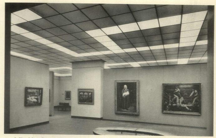
In this painting gallery at the Whitney Museum, the panels of Alba-Lite are dimmed to show the location of the Fota-Lite panels. Louvers are photographically produced in Fota-Lite to transmit light at a 30° angle in this installation. Direct illumination on vertical surfaces at eye level totals 65 foot-candles. Fota-Lite also comes with louvers designed for 45° cutoff.
