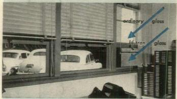
Houze Lo-Tran vision strips in window completely eliminate glare which exists through clear glass window where arrow is pointing. Bright sunshine has completely "washed out" the red brick visible through the Houze view strips.
