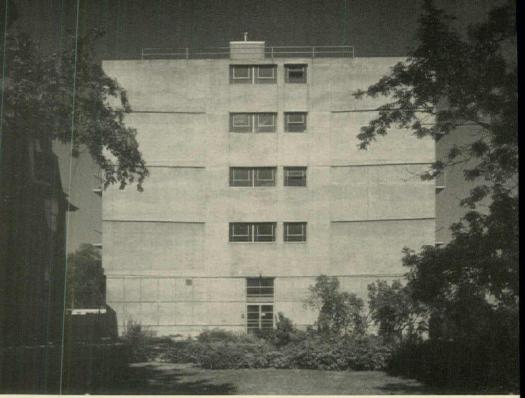
CANTILEVERED FLOORS are expressed with offsets on the solid concrete end walls.
