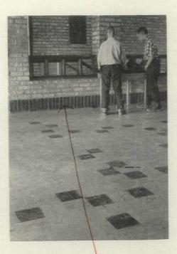
**Lobby wall's** dark soldier courses have made splendid base, show no staining above lowest 4" and that not objectionable. Asphalt tile flooring throughout school has needed no replacement, is in best of condition. Wall is same brick as exterior but exterior has weathered to redder cast.
