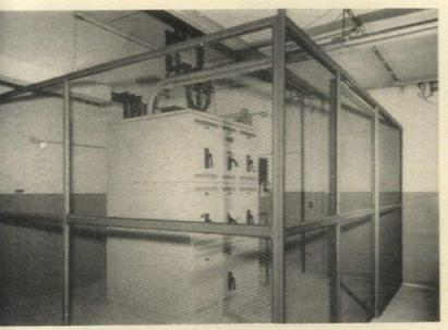
Here is a good answer to the problem of enclosing a switch control room, a tool crib, a parts department or other factory area where safety, privacy or security are important. Expanded metal is only one of the many materials that may be used with UNISTRUT Partitioning.
