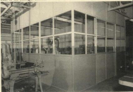
UNISTRUT Partitions are ideal for industrial use such as shown above. They provide privacy where desired and freedom from excessive noise. Any desired arrangement of windows and doors is possible and the partitioning may be easily moved with no loss in material.
