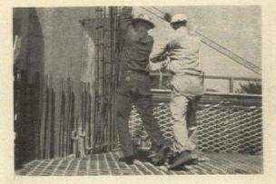
Heavy STEELCRETE reinforcing mesh in floor can be used as a working level until concrete is poured. No special catwalks or temporary "bridges" for concrete buggies are required.
