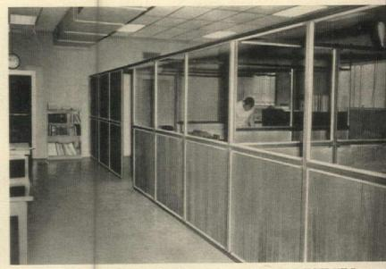
In this handsome office a walnut faced plywood is used in the UNISTRUT Partitioning. The partition shown utilizes standard size plywood panels. UNISTRUT Partitioning may be used as 7-foot office dividers, 8-foot partitions or extend clear to the ceiling if desired.
