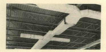
A large section of heating and cooling ducts insulated with L·O·F Super·Fine. Ducts were coated with adhesive, then wrapped around with Super·Fine and secured with light-gauge wire.
