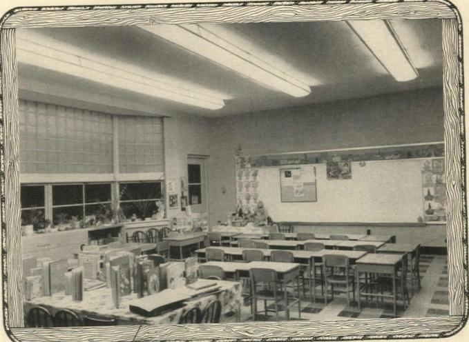
INSTALLATION: North Coventry Township School, Pottstown, Pennsylvania. DESIGNED BY: Eastern Engineering Co., Reading, Pennsylvania. AREA: Lower Grade Elementary Classroom 24' x 30'. CEILING HEIGHT: Approximately 9'-6". FIXTURES: 15 - Litecontrol No. 9224 surface mounted, using Holophane No. 9100 CONTROLENS<sup>#</sup> SPACING: 8' -0" on centers.
