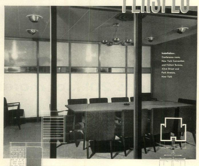
Interior designed by Michael Saphier Associates, Inc. using "PERSPEC" with black recessed steel base at floor carrying electric wires; lower panels 3/811 steel with white factory finish; upper panels 1/2" milk translucent glass; horizontal brass strip.
