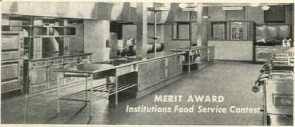
GENERAL VIEW OF MAIN KITCHEN — showing food conveyors lined up opposite cook's tables. When loaded, conveyors are wheeled to elevators and taken to individual floor pantries. Stainless steel cook's table typifies sanitary construction of all equipment, featuring round corners, rolled edges, seamless crevice-free surfaces. Note built-in bain marie.
