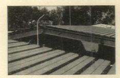
PANELS are laid over the rigid steel frame during course of erection, combining in one unit acoustical ceiling, joist and deck. Be sure to investigate before you plan your next building! Once your building is started, it's too late!
