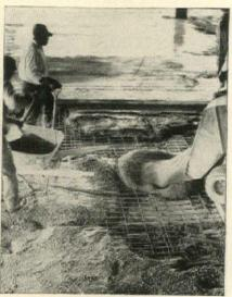
1 floor every 4 days—Fast Cofar construction helped to make up 60% of an 8-week delay. Concrete pours were made in 4 days per floor, more than 50% faster than with ordinary forms. Tight laps between Cofar units kept wet concrete from leaking.
