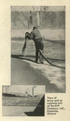
SURCO, cement and aggregates are here being applied by the pneumatic method to resurface and waterproof a brine tank. Deterioration of the concrete was repaired and water seepage stopped by this economical and fast application of SURCO. Coating varied from  $\frac{3}{8}$  to  $\frac{1}{2}$  inch in thickness. SURCO is being applied on many other jobs by conventional hand methods.
