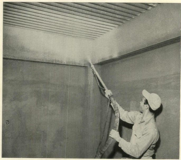
Only 18 Days From Start to Finish! Averaging 3000 sq. ft. per day, workmen spraying 3 coats of acoustical plastic on Cofar completed each floor in only 3 days—the entire job in 18 days!
