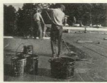
Lower left, perlite-cement grout fills joints. Lower right, unlike poured roofs which must dry before application of built-up roofing, Tectum may have roofing applied as it is laid.
