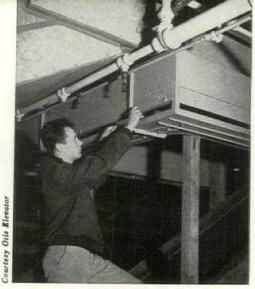
VENTS AND SPRINKLERS are combined to prevent stack of moving stairways from becoming a smoke stack. Fresh air is admitted at top of wellway to further control fire and fume.
