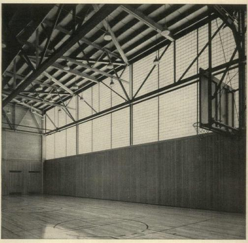
Because Owens-Illinois Glass Block insulate as effectively as an 8" thick brick wall, huge expanses of glass block are practical even in a cold climate.
