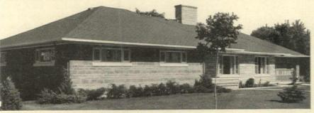
Vibrapac block constructed home. Note unusual effects created by using 4" and 8" high block.
