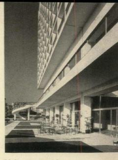
Dining room and bar survey garden through walls of glass. Note expansion joint which runs up columns and overhangs, dividing hotel in half as earthquake precaution.
