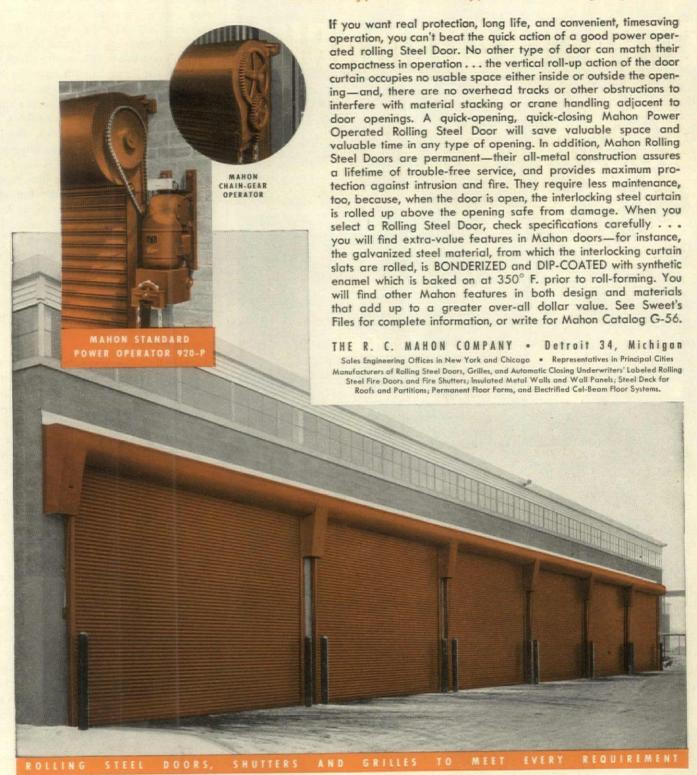
Six Mahon Power Operated Ralling Steel Doors installed in truck openings of a loading dock in the new plant of Sutherland Paper Co., Kalamazoo, Mich. Miller-Davis Company, Designers and General Contractors. A total of thirty-nine Mahon Rolling Steel Doors were installed in various types of openings in this plant.
