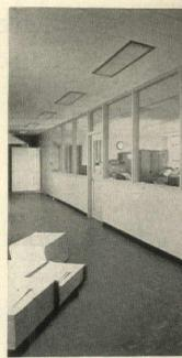
Ceco Hollow-Metal Doors are used throughout the building, in borrowed-light partitions and in separate openings, as shown in these two pictures.
