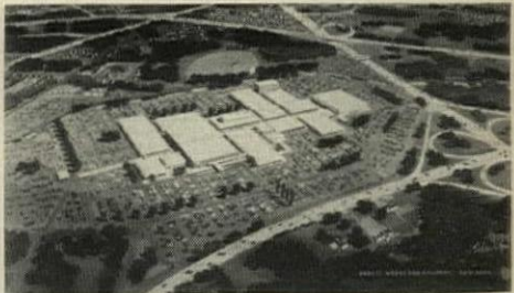
GARDEN STATE PLAZA Shopping Center, Paramus, N.J. Heating load 16,000,000 B.T.U. per hour, present capacity 90,000,000 B.T.U. (with standby). Longest pipe run about 1,250'. Architect-Engineer: Abbott, Merkt & Co. Gen. Cont.: Joseph L. Muscarelle. Heating Contractor: Frank A. McBride.
