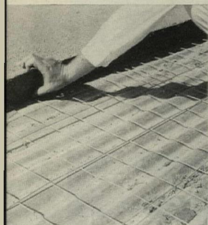
Permanent cast-in-place slab. The lightweight insulating concrete fill forms a strong bond with the galvanized TUF COR sheets. The result is a rigid permanent slab with low dead load and high insulating value.
