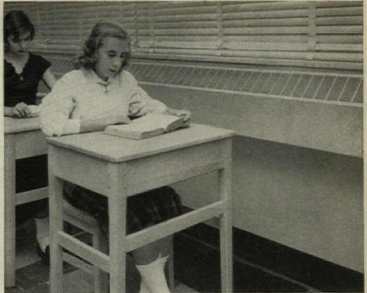
Dunham Sloping Top FIN-VECTOR Radiation extends full length of schoolroom, under windows to eliminate chilling effects of harmful and uncomfortable downdrafts.
