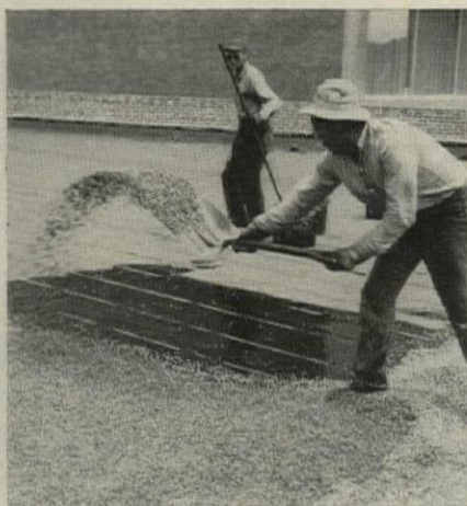
Perfect roofing base. TUF COR deck and concrete slab offer a firm, inorganic, permanent base for the built-up roof. It is not necessary to apply roof immediately. Allow the concrete slab 5 to 10 days for curing.
