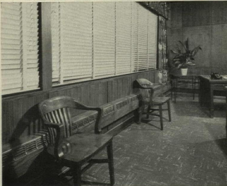
Dunham THERMO-VECTOR Radiation , painted to simulate wood paneling in modern office building. Runs full length along outside walls at any height above 4 in., minimizes wall streakage.
