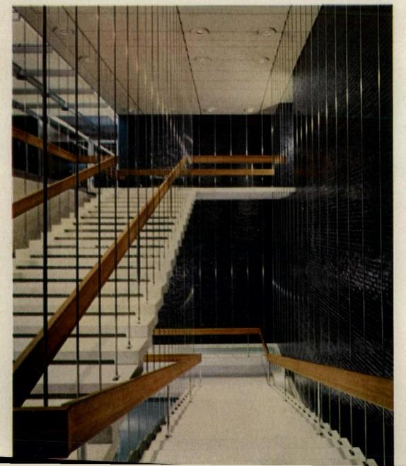
Staircase in Styling Section's administration building is suspended on stainless steel rods over flowing pool cut into travertine floor. Panel ceiling of plastic diffusers in this lobby (right) also contains wiring and air-conditioning outlets, and is typical of the integration of services in the GM design, which has already produced custom prototypes for a number of building elements in mass production.
