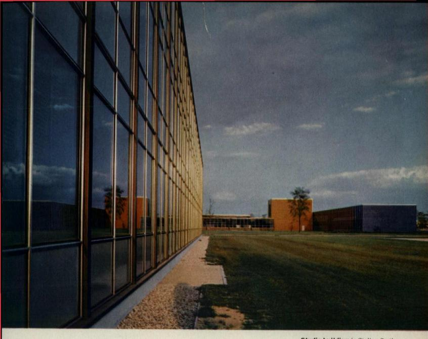
studio building in Styling Section has typical GM wall with steel structure, aluminum frames and plastic gaskets hugging slick glass or porcelain filler panels. Blank end panels of building are filled with glossy bricks in burning colors, another pattern in materials set by Saarinen & Associates in the design of this group.
