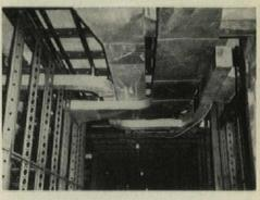
STRUCTURAL FRAME is light steel system formed from sheet stock. Like foundation (see text) frame had been well tested in other building types but never before applied to hospital construction.
