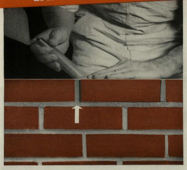
GOOD workmanship is one of the most important factors in preventing leaky brick walls.
