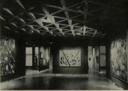
Paintings are exhibited here on remarkable "pogo stick" panels. Easy to install and remove, they provide completely flexible partitioning. Used singly or in groups, they may form the entirety or partial background of a show.
