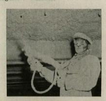
"To fireproof the steel in the Prudential Building, Zonolite vermiculite plaster is sprayed on by machine. Extremely light in weight, vermiculite plaster saves tons..."
