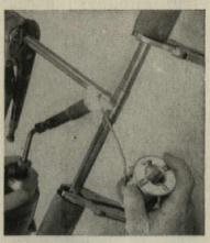
A self-extinguishing material, new Armaflex will not support combustion and may be slipped in place over copper tubing and held back with clamps while sweat fittings are made.
