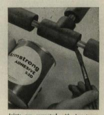
Joints are cemented with Armstrong 520 Adhesive. This easy-to-handle adhesive furnishes a tight, vaporproof bond. No other sundry is required on an Armaflex pipe covering job.
