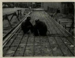
The snow melting system being installed. All 3/4-inch lines and 2-inch headers were of NATIONAL Steel
