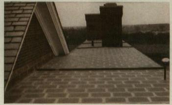
16" x 18" Copper "pans" of easily soldered copper were permanently applied on the horizontal section of the roof. Note expansion joints.
