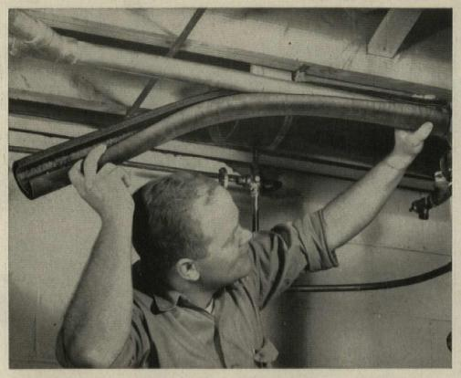
Fast, easy-to-apply Armaflex pipe covering can be slit lengthwise, snapped in place, and sealed with Armstrong 520 Adhesive on lines already in operation. If applied at the same time as piping is being installed, Armaflex can be slipped on, readily follows bends in copper tubing without cutting or fitting.
