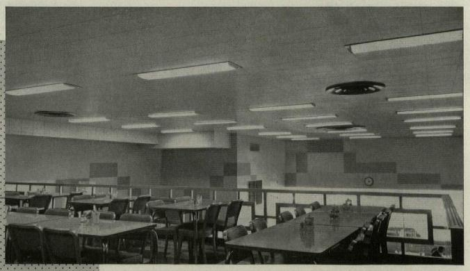
Diners are protected from noise and fire in this cafeteria by an Armstrong Arrestone ceiling. Arrestone is a metal pan unit backed up by a mineral wool pad. Both pan and pad are incombustible and have a noise-reduction coefficient of .85. Installed by mechanical suspension, Arrestone conceals pipes, ducts, and other utilities. . . . Forum Cafeteria, Wichita, Kansas
