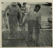
in the pattern; puts another platform alongside and proceeds along the surface. Wherever space is too tight to take the whole platform tool, he uses single and half blade tools. After the slab cures three days, the joints may be filled with mortar to play up the pattern. Surface hardness and porosity of *Ornamented Concrete* is the same as any standard concrete—and even better if the richer mix recommended by the tool supplier is used.
