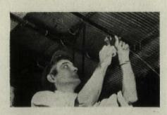
Flat, rigid Wheeling Metal Lath is easier to handle, goes up faster. Makes an ideal plaster base because of its definite keying action.
