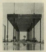
After floors are raised to half-mast, 40' columns are spliced with 27' extensions
