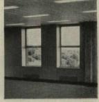
Milcor Type "B" standard wall unit, includes metal wainscot panels in addition to window stool, convector enclosure panels and head and jamb sections for the window openings.
