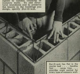
Butt-Weld . Trussed Design
