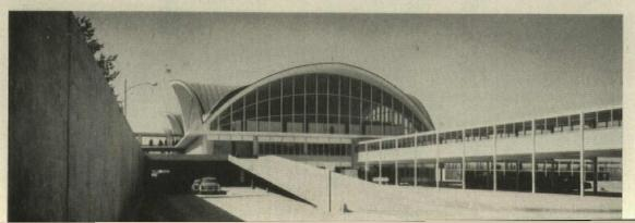
TRAFFIC SEPARATION for maximum efficiency is seen in section and photo (left). Passengers enter on canopied bridge, descend to middle level and out along finger to planes, while their baggage is trucked down the ramp and under the finger to join them. Trucks from the city deliver and pick up in separate tunnel (behind cars in photo). Below field level is pipe tunnel to separate utility building.
