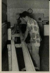
FIXTURES ARE PRE-ASSEMBLED AND PRE-WIRED AT FLOOR LEVEL
