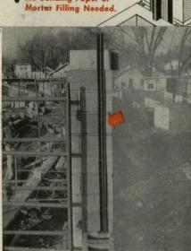
BLOK-JOINT'S "cross-shaped" rubber extrusion design simplifies construction of masonry wall control joints. Use BLOK-JOINT with any standard metal sash block!
