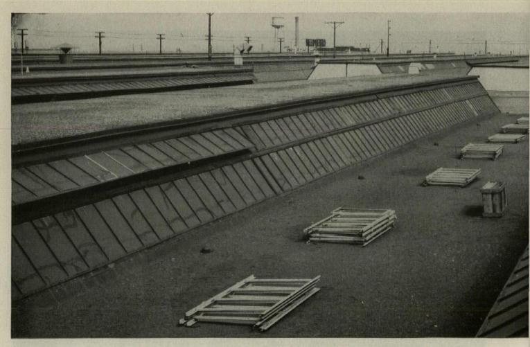
Fenestra Galvanized-Bonderized Industrial Steel Windows ready to replace the old monitor sash on Caterpillar Tractor Co. Building HH, Peoria, Illinois.
