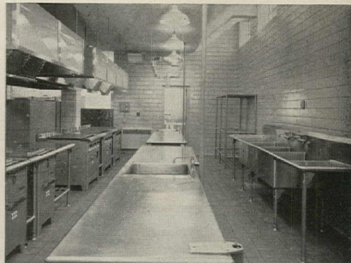
Range tops, sinks, storage racks, work surfaces, deep fat cookers, ventilating hoods and meat hangers are fabricated from ENDURO Stainless Steel. Equipment is mounted on legs which permit easy cleaning and allow air circulation. Well-defined, open aisles maintain smooth traffic flow.
