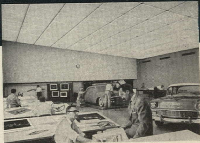
Styling Building, General Motors Technical Center, Detroit, Michigan. Modular lighting units have 5' x 5' pan type diffusers of PLEXIGLAS acrylic plastic. Architects: Eero Saarinen & Associates. Architects-Engineers: Smith, Hinchman & Grylls Inc.
