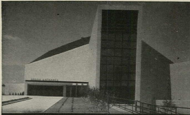
Arena entrance of the Omaha Civic Auditorium. Ceco-Meyer Steelform concrete floor joist construction and Ceco Open-Web Longspan Steel Joists were used in appropriate floor and roof areas of this building.
