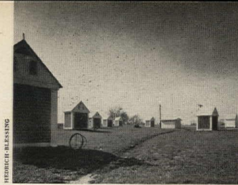
EIGHT HUTS shown here were built by Structural Clay Research to test different curtain walls, including metal, wood, brick, and tile. Shorter building, near center of picture, is control center, where heat flow measurements are recorded.
