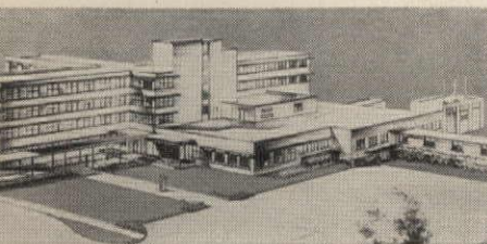
SelectTemp will heat the new wing of the Blanchard Valley Hospital, Findlay, Ohio, designed by Wilbur Watson Associates, Cleveland. In addition to room-by-room temperature control, SelecTemp's non-electric fans and thermostats insure safety in operating and other rooms.
