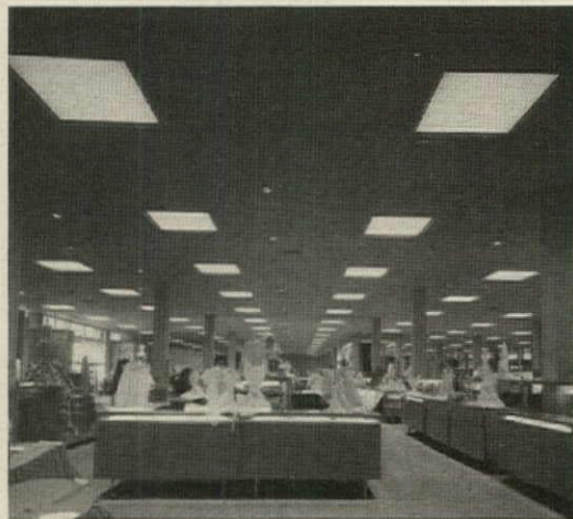
Above: Garcy No. RS7900 units installed in John Wanamaker's, Wynnewood, Pennsylvania
