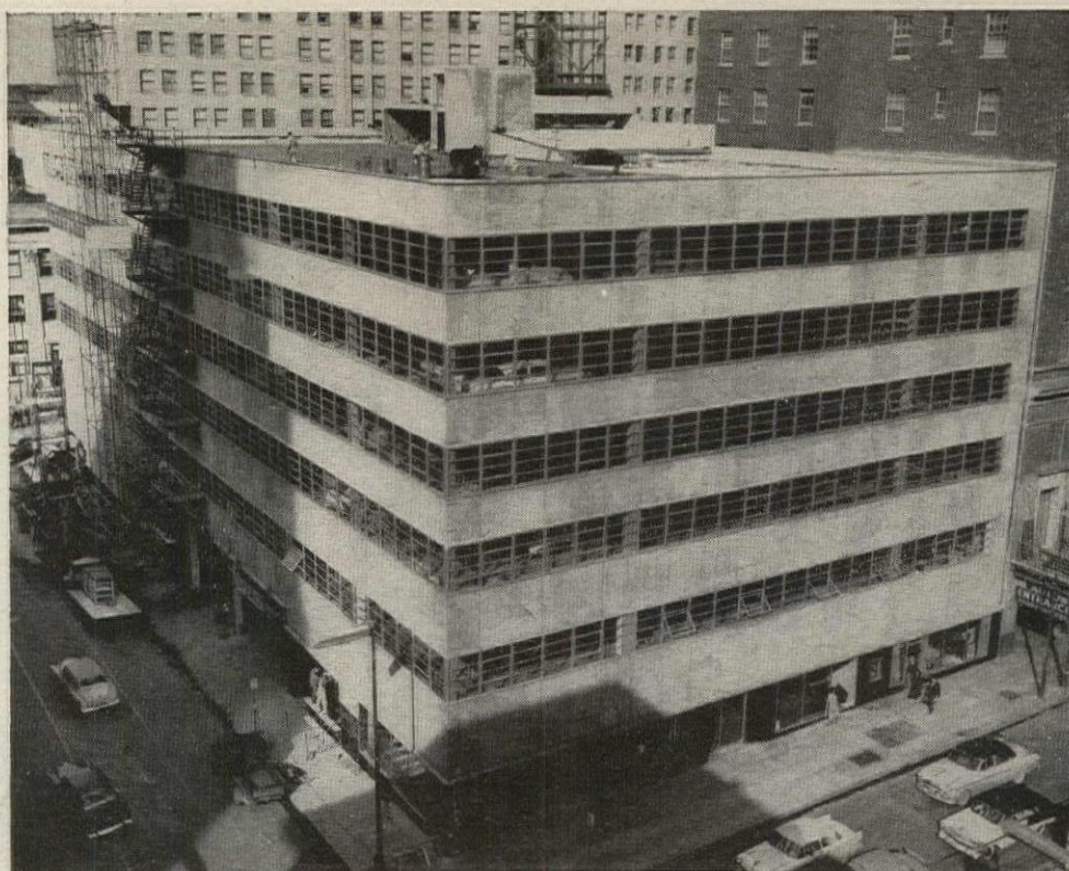
'Incor' Speeds Completion of 650-Car Garage
