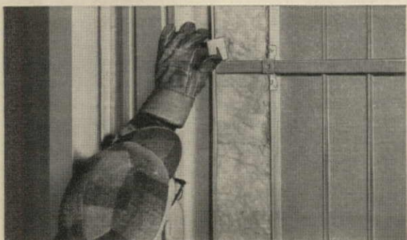
Exterior panel is clipped to 10-foot bar and crimped in place. Next panel overlaps and covers clip for an unbroken surface.
