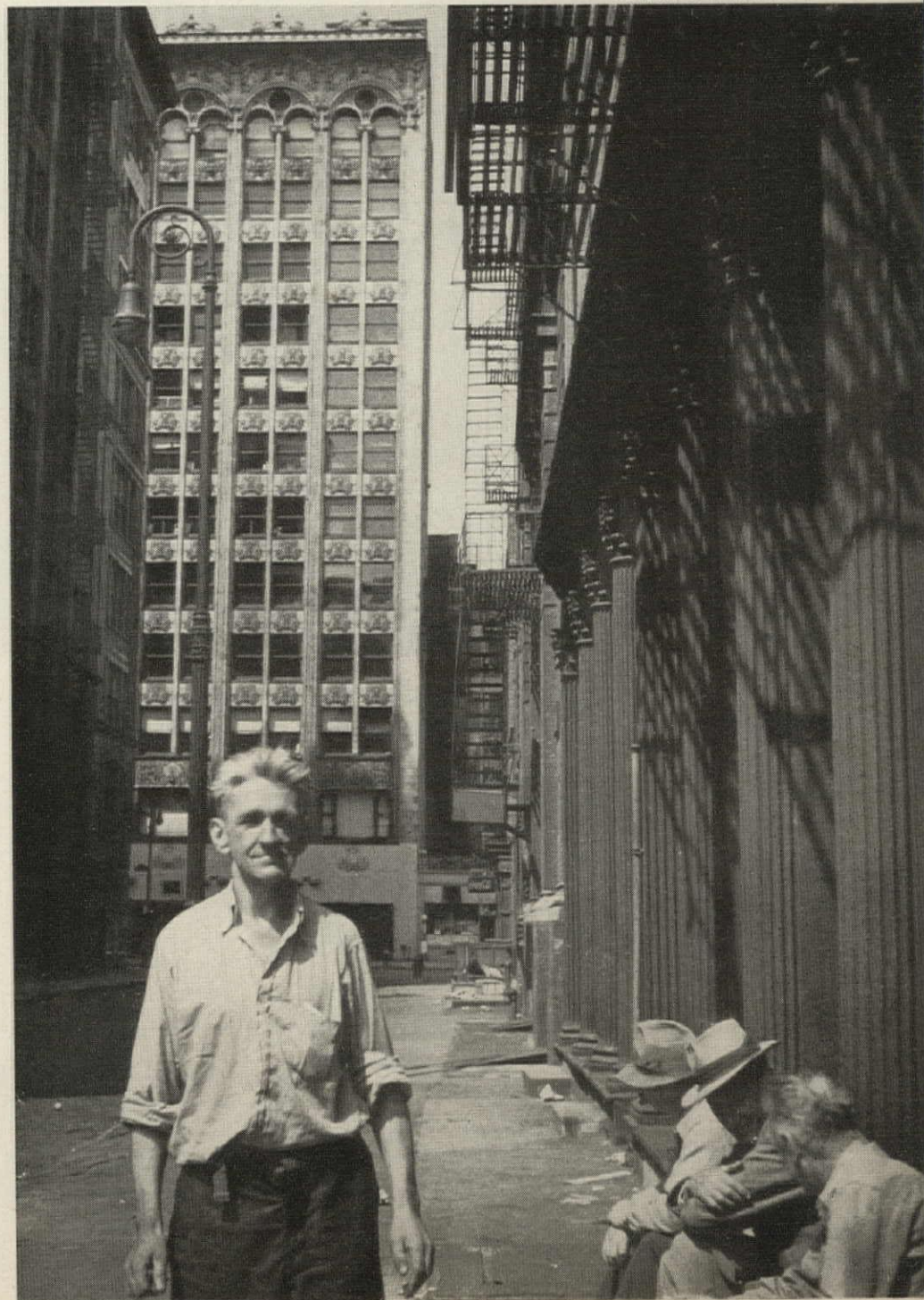
Condict Building, New York, 1897-98
