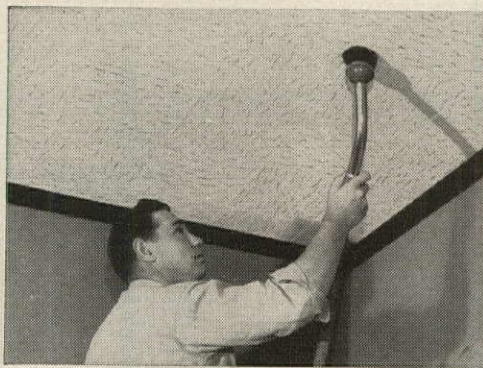
Vacuum cleaning with conventional attachments helps to keep Armstrong acoustical materials clean and new looking. A cloth slightly moistened with soapy water, or wallpaper cleaner, can also be used to remove most smudges.
