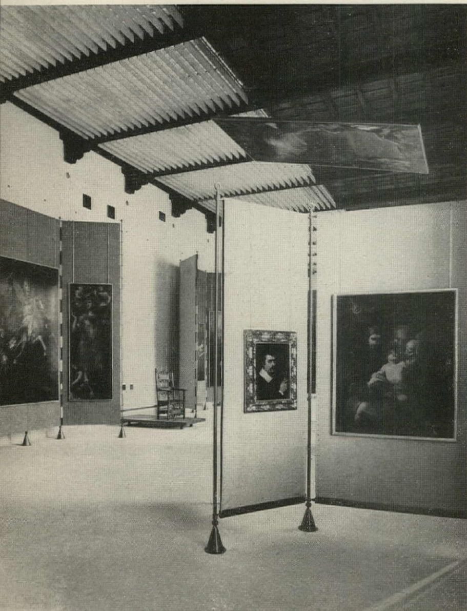
Lighting , as far as possible, is fitted into the building, not attached by a profusion of fixtures. A particularly recondite effort is made to use natural light, much in the technique of sophisticated photographic studios. The old ceiling, shown in photo (left) was opened to insert panels of adjustable vanes. Made of American larch, these can be tilted to compensate for angles of the sun.
