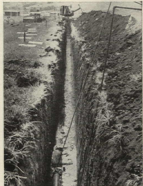
UNGRADED DITCH. Concrete pads were located at 10-foot intervals and 4" transite pipe supports placed on top of them.
