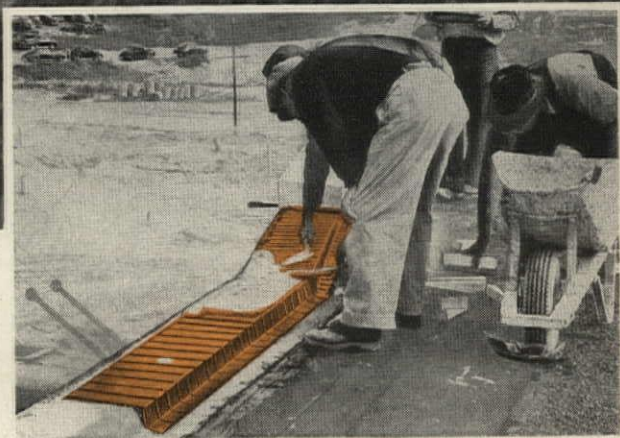
Typical Chase Thru-Wall Flashing installation.
