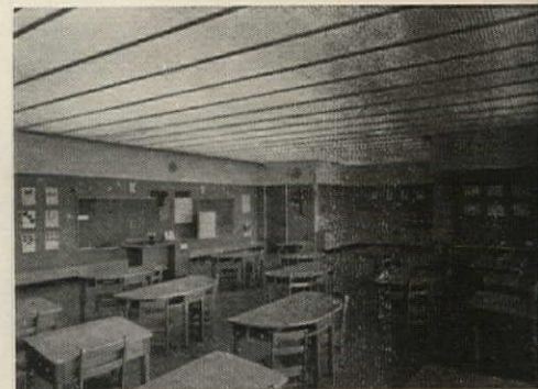
Luminous ceiling , among the first used in a school, given even light of 41 foot-candles at desk level (99 incl. daylight). Light from fluorescents is diffused through plastic.
