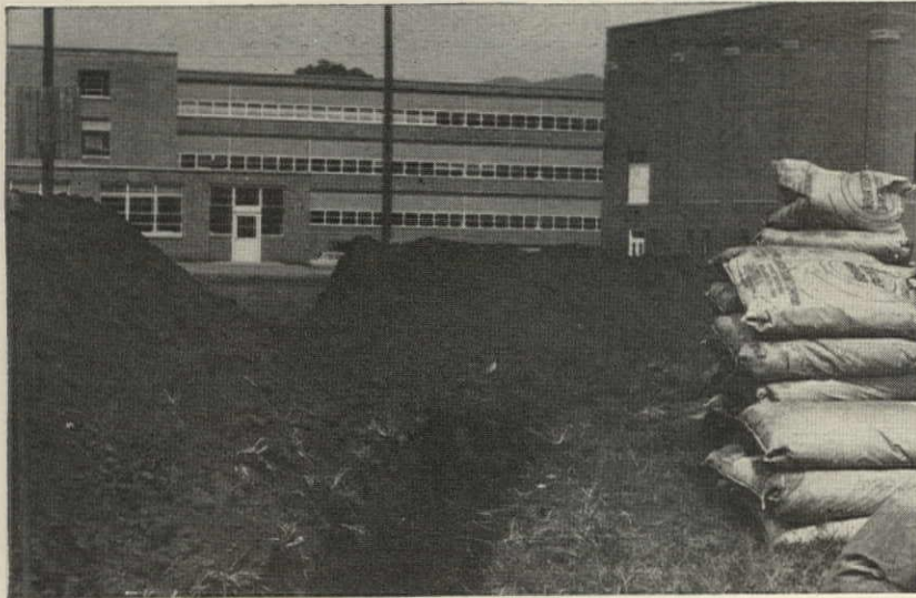
74 TONS of GILSULATE were poured around 1500-foot steam line.
