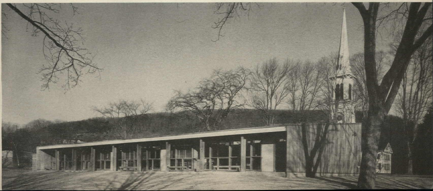
New school of simple horizontal lines sits modestly across road from old church. Photo (left) shows entrance at center, multipurpose wing at right, classroom clerestory at left above colored panels shielding toilets. At rear (below) classrooms open to south sun and playfield under 3' overhangs. Exposed columns support 33'-6" spans.
