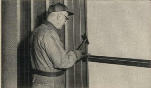
Back-up panel is clipped to horizontal girts of the building's framework. At the joints, the panels overlap and interlock.
