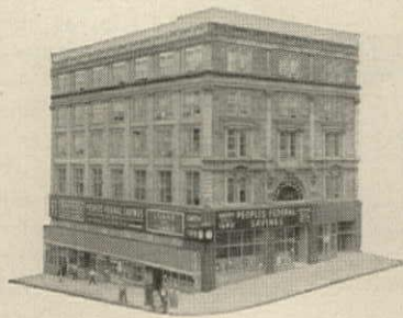
Modernization of Akron's oldest office building (Everett Building) included SelectTemp heating. Through an entire heating season the steam savings were 49.5%. This building uses district steam.
