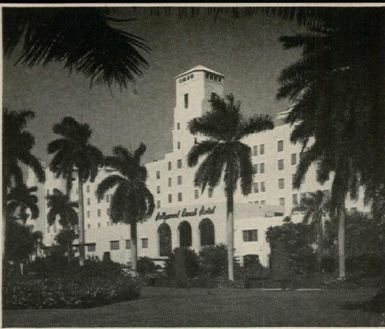
500-Room Hollywood Beach Hotel , Hollywood-by-the-Sea, Florida, was recently air conditioned, using a York TURBOMATIC system.
