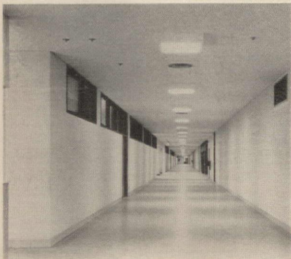
Typical corridor area lighted with Day-Brite fixtures. Note uniform illumination over entire corridor length.
