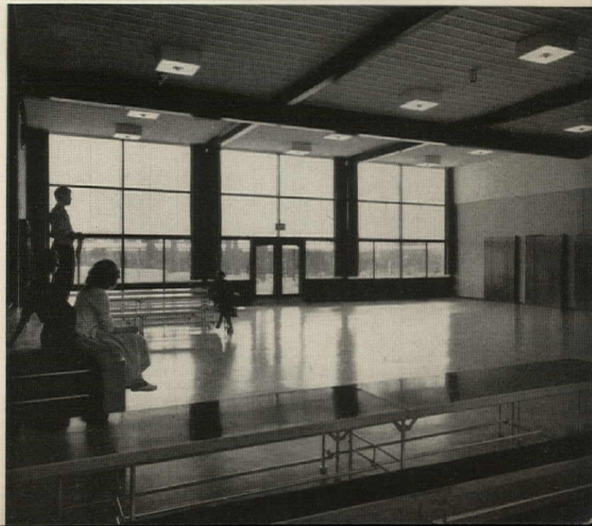
Meeting room has stage at left, folding lunch tables in walls. Translucent plastic shields upper two thirds of windows.
