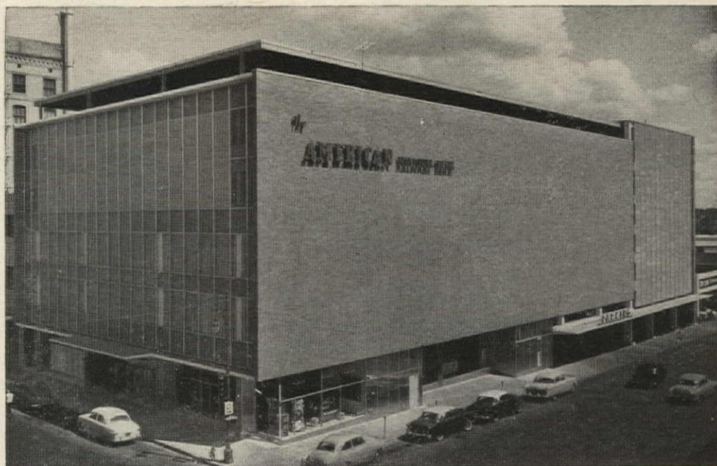
In Texas —American National Bank of Austin, Tex. Architect—Kuehne, Brooks and Barr, of Austin; Contractor—J. M. Odom of Austin.
