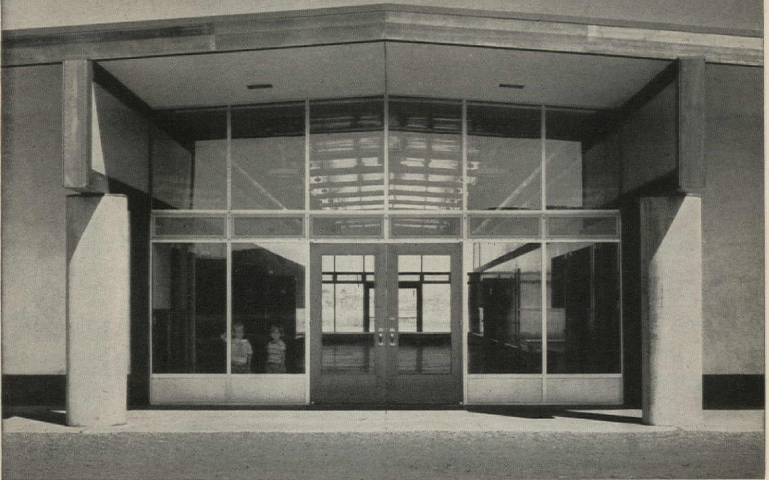
Broad hall , 20'-wide enclosed against wind and dust, is used for lunch, meetings. Hall is daylighted through end walls of glass in aluminum sash. What appears to be skylight is reflection on smooth ceiling.
