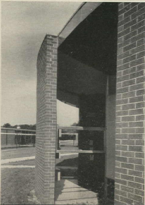
Library's "cogwheel" wall forms little light alcoves which would be greatly enhanced by planting in outdoor niches. Circular roof is cantilevered beyond indentation line. Shelving is backed by cement asbestos panel with glazing above and below.
