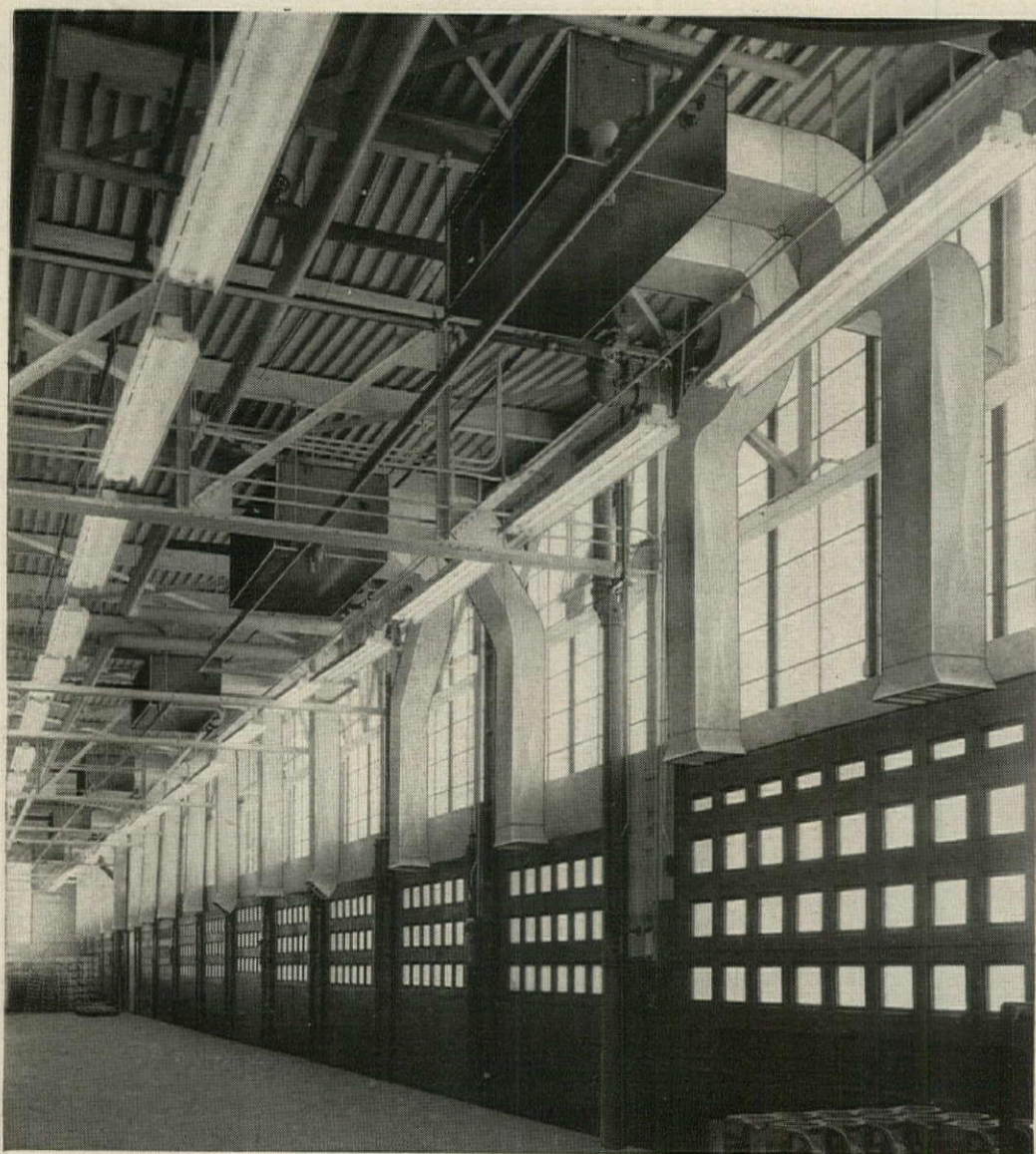
1. SIX HERMAN NELSON HEATING AND VENTILATING UNITS blanket the Chrysler Corporation's Transmission Plant shipping department doorways. Suspended from the ceiling, they hang out of the way . . . provide quiet operation. Available in heat capacities ranging to one million BTU's.
