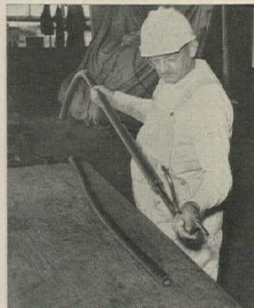
Slipped right over lines before they're put into operation, Armstrong Armaflex follows contours readily without time-consuming special cutting or fitting.
