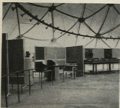
INTERIOR is huge, with 8,000 sq. ft. of unimpeded floor area. Weight per sq. ft. of enclosure is extremely low: 1.34 lb. Aluminum frame weighs 9,200 lb.; nylon skin, 1,300 lb.
