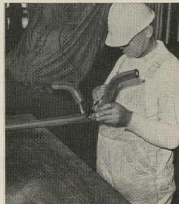
Joints are cemented with Armstrong 520 Adhesive. When they are required, fitting covers can be easily fabricated from miter-cut pieces of Armaflex.
