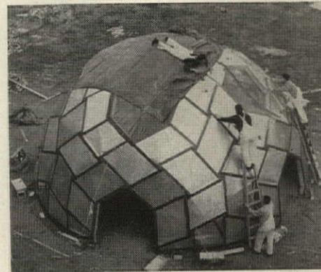
ALUMINUM IGLOO looked like this on Saturday morning. Students built it to serve no special purpose, only as exercise in creative thinking, using geodesic idea as a basic framework.
