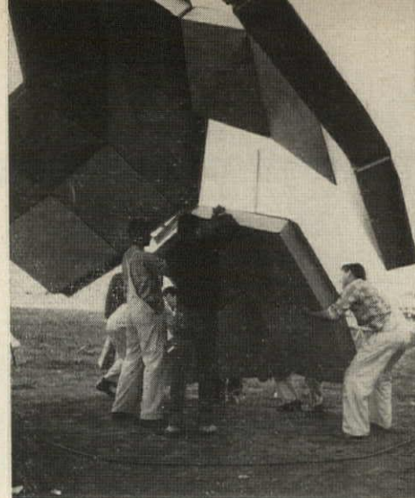
IN MONTREAL Fuller dome was designed and put together by architecture students at McGill University. Dome has aluminum skin, backed by paper-board boxes. Total weight: 1,000 lb. Left: detail of panel joint.
