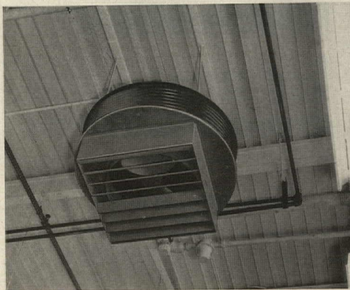
6. A HERMAN NELSON VERTICAL UNIT HEATER with louver diffuser discharges air vertically downward or at angle in various directions. Located in the main factory area, it is high on the ceiling, out of the way, yet directing warm air, without drafts, wherever it is needed.
