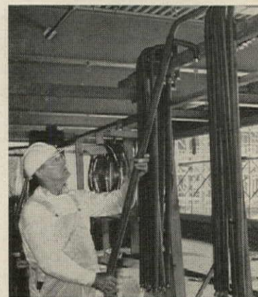
Pre-insulated with Armaflex, these heating-cooling lines are ready to be connected to the air-conditioning units. No further insulation is needed.
