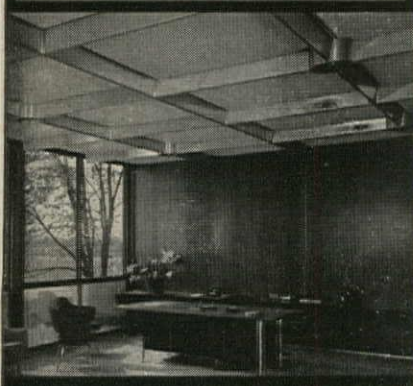
This executive office in the Research Administration Building, one of seven at the General Motors Technical Center air conditioned by Thermotank, shows a typical installation of Thermotank's custom-designed diffusers with integrated sprinkler heads
