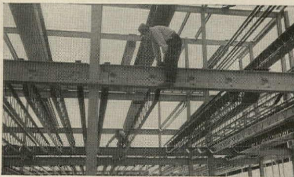
Floors in the Dutch Broadway High School, Elmhurst, N. Y., are made lightweight and fire-resistant with Truscon "O-T"® Open Truss Steel Joists. Here are strength and safety at low cost per square foot. Do you know about Truscon's new Clerespan® Steel Joist, 96 feet long? Send coupon for details.
