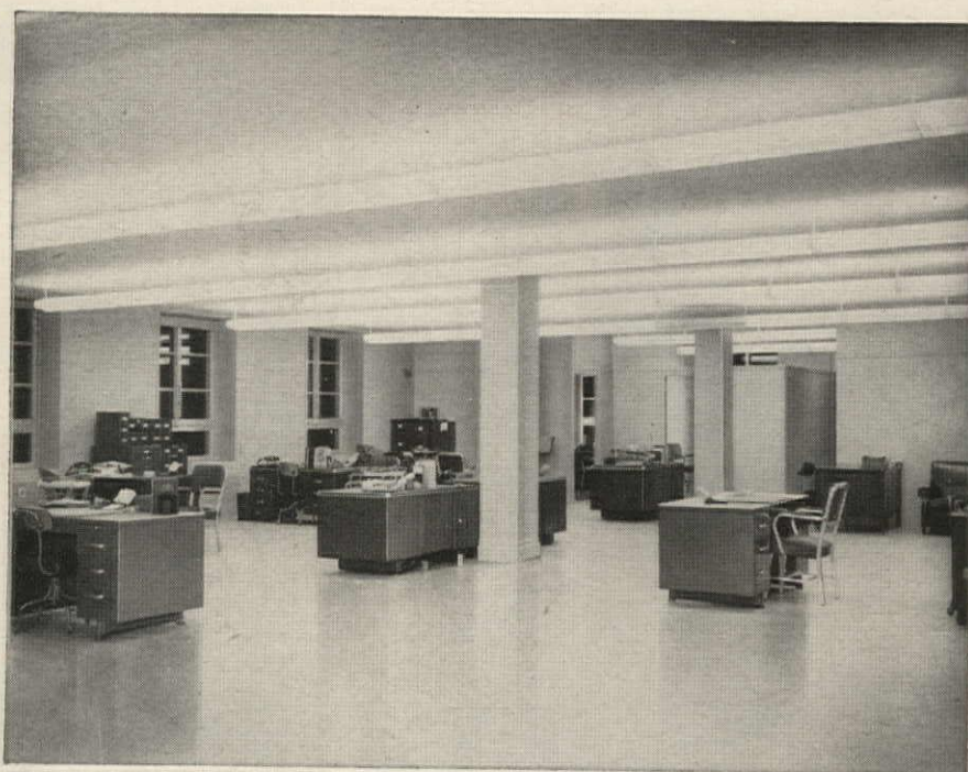
Here's an interior view showing a small part of the installation of Gold Seal Inlaid Linoleum. Actually, about 3½ acres of floor space are covered with this ¼" burlap-backed "Veltone."
