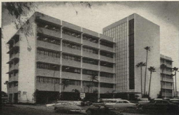
General Telephone Company, Santa Monica, California. This new 6-story office building uses Fenestra Electrifyfloor for "built-in" electrical availability and as a lateral diaphragm to resist earthquake and wind loads. Architects and Engineers — Albert C. Martin and Associates. General Contractor — George A. Fuller Company. Electrical Header Duct — National Electric Products Corporation.
