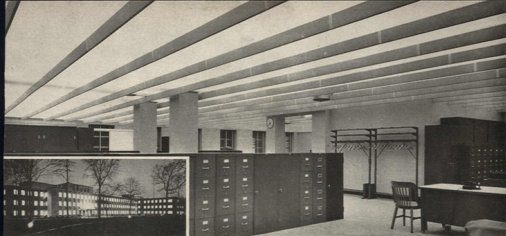
Cabin Hill, new central office of West Penn Power Company, Greensburg, Pa., has almost 90,000 square feet of illuminated ceilings. The ceiling components by Sylvania Electric Products Inc., Wheeling, W. Va
