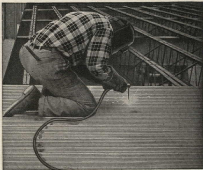
Ribform is easy to handle. Just weld it to the joists —the rigid sheets need no supplementary bracing.
