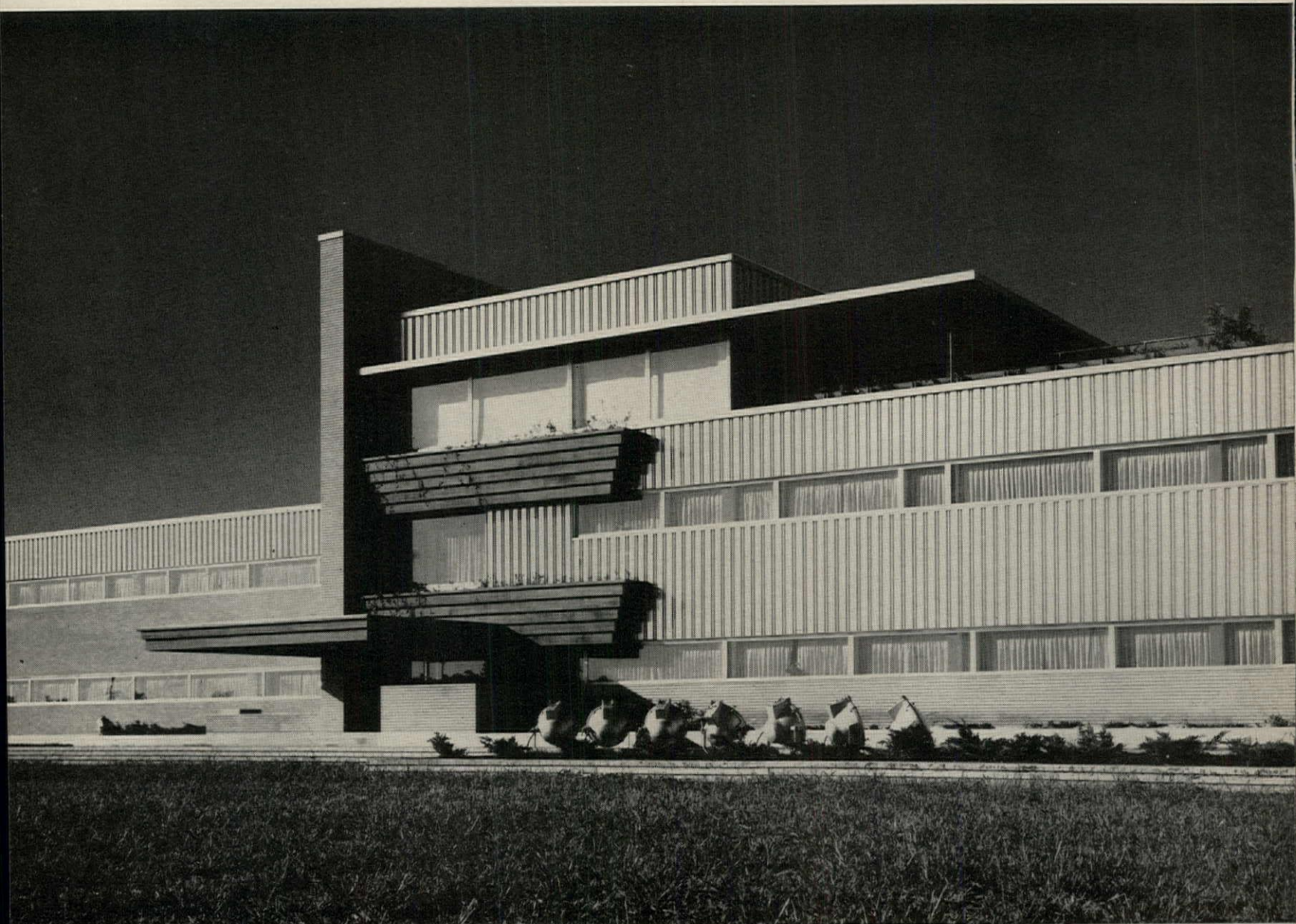
Office Building and Plant of the Schlumberger Well Survey Corporation, Houston, Texas. Over 20,000 sq. ft. of Mahon Insulated Metal Walls were employed in the design of this outstanding structure. Mackie & Kamrath, Architects. Tellepsen Construction Company, General Contractors.
