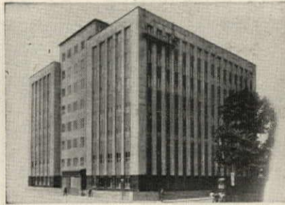
Continental Casualty Building, Toronto. Marani & Morris, architects. H. H. Angus and Associates, mechanical and electrical engineers. Canadian Comstock Co., Ltd., electrical contractor.
