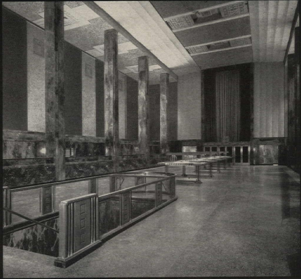
The First City National Bank of Houston, Texas, where wall and ceiling panels are sound conditioned with Sprayed "Limpet" Asbestos.
