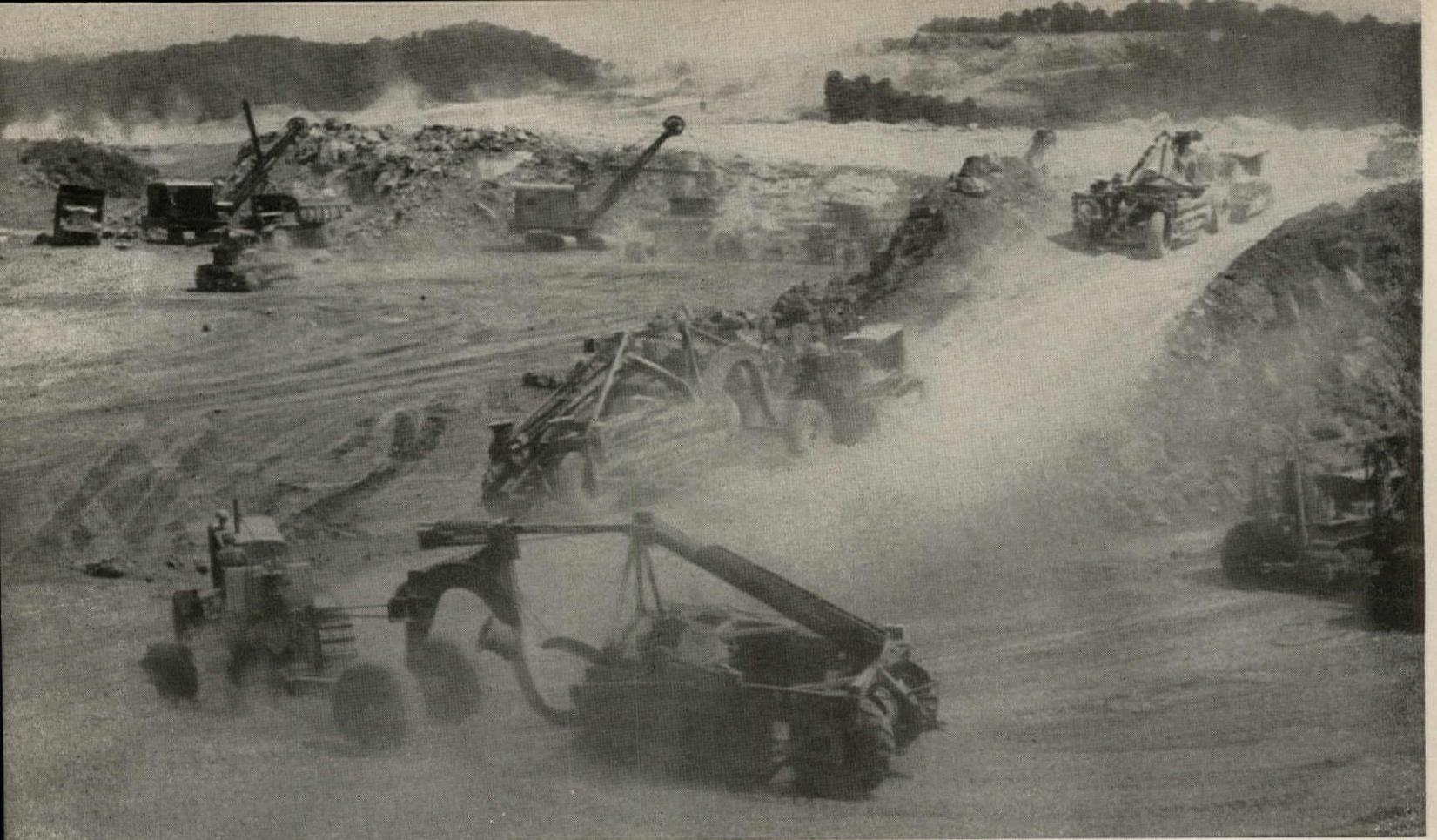
Scrapers, trucks and shovels race to quarry earth for a huge airport runway.
