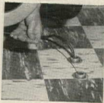
Next, install fitting in floor and fish wire.
