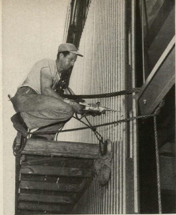
Industrial curtain wall of ribbed aluminum skins and glass-foam insulating core shows the essential simplicity and speed of assembly that such sandwich-wall panels bring to building.
