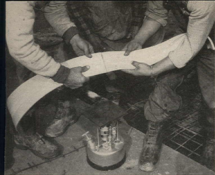
Splicing two sections of "Durajoint" waterstop is accomplished in the field by butt-welding ends after heating, without vulcanizing and with readily available equipment (soldering iron, hot plate and plumbers' torch). Operation is fast, clean, and efficient. It results in a strong, watertight bond.
