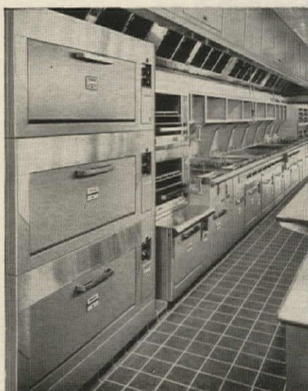
MAIN COOKING AREA • A 39' long section with 15 all-electric ovens, broilers, ranges and fryers. The entire area is covered by a stainless steel hood with built-in automatic CO 2 fire extinguishers that flood the hood when temperatures get too high.
