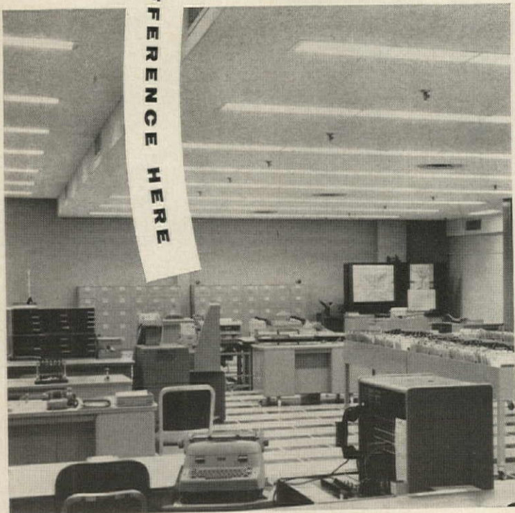
Office area lighted with Day-Brite recessed troffers.
