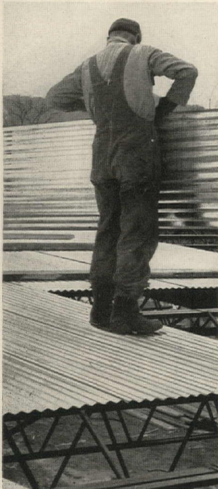
EASY TO HANDLE. Light Corruform sheets span up to 30", are quickly welded or clipped to steel joists, can be easily cut to fit openings.
