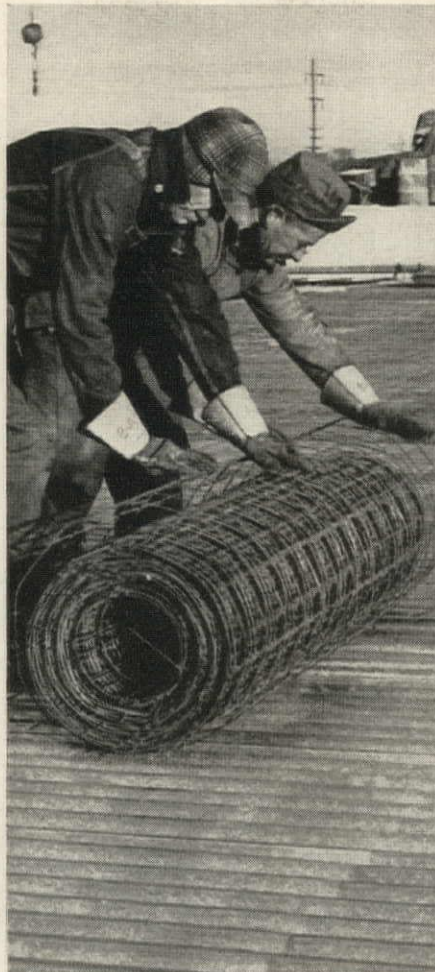
ROLL OUT MESH. Corruform in place offers an immediate, safe work platform, withstands normal construction abuse, adds stiffening to joists.
