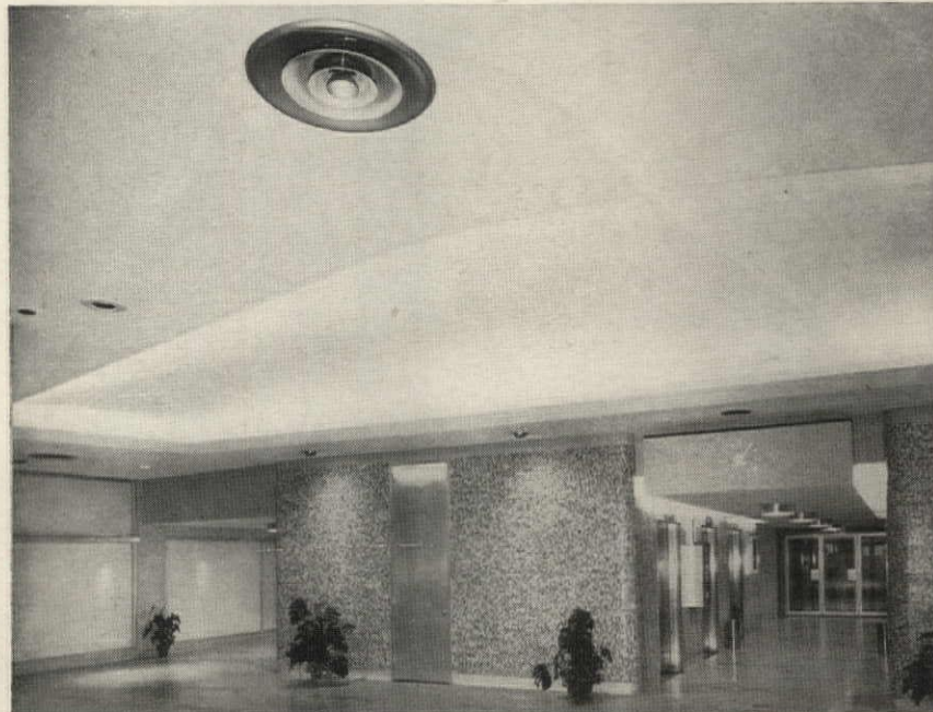
View of lobby showing Anemostat Air Diffusers
