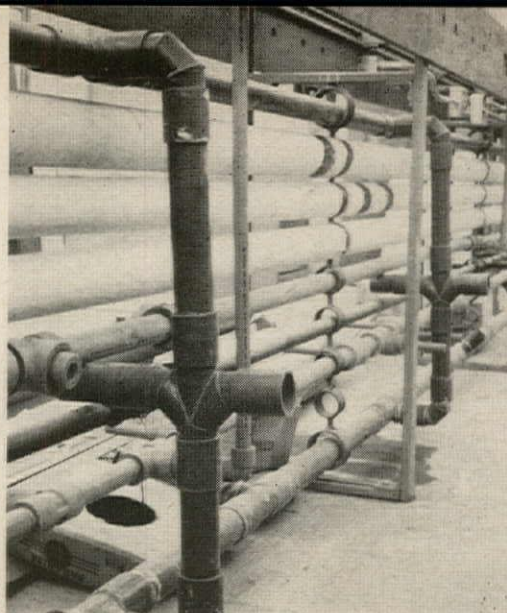
PLASTIC PIPE (polyvinyl chloride) is widely used (right) for all heating, ventilating, air-conditioning and laboratory services.
