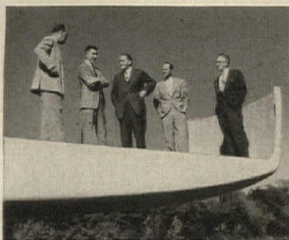
A molded "sandwich" section filled with rigid foam for added strength. Based on practical engineering principles for modular "bents" developed in the recent Monsanto-sponsored M.I.T. study, "Plastics in Housing."
