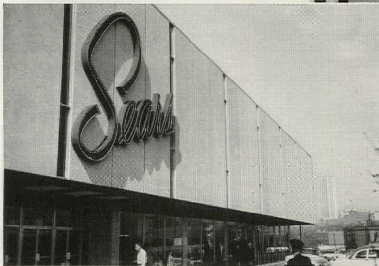
Modern architectural beauty is achieved with Marietta precast wall panel construction in a Nashville, Tenn. shopping outlet
