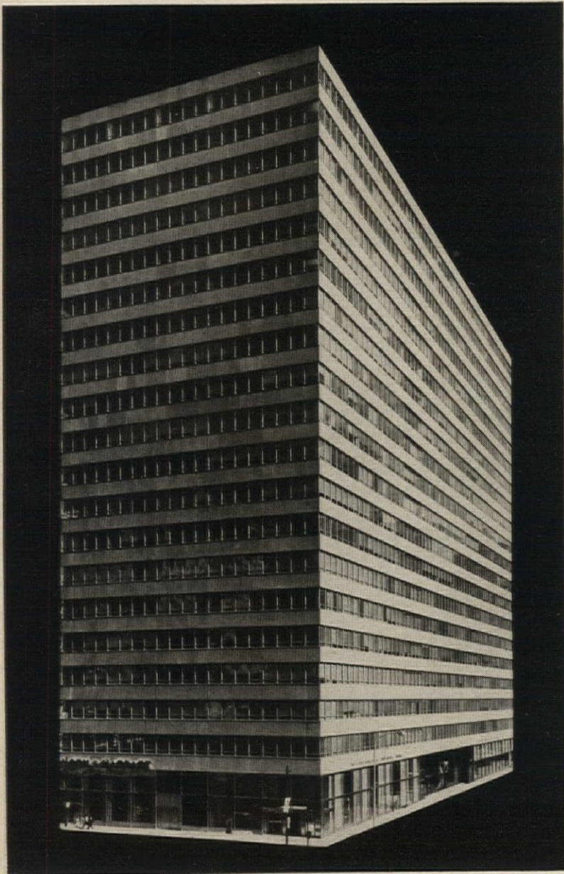
3 PENN CENTER, Philadelphia, Pa. Architects: Emery Roth & Sons. Contractors: Caldwell-Wingate Construction Co. Combination fixed and ventilator windows adapted from a standard Lupton design.
