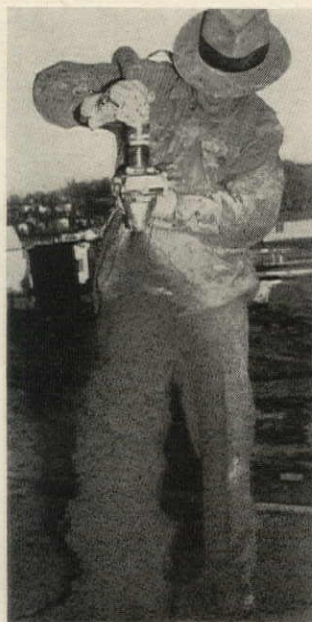
PREMIXED CONCRETE of controlled density and moisture content is gunned into place with pneumatic mortar equipment. Operator, armed with a long hose, places concrete for a dome or tall tower while the machinery stays on the ground. Operator in photo at right demonstrates low slump character of concrete.
