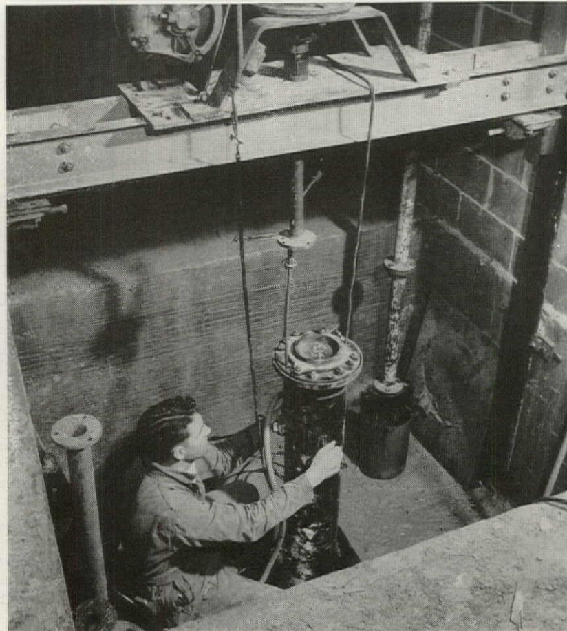
■ PLUNGER CASING is lowered into completed hole and anchored to steel pit beams resting on slab. All weight of the elevator will be supported here, eliminating the need for costly, heavy supporting sidewalls.
