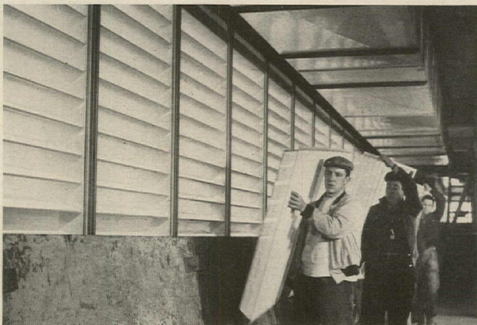
PLASTIC WINDOWS (acrylic) are lightweight, as seen above, cut out direct sunlight without the need for blinds or maintenance.
