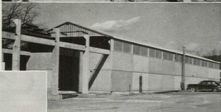
Marietta employs precast column, beam, girder and wall panel construction for fast erection of a precasting plant. Precast structural components are easily erected with a minimum of labor
