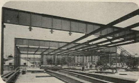
IN CONSTRUCTION —the immense exposed plate girders in place, with purlins being hung.
