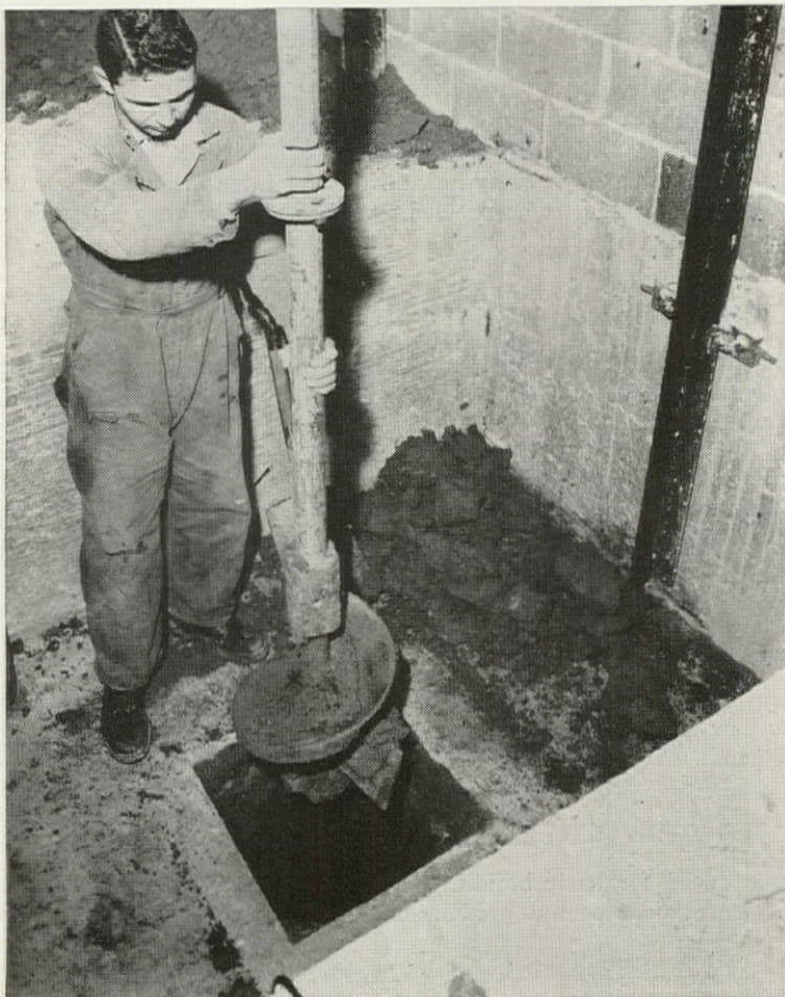
■ A POWERFUL hydraulic jack moves and supports the modern Rotary Oildraulic Elevator. This jack, raised by oil under pressure, will be installed in the hole being drilled in the elevator shaftway concrete slab floor.
