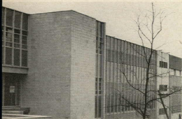
PLASTIC-FACED CONCRETE BLOCK (polyester) for external masonry (left) adds warm-toned waterproof quality to an old material.
