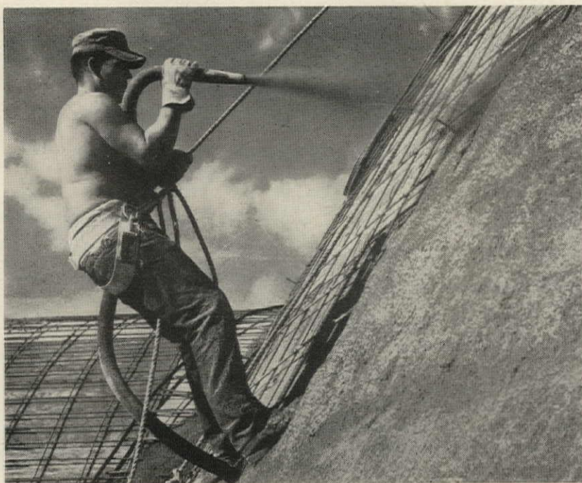
PREMIXED CONCRETE of controlled density and moisture content is gunned into place with pneumatic mortar equipment. Operator, armed with a long hose, places concrete for a dome or tall tower while the machinery stays on the ground. Operator in photo at right demonstrates low slump character of concrete.
