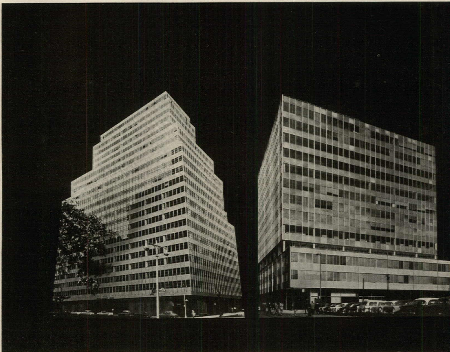
COLGATE-PALMOLIVE BUILDING, New York City. Architects: Emery Roth & Sons. Contractors: Uris Brothers. Lupton Aluminum Curtain Wall, Type "H", with 4'5" width module.
