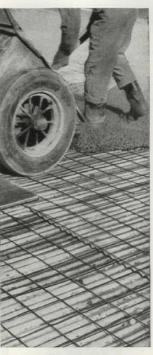
FAST CONCRETING. Rigid Corruform sheets permit slab to be cast and finished in one operation. The finished slab is ready for floor covering.
