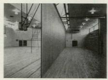
A single Cookson Partition, 104' long by 18' high, sections off an area 23' wide the full length of the gymnasium. A second Cookson Partition, 23' long by 18' high, is closed at right angles to provide two smaller rooms. The latter partition has a 3' by 7' opening. Both are operated by concealed, remote controlled electric operators.
