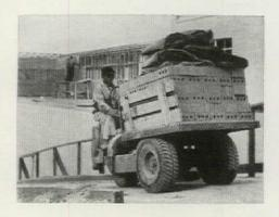
Scott Cretes and a ramp (above) in lieu of an elevator or scaffold and hoist in the construction of a three-story plant in Kearny, N. J. The 14 cu. ft. truck pictured has interchangeable platforms for carrying different loads. It costs about \$1,200—or \$1 a lb.
