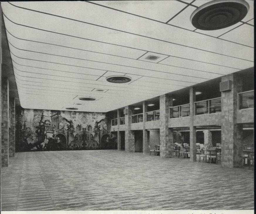
2,300 square feet of light in a ballroom of New York's Park Sheraton Hotel can be varied in intensity to suit the activity. End sections are curved to enclose the fixtures near the balcony. The panels resist warping, cracking and discoloration—are normally unaffected by moisture and oil. Another UL listed installation. Ceiling components in this installation by Luminous Ceilings Inc., Chicago, Ill.
