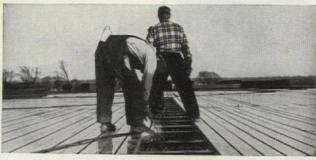
Truscon Ferrobord® Steeldeck, welded or clipped to the top of Clerespan Joists, produces an ideal, fire-resistant roof. Ferrobord is light, easy to handle, easy to place. Long lengths span three or more purlins. It roofs large areas quickly—flat or pitched. Full-length interlocking increases strength. When laid, Ferrobord provides the perfect surface for application of insulation and built-up waterproofing. Send coupon for specifications and tables.
