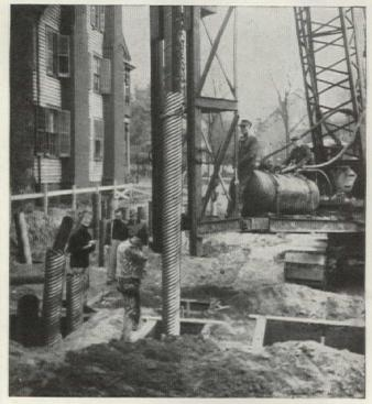
Armco Pile Shells are driven with a mandrel. Required penetration on the Augusta building was four blows per inch.
