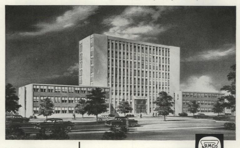
Drawing of the new Augusta-Richmond County Municipal Building in Augusta, Georgia. Building rests on 691 piles consisting of concrete-filled Armco Hel-Cor Pile Shells.
