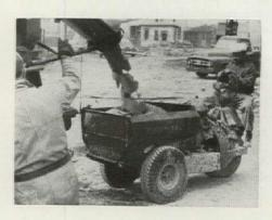
needed. Driven and unloaded by one man, the T 52 model has forward and reverse speeds up to 15 mph and can climb inclines as steep as 25%. Drive wheels are situated directly under the load for power, and heavy duty tires are reported to grip any indoor or outdoor surface. A locking brake lever holds the buggy immobile when necessary. For fast and convenient materials handling, Builder Carl Buhr used three
