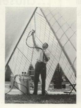
lieves the technique may eventually yield better and less-expensive houses. To a tubular steel frame (picture) is added a gridwork of cloth tape, spaced at 6" intervals. The fibers of the sprayon vinyl form a base-coat web across the grid. A second spray coat, with white pigment added to protect the plastic from deterioration by sunlight. shrinks to a rubbery hardness, giving the structure a prestressed skin.
