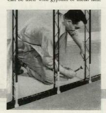
GOLD BOND GYPSUM LATH, locked with Gold Bond Clips, gives a strong plaster base. Holostud, with gypsum lath, gives sound transmission loss rating up to 50 decibels.
