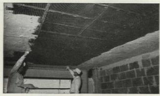
Suspend a fire-resistant ceiling from Clerespan Joists by using Truscon Metal Lath, channels and plaster. When plastered, it forms a lightweight fire-resistive "membrane", wall to wall, protecting structural members from any fire below them. Truscon offers more than 40 different Metal Lath items and accessories that are accepted by all building codes. Your plastering contractor knows them.
