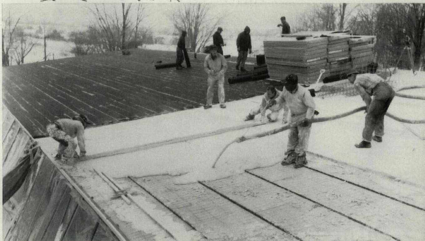
FIREFIGHTER GYPSUM DECKS can be poured in the coldest weather during which mechanics normally work. This job: 15° above zero.
