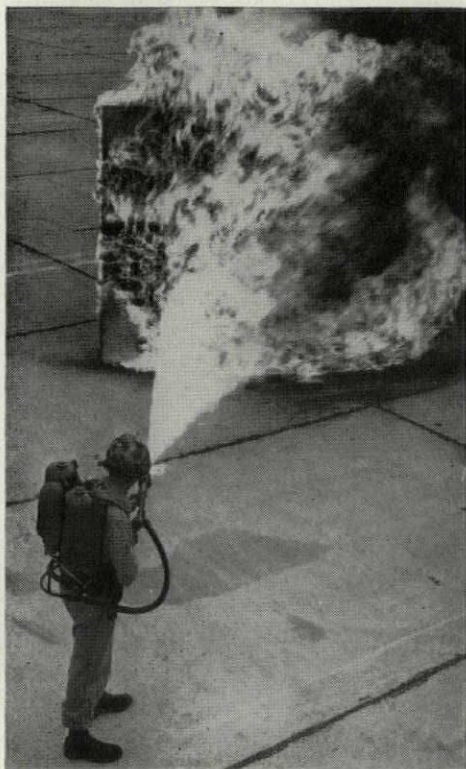
After Marine's flame-thrower blast . . . the panel stands—smudged but in good shape.
