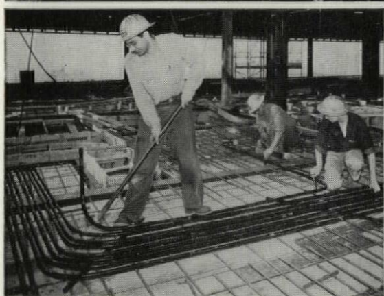
Installing steel conduit on the 18th floor of the first Penn Center Plaza Building.
