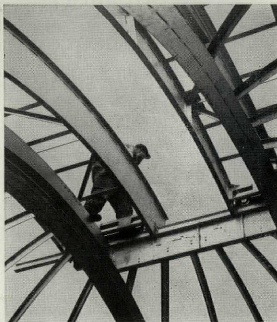
The dome being erected at the observatory.
