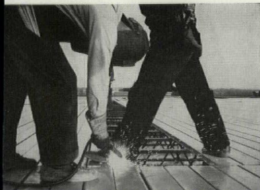
Truscon Ferrobord® Steeldeck is welded to the top of Clerspan joists to produce a fire-resistant roof. Ferrobord is light, easy to handle, easy to place. Long lengths span three or more purlins. It roofs large areas quickly. Top surface is ideal for the application of insulation, and built-up waterproofing.
