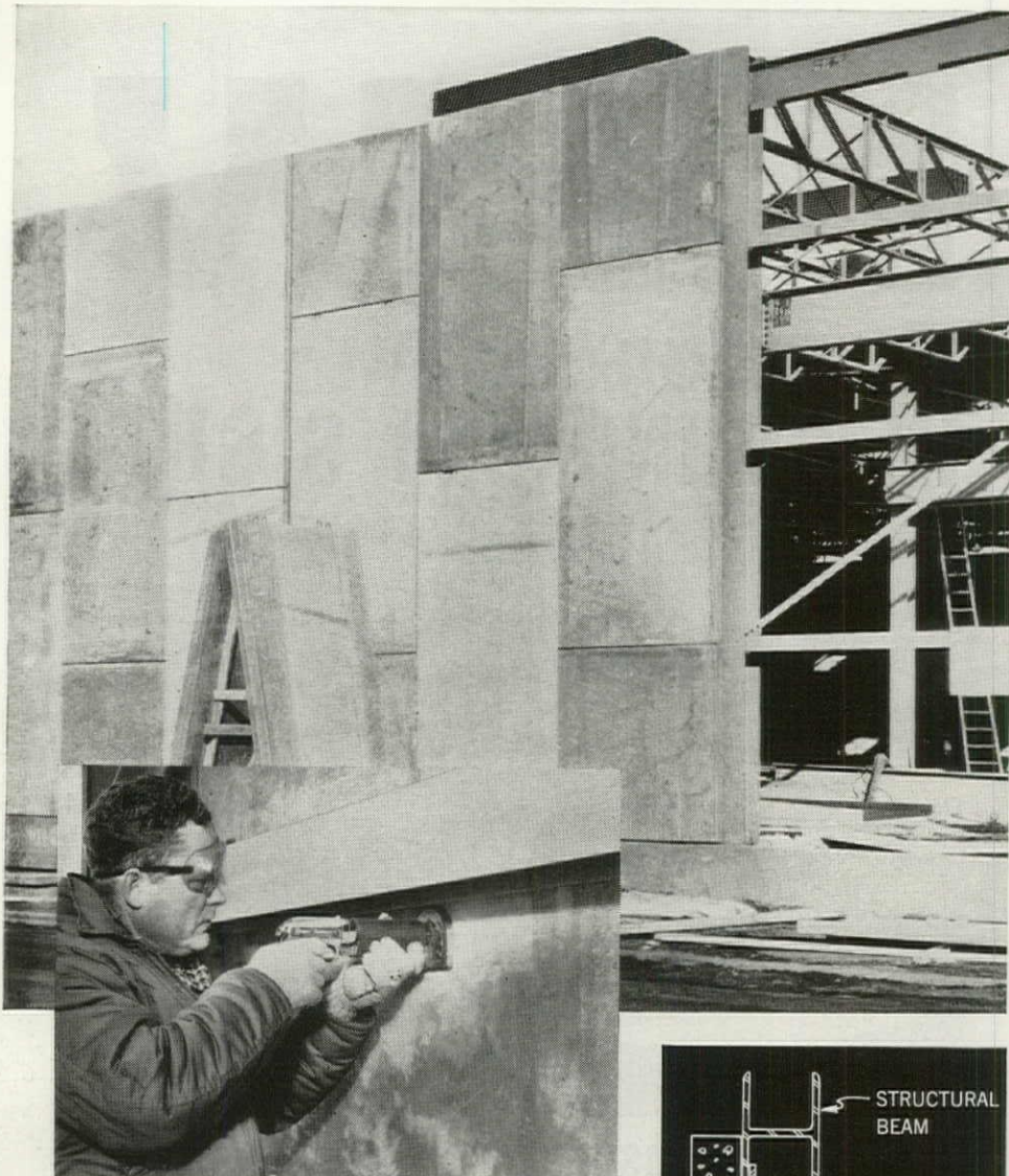
Two 3-inch RAMSET threaded fasteners hold each of these pre-cast concrete curtain-wall slabs . . . some weighing as much as 2 tons!
