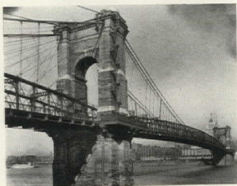
THE SUSPENSION BRIDGE, represented by the historic Cincinnati structure above, the first large suspension bridge in the US, designed and built by the great John A. Roebling shortly after the Civil War, provided the principle of steel-in-tension for the historic modern building (left), the first big suspension-roof structure of its kind in the US. This shows the raising in 1952 of the great cable roof of Raleigh Arena for North Carolina State College, conceived by the late Matthew Nowicki, built by Engineer Fred Severud.
