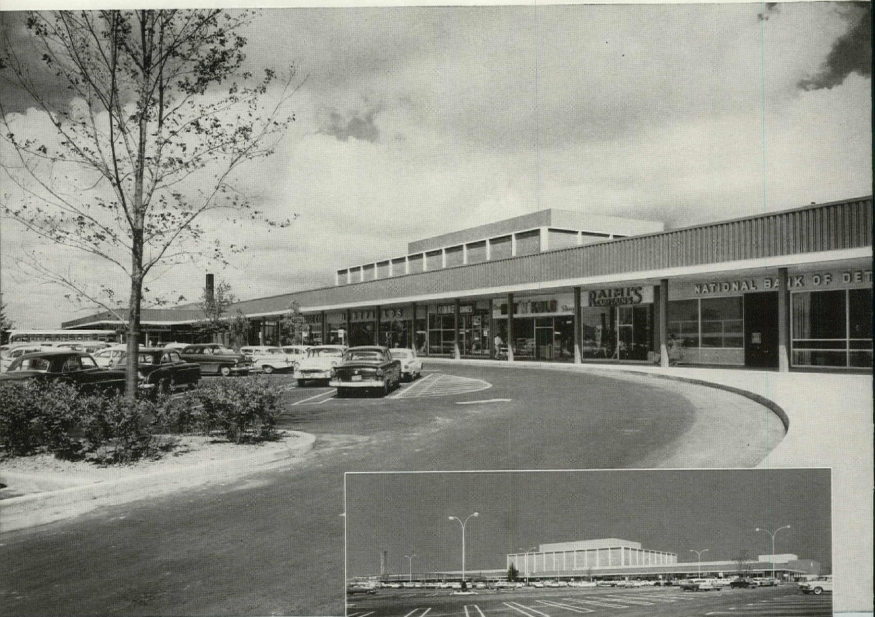
Eastland Shopping Center in the northeast section of Detroit, Michigan. 56,000 Sq. Ft. of Mahon Insulated Metal Curtain Walls and 48,000 Sq. Ft. of Mahon Steel Roof Deck were employed in the construction of this outstanding and colorful structure. Victor Gruen & Associates, Architects. O. W. Burke Co., Gen. Contrs.
