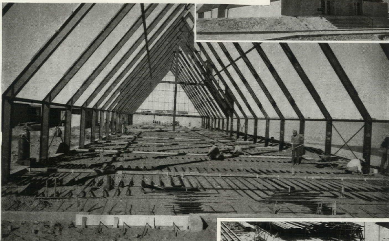
Steel Pipe Radiant Panels in main auditorium, 1" standard black pipe on 12" centers.
