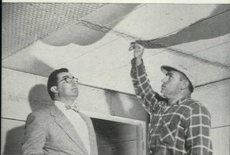
Eby (left) inspects application of Keycorner, used to reinforce joints. Keycorner is also used at all wall and corner junctures.
