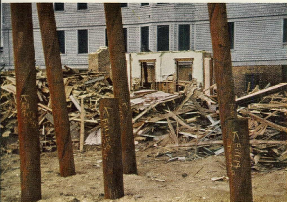
The bars and shops of Bridgeport's West Side were blanched by unexpected sunlight when the wreckers swept past. After destruction came pipe pilings, sunk through mud to bedrock.
