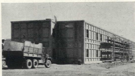
BARRACKS of Schokbeton, or densified concrete, show neatness of this thin, hung masonry-panel construction. Below is cross-section detail of wall showing interior insulating panel.
