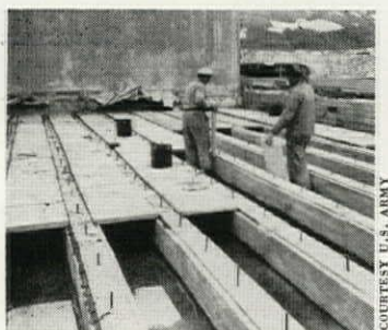
VENTILATION DUCTS of pre-cast concrete and other materials are formed in foundations of heavy utility buildings.
