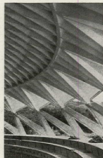
Triangular sections web out from 36 support points to tie the diamond-shaped sections to the wide-spaced piers.
