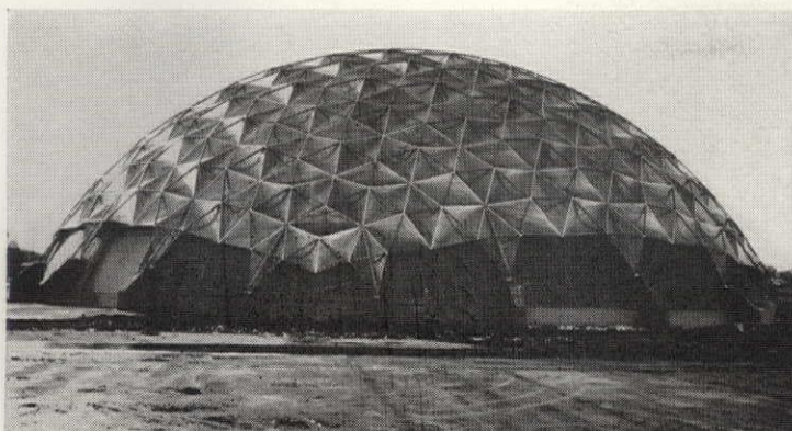
COMPLETED DOMES , a factory in Kansas (left) and an auditorium in Hawaii illustrate the dome's range of applications. Hawaiian dome points up the architect's importance: Welton Becket, who designed entrances, periphery, and interior at Hawaii, had to develop a wall system and cope with noise control and mechanical problems. Dome is not completely predesigned.
