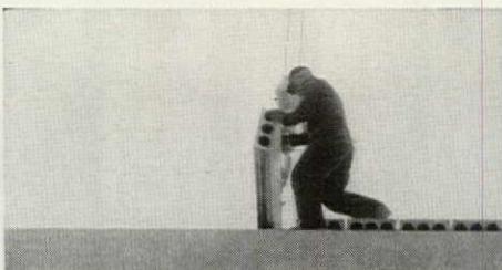
Left: Erection of precast bent. Center: Flexicore slabs used for second floor and roof. Right: Flexicore exposed for guest room ceiling.
