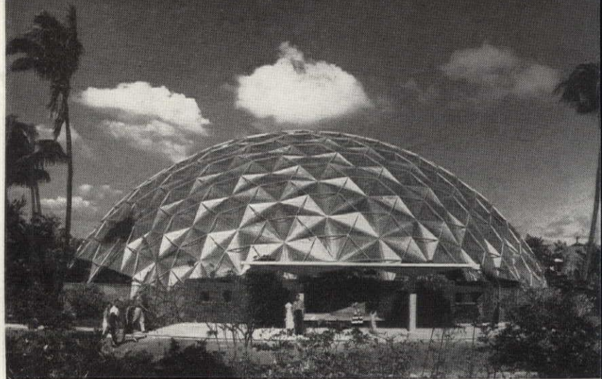
COMPLETED DOMES , a factory in Kansas (left) and an auditorium in Hawaii illustrate the dome's range of applications. Hawaiian dome points up the architect's importance: Welton Becket, who designed entrances, periphery, and interior at Hawaii, had to develop a wall system and cope with noise control and mechanical problems. Dome is not completely predesigned.
