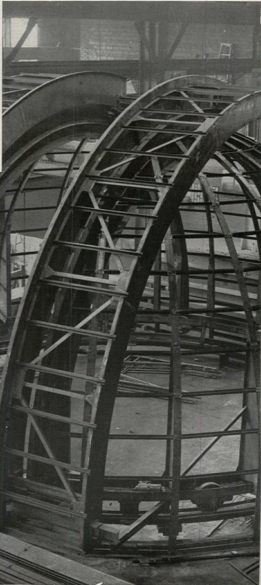
The Nassau Astronomical Station. The viewing opening is comprised of two shutters, which slide to the right and left. Fully open, the port is 7\frac{1}{2} feet wide. A 1 h.p. motor opens and closes the shutters.
