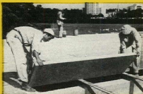
INSULROCK roof slabs are easily and directly applied to roof spans
