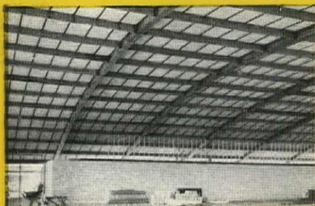
INSULROCK furnishes 196-ft. acoustical ceiling in new Selma, Alabama, armory
