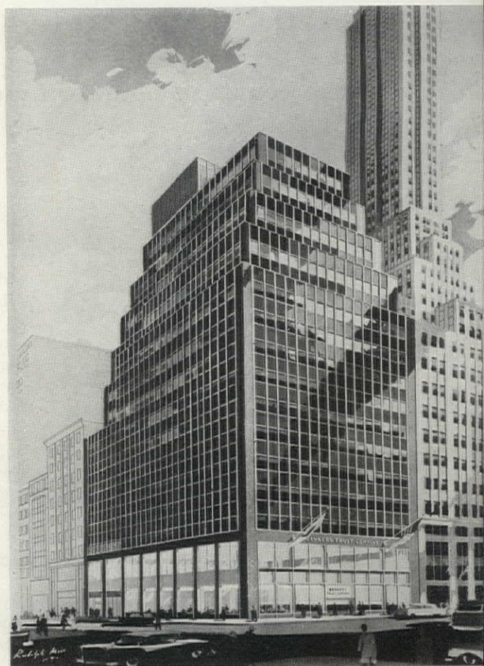
NEW BANKERS TRUST (right), sheathed in glass and aluminum, will be 19 stories high, with new section at rear. Added floors above old building, whose original frame could support only 17 stories, are made possible by unusual structural scheme (left). A big bridge truss (heavy lines) will be cantilevered out over the old building from new wing, and part of the weight of the top floors will be hung from this truss.
