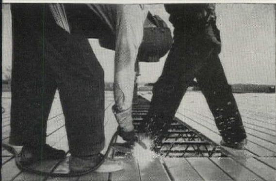
Truscon Ferroboard® Steeldeck is welded to the top of Clerespan joists to produce a fire-resistant roof. Ferroboard is light, easy to handle, easy to place. Long lengths span three or more purlins. It roofs large areas quickly. Top surface is ideal for the application of insulation, and built-up waterproofing.
