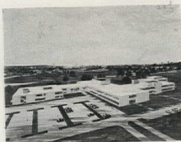
Suffolk County Courthouse, Riverhead, N. Y.—an example of curtain wall construction using Slidewall's new modular panel system made with Bridgeport Aluminum.
