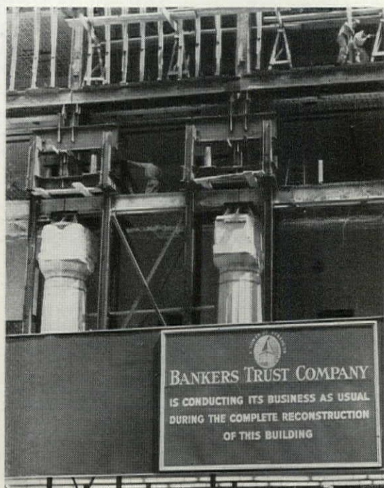
OLD BANKERS TRUST BUILDING (left) was stripped down to its 12-story steel frame (right). Big, 30-ton marble pillars (above), supporting part of the old steel frame in the Victorian anomaly, were removed by jacking up the frame above them, replacing them with new steel columns.
