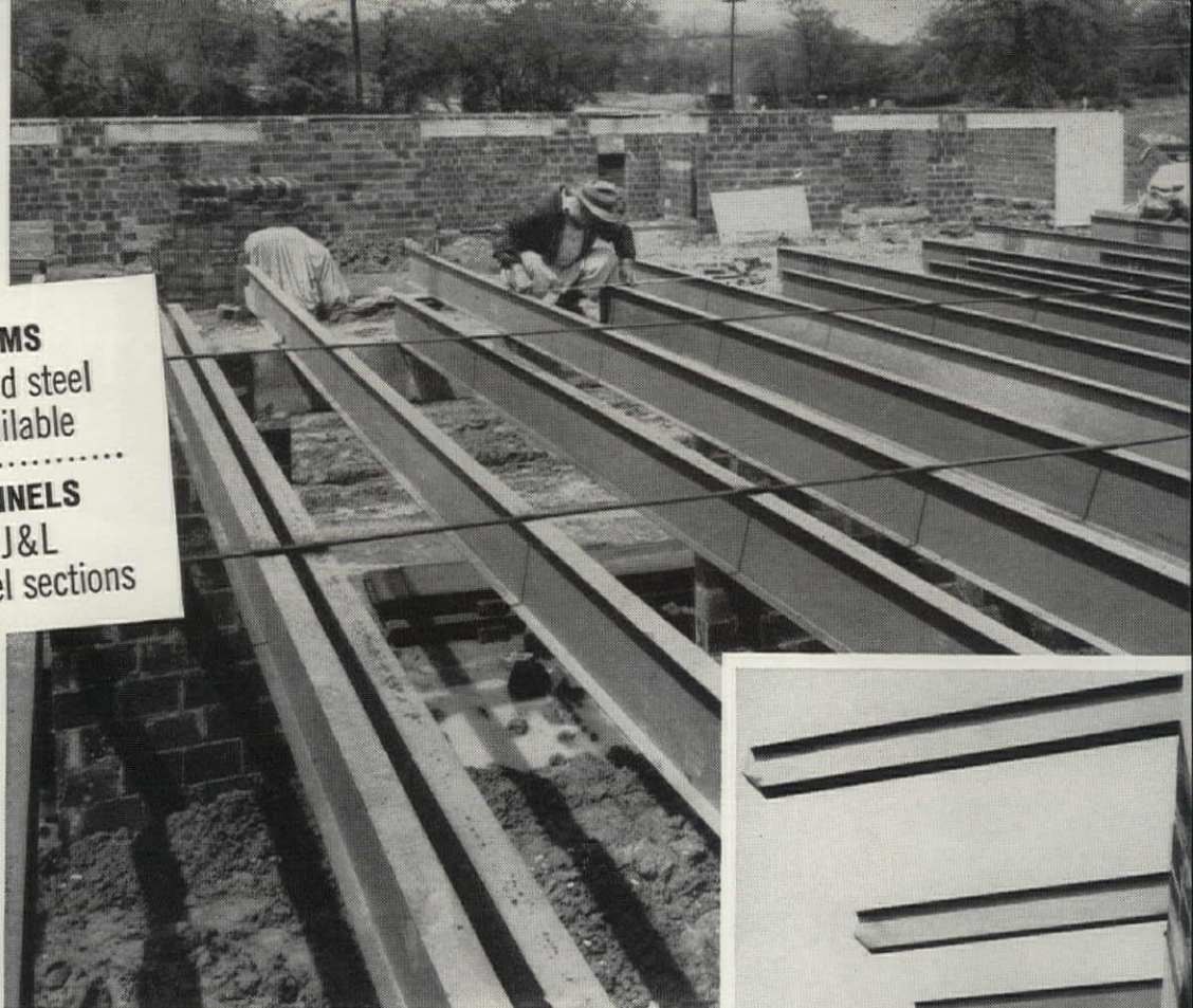
10" (9#) Junior Beams are used in this two-story motel as second floor joists and as roof purlins. Second floor system and balcony will support a 40 pound per square foot live load.
