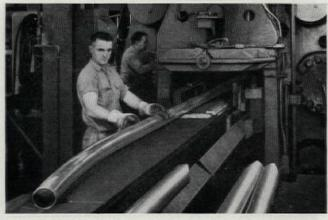
Aluminum tubing for the ASM "space lattice" emerges from extrusion press at Kaiser Aluminum's Halethorpe, Maryland plant. About 5¼ miles of tubing were supplied (4 and 6-inch diameters) ...plus aluminum sheet, castings, forgings and 7¼ miles of extruded tension rod. Total: about 200,000 pounds of aluminum!
