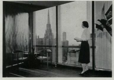
The curtain wall has floor-to-ceiling units of TWINDOW-Pittsburgh's twin-pane insulating window-glazed with SOLEX to keep interiors comfortable. Each reception area has its own handsome entrance with departmental listings mounted in the center of suspended HERCULITE panels.
