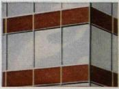
Vitrolux is heat-strengthened polished plate glass for spandrels. Ceramic color is fire-fused to the back surface. It won't fade or deteriorate – ever. Your choice of 16 standard colors, black, white, or matched to your color sample.
