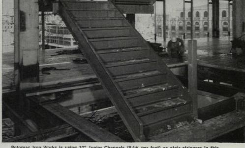
Potomac Iron Works is using 10" Junior Channels (8.4% per foot) as stair stringers in this 15-story Baltimore, Maryland, state office building with 12-gauge J&L hot rolled sheet steel as risers. General contractor: Blake Construction Company, Washington, D. C. Architects: Fisher, Nes, Campbell & Associates, Baltimore.
