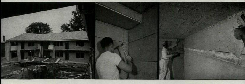
A typical quality Olson Lathing job goes into this 17-flat apartment building in Chicago. Many builders are switching back to lath and plaster because of the increased fire resistance, lower maintenance and permanent beauty that plaster walls provide.
