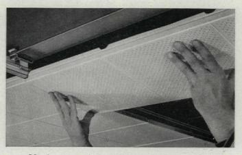
Metal pan acoustical panels snap into place. No studwelding, no attachment pins necessary.
