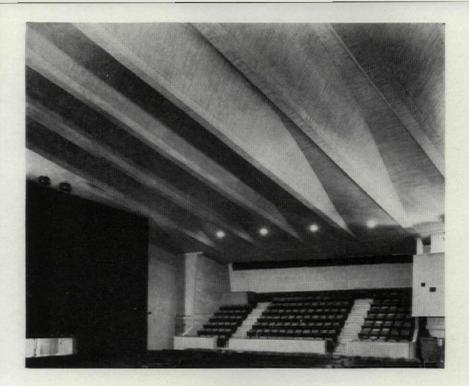
**Ceiling** of Plenary Session Hall shows the triangular corrugations of the roof and the undulating slab that intersects this triangular space-frame. The concrete ceilings and the columns in the Delegates' Lounge were left in natural finish. Press, radio, TV, newsreel and simultaneous translation facilities are recessed in the paneled side walls of the Hall.
