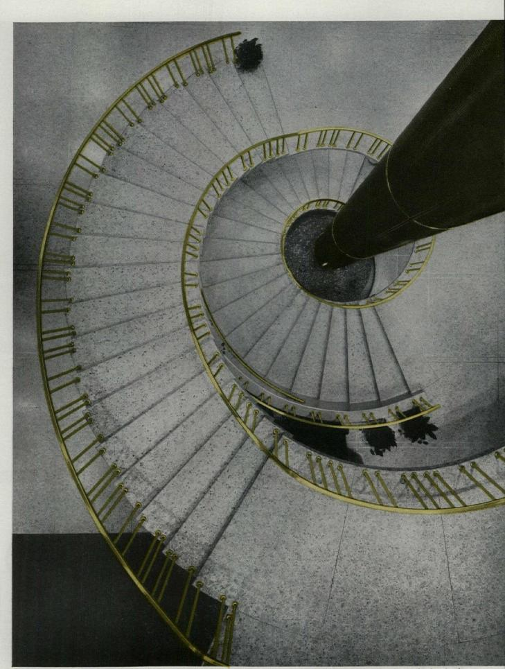
This graceful spiral stairway was used by Architect James S. Sudler of Denver to integrate several floor levels in a bank. The design and the color of the architectural metal help establish an air of friendliness-yet contribute dignity and a feeling of stability. The column is enwrapped with woven bronze wires that have been partially colored to give a pleasing black-and-gold effect.
