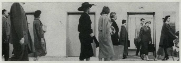
*"Everything* is automatic. The entire system is electronically controlled to serve passengers quickly, yet courteously. Traffic Sentinel Doors open automatically as car arrives. The doors remain open and motionless as long as necessary for passengers to leave or enter.
