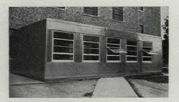
new unit is designed to accommodate 30 to 40 students. It is formed of two half-sections—each 40 feet long and 10 feet wide —which are simply bolted together. All wiring is installed and can be attached to the existing power source or to a portable generator. An oil-burning furnace mounted on the outside of the building (not shown in photo) supplies the heat. Cost: about \$16,000, or roughly half as much as a permanent, masonry room of the same size.
