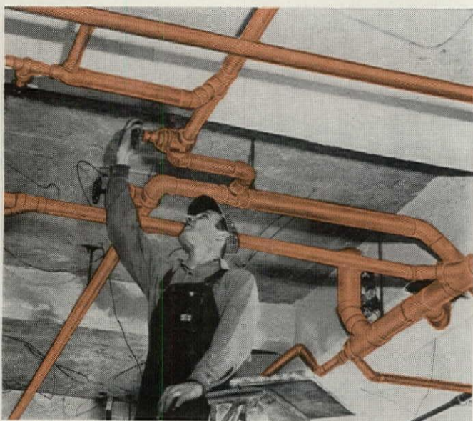
TESTING A VALVE on the hot-water supply system. Other copper tube lines in view are part of the sanitary drainage system, ranging in size from 1½ inches to 4 inches. Because connections are easily made, even in tight quarters, the lines can hug the ceiling.
