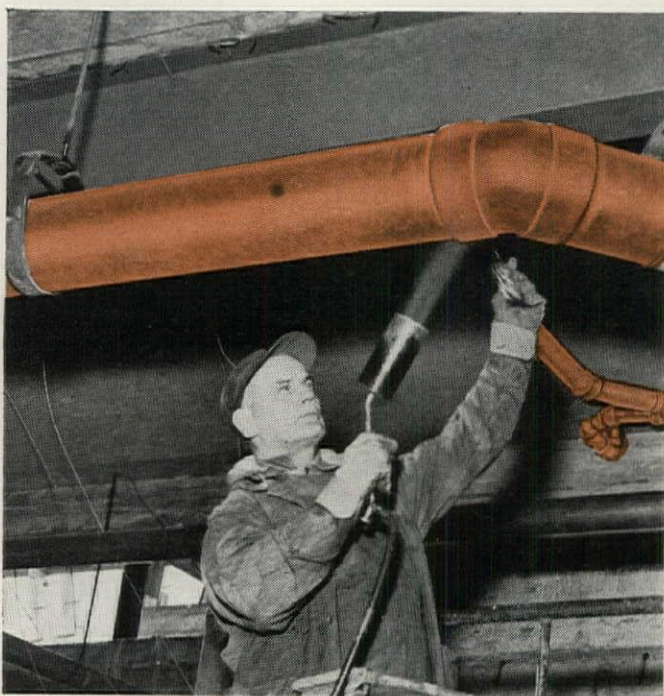
MAKING A SOLDER JOINT on an 8-inch copper soil and waste line — the largest size used in the drainage system. Solder-joint connections are one of the important reasons why copper tube systems are so much easier and faster to install.
