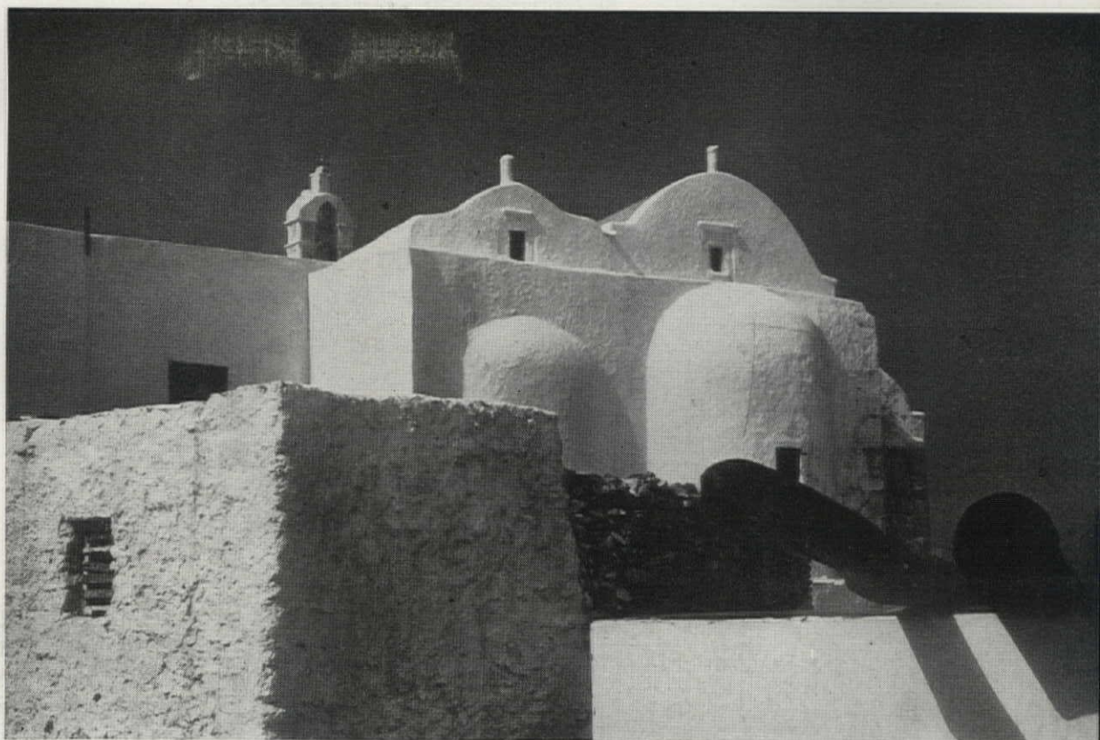
A house beneath a double-vaulted church shows the secret of Mykonos construction: rock walls plastered with whitewashed sand and dung.
