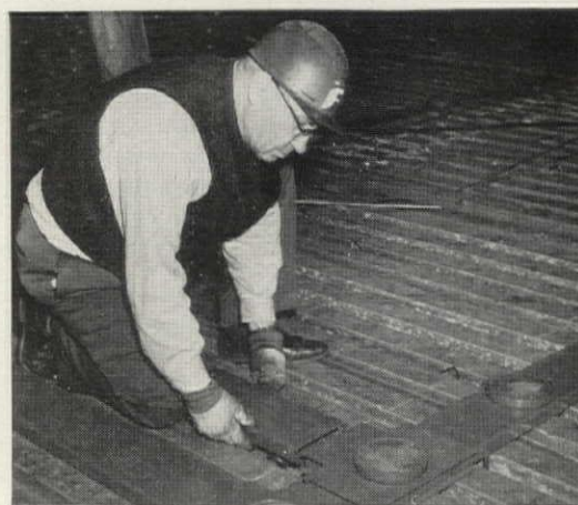
Electrical header duct carries electrical feeder, circuits from the distribution panel transversely across Celluflor cells. Definite patterns of service repetition are established so that proper raceways are easily located, when electric power, telephone, signal, or other service outlets are required in any floor area.
