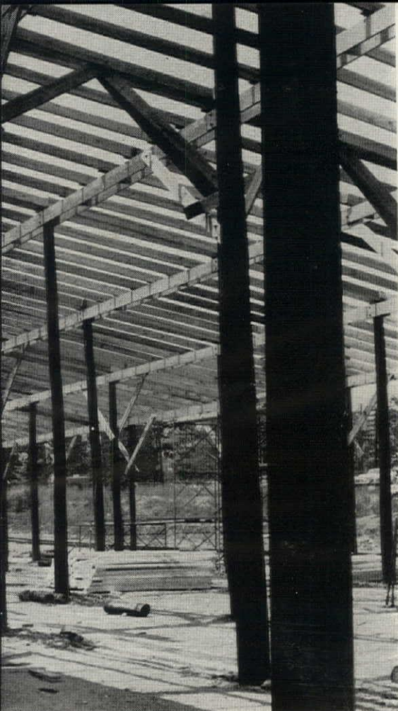
POLE WAREHOUSE (left), for Southern Chemical Cotton Co., Chattanooga, Tenn., has 184 pine poles spaced 14 ft. and 19 ft. With metal sheathing and roofing, 39,900 sq. ft. of warehouse came to $1.05 per sq. ft., without concrete floor.
