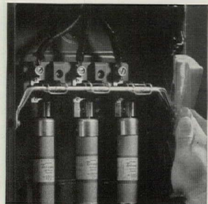
Bulldog Vacu-Break chamber smotheres arcs before they can cause damage. Both are 100-amp, 600-volt switches, operating under 90-ampere, 440-volt load with 40% to 50% power factor.
