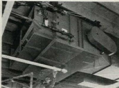
Close-up of Dunham-Bush 'HAH' which cools, heats, filters, dehumidifies air.
