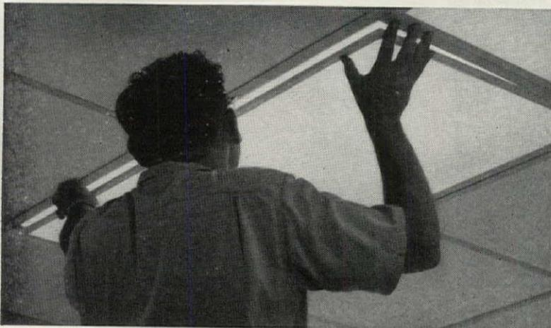
**The discomfort of direct and reflected glare is reduced** with Fiberglas Polarizing Light Panels, which also conform to the established ceiling module. The Fiberglas Polarizing Light Panel combines the two most sought-after properties in lighting control—cutting off direct glare like a lens or louver . . . and reducing reflected glare like a diffuser. The textured appearance of Fiberglas Polarizing Light Panels provides interesting, decorative effects which are architecturally neutral.
