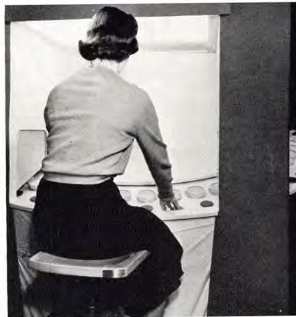
Revolving wheel helps the scientists to determine the eye's ability to see under dynamic conditions, such as reading or writing, where the eye is in motion.
