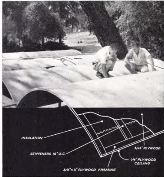
CURVED PANELS over living areas have same basic construction as flat panels. Underside serves as finish ceiling.
