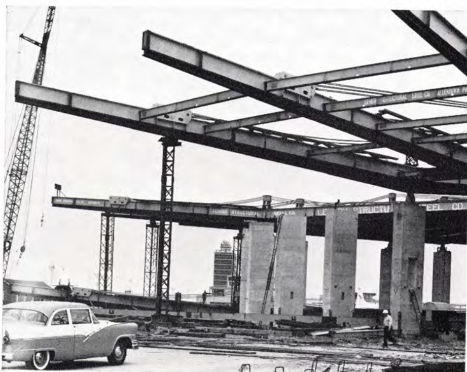
Girders are temporarily supported until anchored.
