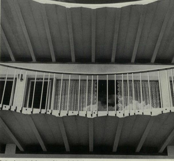
Prestressed concrete planks were used to span both the first story and the roof of the long narrow building.
