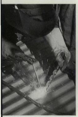
Exclusive Fab-Form Welding Washer Stick reduces installation time. After the end washer on the stick is bent up, the welder makes a plug weld and snaps off the washer. Then mesh is installed and slab is poured.
