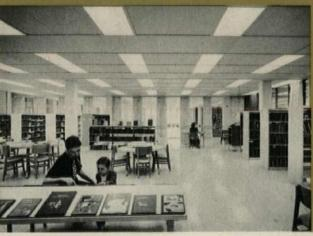
**Golden** is silence, too! Reynolds Aluminum perforated acoustical panels, pyramid type, are suspended from this Library's reading rooms. They serve both to control sound and as a diffuser for the air-conditioning system. Whether you are specifying for an educational, commercial or manufacturing building, consider the proved values of Aluminum.
