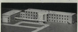
Model of Chapel and Novitiate Building, Brothers of the Holy Cross, Kinderhook, N. Y. Anaconda Type DWV copper drainage tube and Anaconda cast-brass drainage fittings were used on interior soil, waste, and vent lines. Architect: Toole and Angerame, Albany, N. Y. Plumbing and heating contractor: Farrell Bros., Albany, N. Y.
