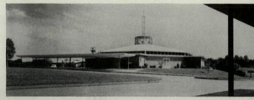
Octagonal auditorium roof fabricated from USS Structural Steel makes a pleasing design. This shape permits maximum seating close to altar.
