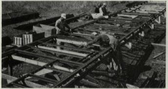
Eason, Anthony, McKinnie & Cox designed 31 Memphis project apartment buildings with Stran-Steel components. Sidewalls and trusses were assembled on wood jigs near building sites.
