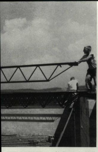
TRUSCON "O-T" STEEL JOIST was used in this construction, Attle W. Wampler & Sons Furniture Store, Baltimore, Md. E. S. Armacost & Son were the builders and designers. Truscon Wire Fabric, Bars, Structural Steel, Steeldeck, Series 57 Doors, Commercial Projected and Security Steel Windows, are other Truscon products that have been specified for the job.
