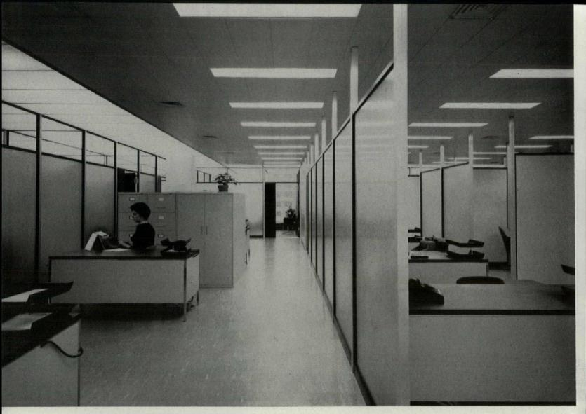
Well-lighted offices are a restrained buff white with black line accents. Hung ceilings, luminous at the perimeter, are plenums drawing return air in along the core (below), which neatly lines up services at the back of each office floor (see plan, right).
