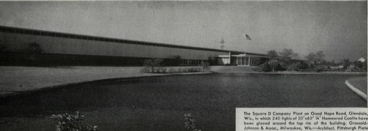
The Square D Company Plant on Good Hope Road, Glendale, Wis., in which 240 lights of 30°x60° ¼° Hammered Coolite have been glazed around the top rim of the building. Grassold-Johnson & Assoc., Milwaukee, Wis.—Architect. Pittsburgh Plate Glass Co., Milwaukee, Wis.—Glazing.
