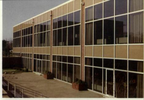
Façade of glass. Even the spandrels are glass—*Vitrolux®* heat-tempered polished plate glass with ceramic color fused to the back.
