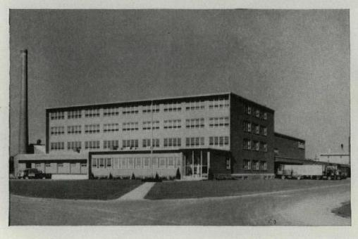
Borden Foods Company, Plymouth, Wis. South, east, and west elevations glazed with ½' Mississippi Lux-lite Coolite, Heat Absorbing Glass. Cowell & Robinson, New York, N. Y., — Architects-Engineers. McDonough Construction Company of Georgia—Contractors.
