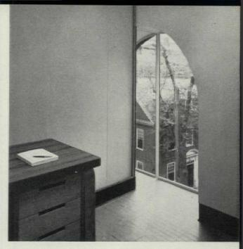
Window detail illustrates how old arched openings provided light for four offices. Arched opening is cut horizontally by new floor, split vertically by new 1½-inch gypsum partitions. Mirror on partition in arch adds apparent size to window.
