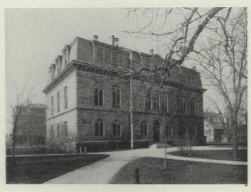
Exterior before and after (above and below) shows little change except for new fixed glass filled into the old stone arches formerly filled with heavy wood sash. Stone walls were left as they were, marked with the patina of a century's weather.
