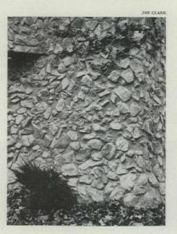
willing to try it, finally remembered hearing of an obscure firm, Prepakt Concrete Co., that repairs dams and other works by pumping in concrete around rubble. He tracked them to Cleveland, and they are now enthusiastic collaborators. The main trick is to use an expanding agent in the grout to prevent it from contracting on setting, thus tightly bonding the stones.
