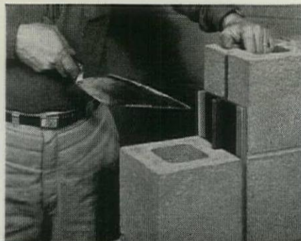
Two engineered products that meet a need. Dur-o-wal reinforcement, shown above, and Rapid Control Joint, below. Weatherproof neoprene flanges on the latter flex with the joint, simplify the caulking problem.
