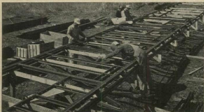
Eason, Anthony, McKinnie & Cox designed 31 Memphis project apartment buildings with Stran-Steel components. Sidewalls and trusses were assembled on wood jigs near building sites.
