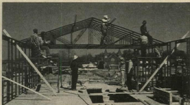
Every five minutes, workers lifted 31' trusses weighing only 140 pounds into place—including welding to the top channel of the load-bearing wall.
