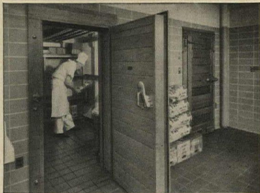
Both walk-in refrigerators are insulated with Styrofoam.
