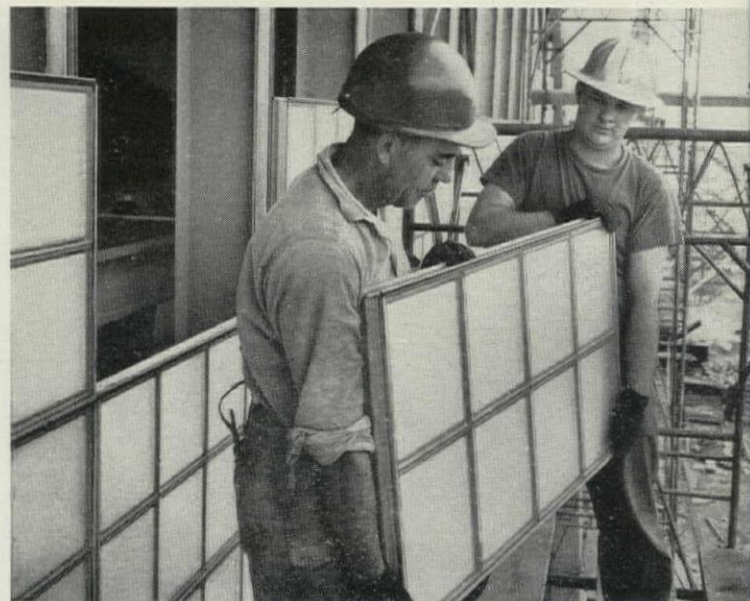
IN THE EARLY STAGES, Thinlite prefabricated panels fill the arches on Northeast and Southeast side of Project Turnkey.
