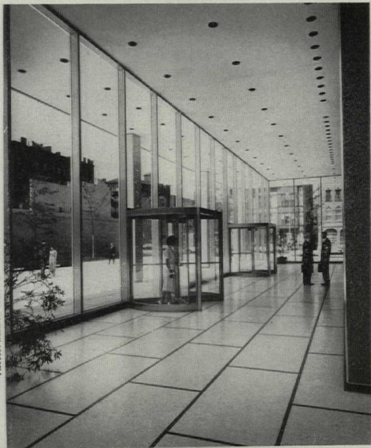
Terrazzo floor panels, 3 by 6 feet in size, march through the lobby . . .
