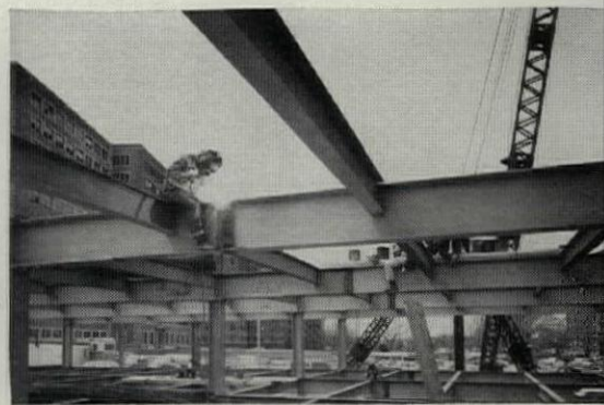
24-inch main carrying members being welded with 100% full penetration butt weld.
