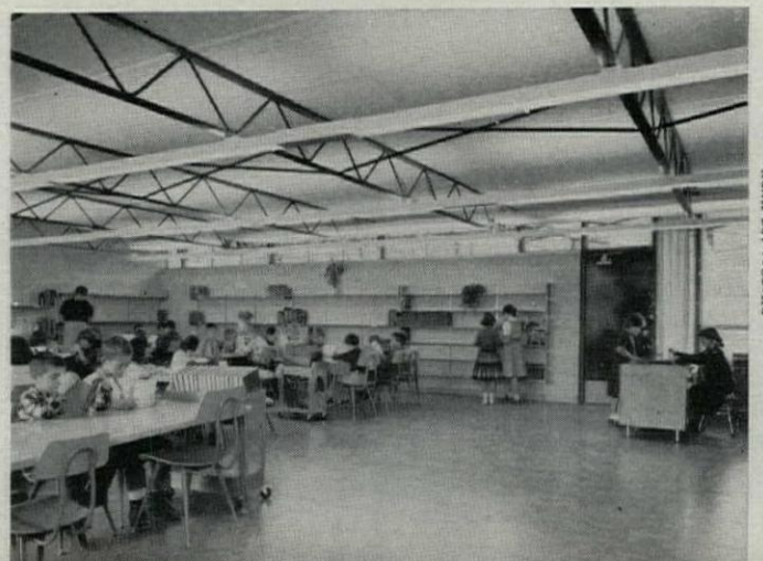
Light troffers run perpendicular to open-web joists in library.
