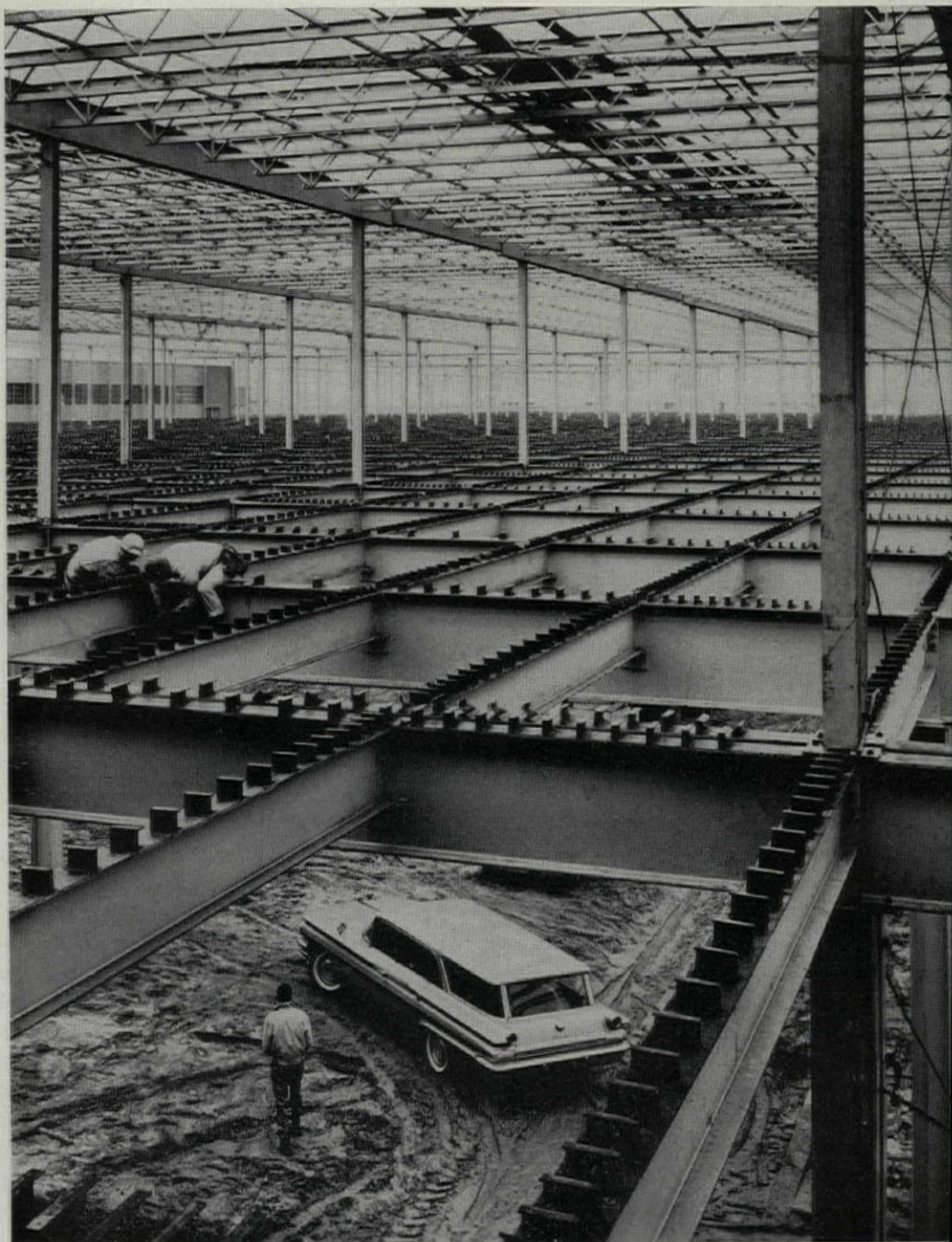
Channel-shaped connectors were used in the composite design of this huge plant for Steelcase, Inc., in Grand Rapids, designed by J. and G. Daverman Co., architects and engineers. Building uses 3,400 tons of structural steel.
