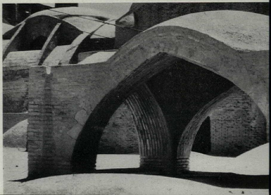
Using very adhesive mortar, masons threw these vaults without centering.
