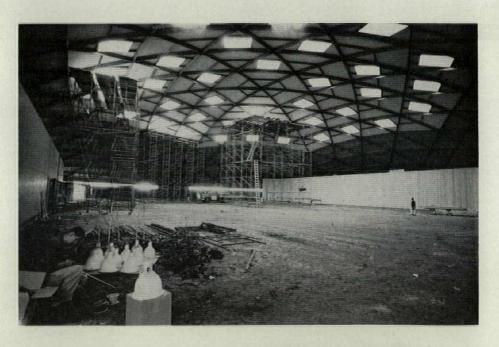
Field house spans 200 feet on 4 in. by 14 in. laminated timbers and a 2 in. wood deck. Lower walls shield special exercise areas and locker rooms. The treated dirt floor will have a running track, demountable basketball court and bleachers, room for an "all-sports, all-students" program
