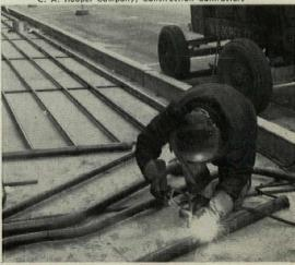
Easily formed and joined steel pipe, imbedded in concrete, circulates hot liquid that keeps the sidewalk summer-safe
