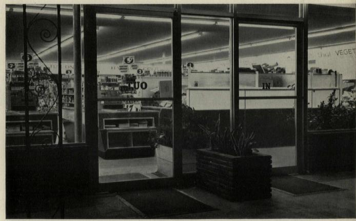
TUBELITE DOORS installed in a PPG Open-Vision front—Harris' Super Market, Waycross, Georgia. PPG's heavy-duty, high-traffic Tubelite entrances have concealed channel type anchors which keep frame seams to a hair line. Door trames have an exclusive interlocking feature that insures rigidity. For shopper convenience, doors are mat operated by PPG's Pittcomatic automatic door opener. Contractor: Business, Inc., Waycross, Georgia.
