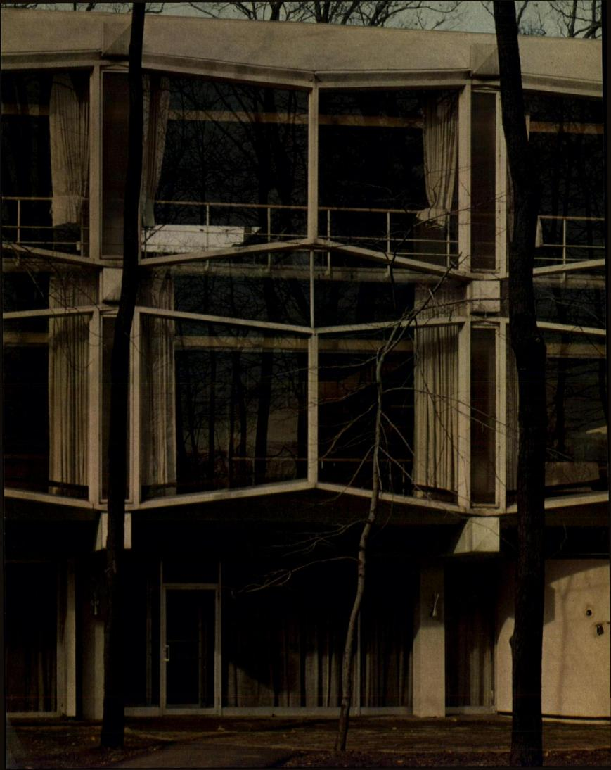
Exterior folded plane of tubular steel and glass is fastened only to the cantilevered ends of the fireproofed steel beams which support the second floor. Some sections of this curtain wall open, but the main ventilation of the buildings is forced, through ducts. The duct returns for the two upper floors are in the hung ceiling.
