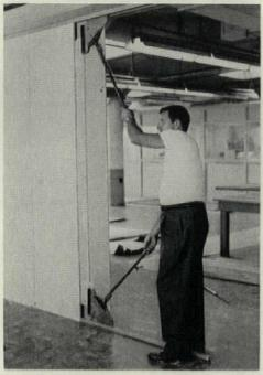
Movable Pabcowall panel being jacked into position between ceiling and floor strips.
