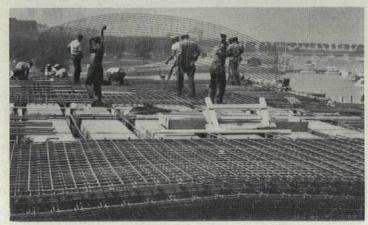
The cast-in-place pan-type reinforced concrete floor is designed for a live load of 400 psi.
