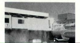
Other nozzles beneath the bridge spray water down onto the concrete apron and wash away burning fuel. Each of eight loading bridges at the terminal is equipped with the spray system.
