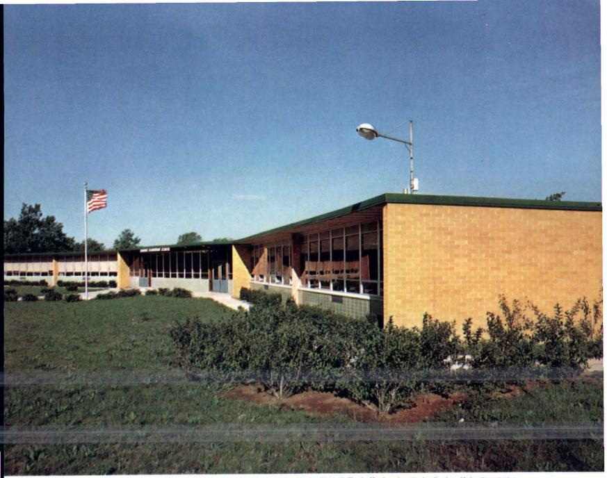
View of the modern Ivanhoe Elementary School in Gary, Indiana, showing its walls of Natco Uniwall. The buff colored vertical walls show Uniwall's exterior rugg-tex finish. The light green panels under windows show a unique use of Uniwall's interior face installed in reverse. Architect: Jos. P. Martin & Assoc.
