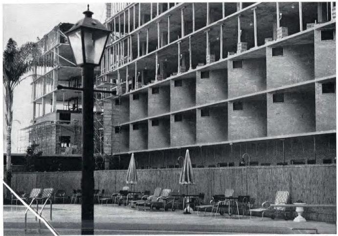
Installation is easy. Galvanized steel sleeves for General Electric Heat Pump Air Condi Moning units are built in during construc-
