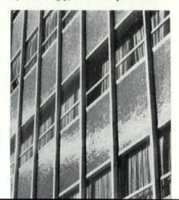
Panels may be specified in several Mosaic Tile types, and may be designed to fit all standard curtain-wall systems. The recommended maximum panel size is 4 by 8 feet. The in-place cost is about \$3 to \$3.75 per square foot.
