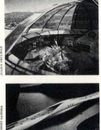
Domed desert house by Soleri and Mark Mills (top) was built ten years ago. Tubular bridge (bottom) was designed by Soleri in the late forties; it unfolds where structural stresses are small, closes back into tube shape at midspans. Opposite: detail of formwork for Soleri's new "earth houses."
