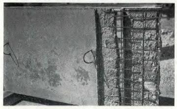
concrete reinforcement of the pan-type floor construction. The floor is designed for 400 psi live loads with columns at 60-ft. centers. The joists are 14" deep with the top 41/2" slab reinforced with welded wire fabric sheets. Welded wire fabric reinforcement was also used in the construction of the ground floor slabs, terrazzo floors and gypsum roof decks.
