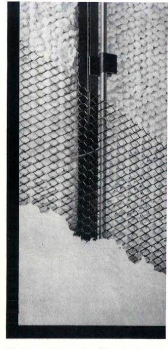
**New slim sound-isolating partition**—This partition develops a 42 db sound rating in 2%" thickness by attaching a pencil rod to a ¾" channel stud with Resilient Clips. Finished with metal lath and plaster on both sides.
