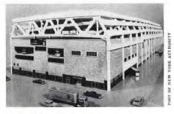
GIANT TRUSSES will support three new auto-parking decks over Port Authority bus terminal in New York without placing any additional load on remodeled structure below.
