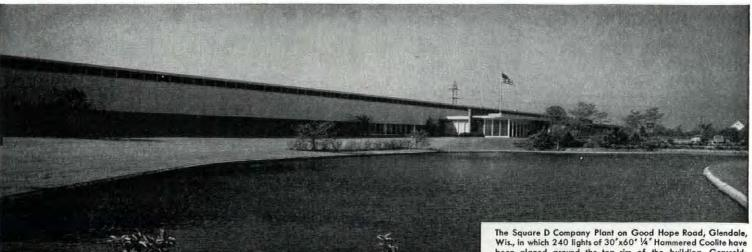
The Square D Company Plant on Good Hope Road, Glendale, Wis., in which 240 lights of 30<sup>°</sup>x60<sup>°</sup> <sup>1</sup>/4<sup>°</sup> Hammered Coolite have been glazed around the top rim of the building. Grassold-Johnson & Assoc., Milwaukee, Wis.—Architect. Pittsburgh Plate Glass Co., Milwaukee, Wis.—Glazing.
