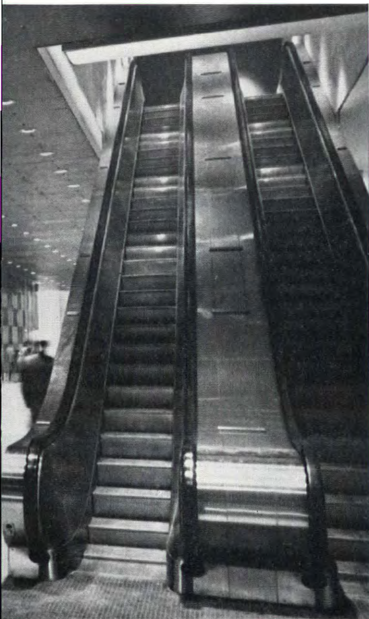
GENERAL BRONZE CORPORATION fabricated more than 20 tons of Republic Stainless Steel (Type 302 with a 2B finish) for wall- and column-panels, entrance ways, elevator doors, and other applications. Time & Life Building, Rockefeller Center, New York 20, New York.
