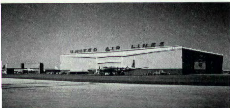
Wash hangar, at left of the main hangar (above), is framed in a delicately detailed skeleton of welded steel.
