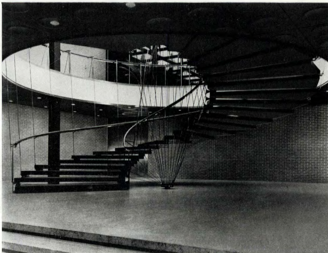
Suspended stairway in administration building of leading manufacturer relies on the supporting strength of Type 18-8 Nickel Stainless Steel rods.
