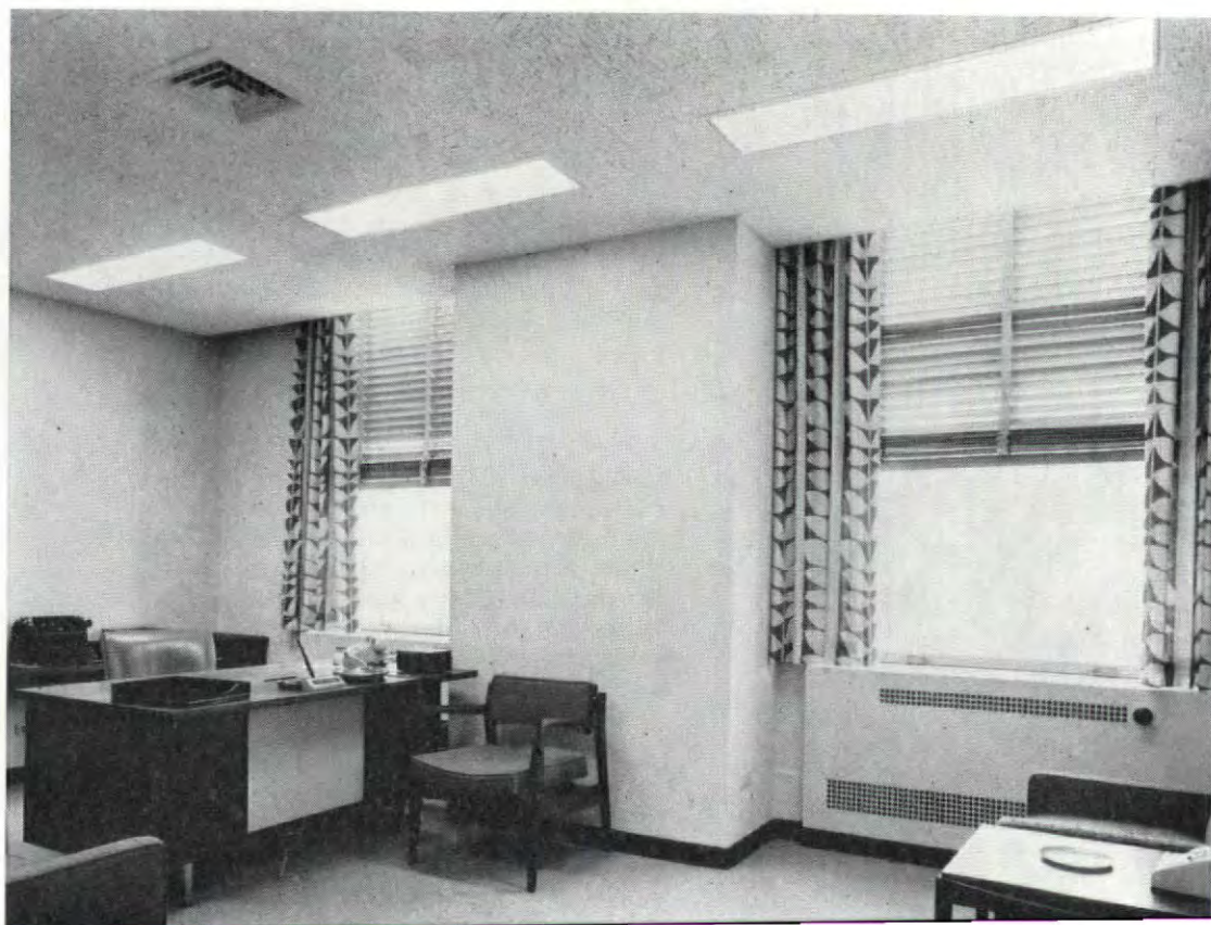
Offices in the redesigned building (right) use existing radiators to supplement the hot-and-cold-air system. Old lighting (above) has been replaced with flush fixtures yielding an illumination level of 45 and 50 foot-candles.
