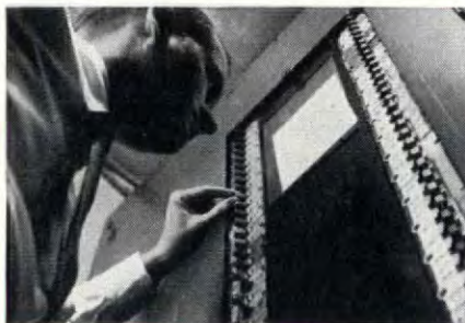
Old system controlling corridor lights required manual operation of panel switches on 33 floors. A half-hour job!
