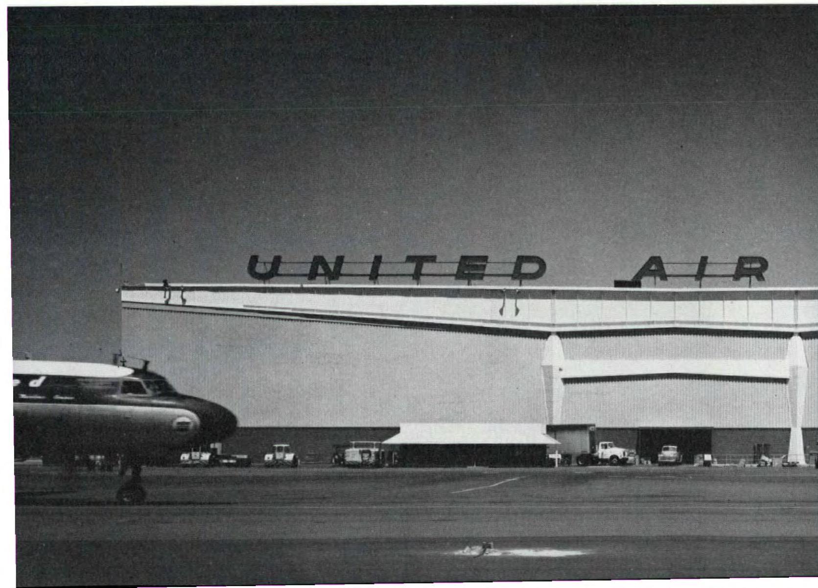
Sheathed in metal, the structure is expressed clearly on the façade.
