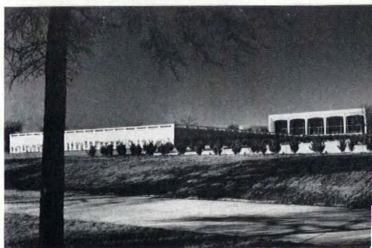
Granite retaining walls of the plaza form pedestal for building.
