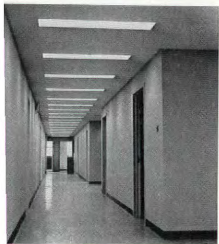
Corridors seem brighter, broader than their 6-foot width after air conditioning and new lighting were installed in the ceilings, which were dropped from 8 feet, 6 inches to 7 feet, 10 inches.
