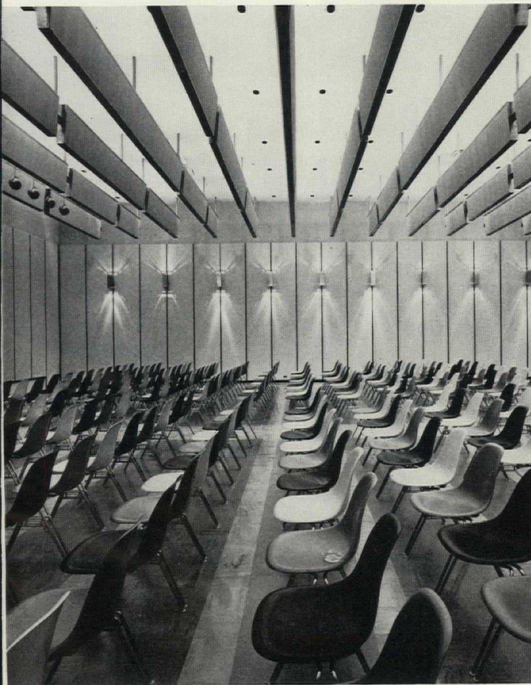
Main-floor auditorium has ceiling sound baffles and elaborate spotlighting.
