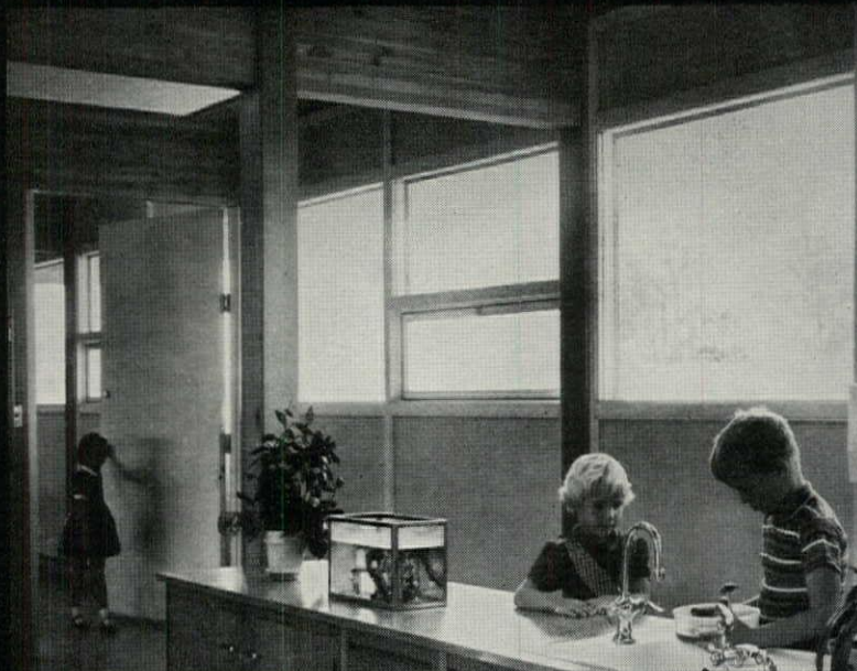
Shown in this interior view is one of the 8' doors that open between each classroom. All Steelcraft doors can be prepared for choice of hardware such as panic devices, and concealed closures, trim and finish—and are available with standard cutout for cylindrical, mortise, unit and integra-locks. Note the steel, hopper-type window, fitted into the metal frame.
