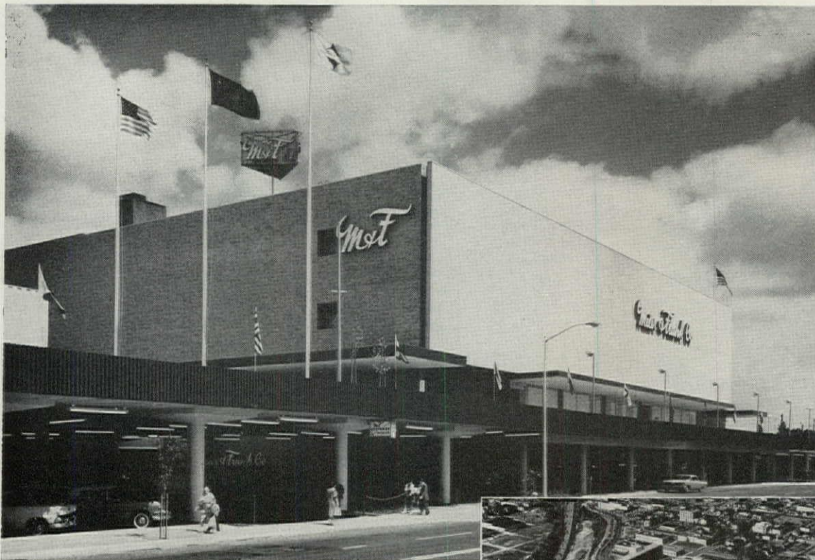
The huge Lloyd Center, Portland, Oregon—one of the nation's largest shopping centers. Round concrete columns used for supports throughout ground levels. Developers: Lloyd Corporation, Ltd. Architects & Engineers: John Graham & Co. Prime Contractors: Donald M. Drake Co. and Max J. Kuney Co.
