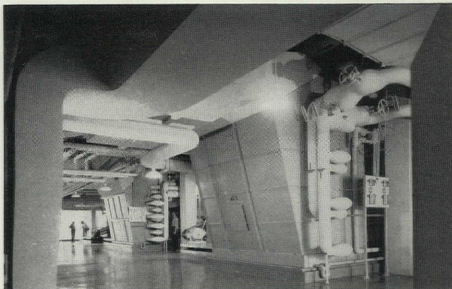
Air-conditioning and ventilating equipment inhales and exhales as much as 200,000 cu. ft. of air per minute.
