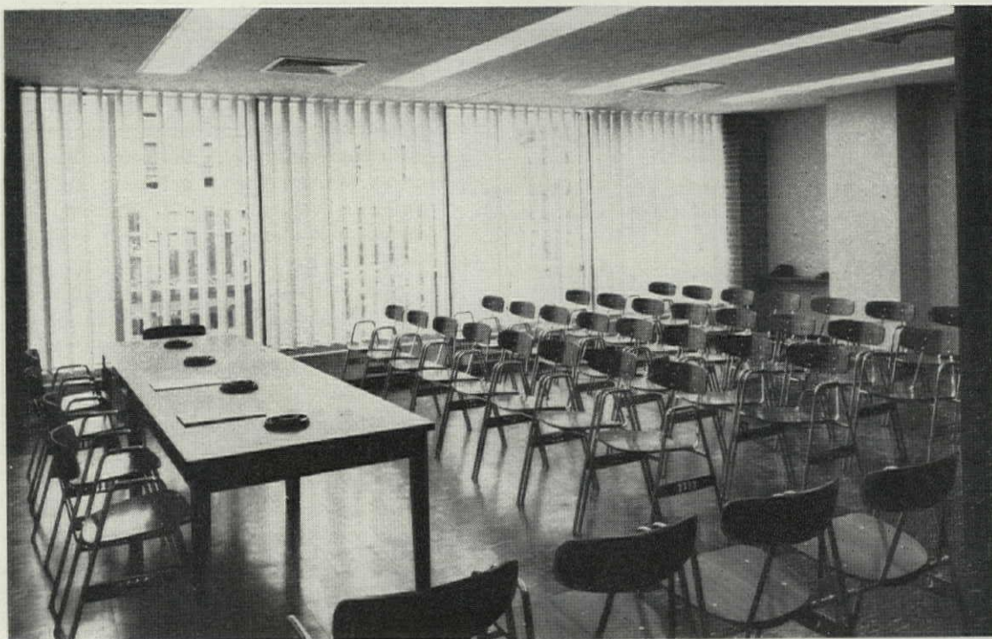
Vertical Venetian blinds throughout screen the sun and reduce air-conditioning loads.
