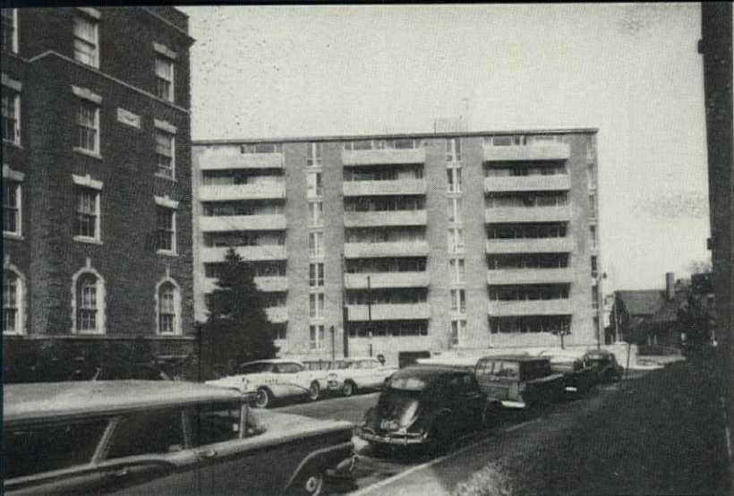
Construction is flat two-way slab with balconies on seven floors.
