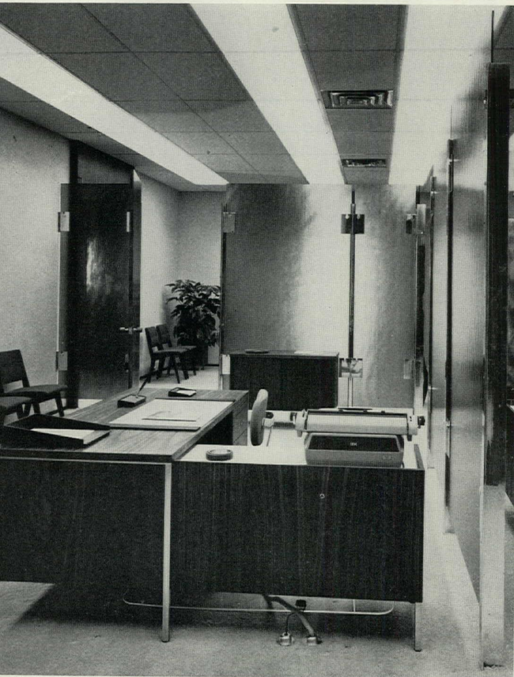
Ordinary offices have newly developed fluorescent fixtures, recessed in fiberboard ceiling.
