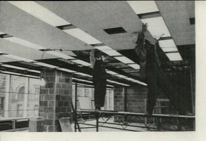
Air conditioning is delivered between aluminum lighting fixtures in the ceilings of inner office areas (above) and underwindow induction units along the outside walls (plan below). Ceiling diffusers are fed from the ceiling above; window units, from the floor below.
