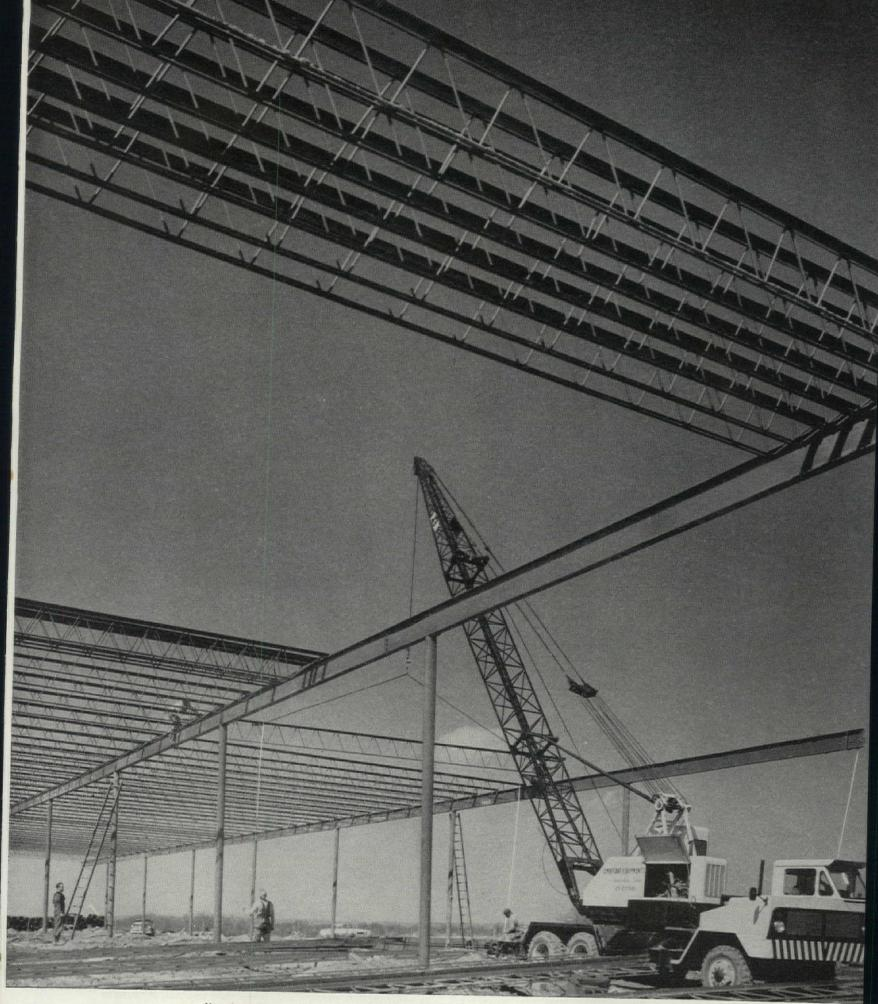
New plant of Dominion Electric Corporation, Gallatin, Tennessee, under construction by General Builders Corporation, Nashville, Tennessee. Higher strength USS A36 Steel Beams saved 6 tons of steel. Note simplicity of design.
