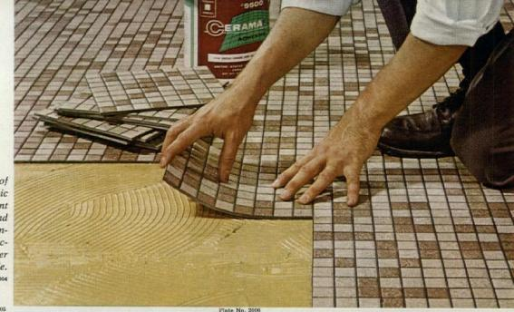
CERAMAFLEX®... newest development of Romany\*Spartan research. Sixty-four ceramic mosaic tiles securely bonded in a resilient rubber grid, pre-grouted and laid quickly and inexpensively in 9" squares. Quiet and comfortable underfoot. Choose from 12 attractive Buckshof® patterns for installation over any sound sub-floor above, on or below grade.
