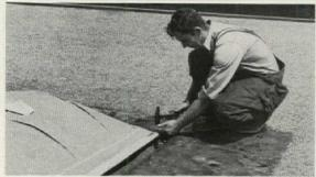
Twin Dome is installed in 15 minutes. Continuous 3" flange is nailed to roof deck, covered with 4 alternating layers of mastic and roofing felt, plus hot tar, gravel.
