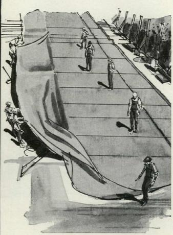
protection for Building foundations from both hydrostatic pressure and water infiltration is provided by sheeting of Enjay Butyl rubber. Butyl's high tear strength withstands rough handling on the job site.
