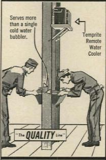
TEMPRITE REMOTE COOLERS mount overhead or behind a wall to save floor space and prevent possible damage to cooler from lift trucks and moving equipment. Models available with water-cooled condensers for use in confined areas or where dust or lint-laden air prevails.
