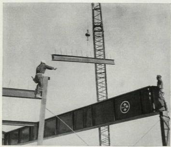
The five long-span girders, 106 feet, 8 inches, are joined to intermediate and peripheral framing to form the hexagonal roof support. General contractor for the entire project was Dickie Construction Company, St. Louis, Missouri.
