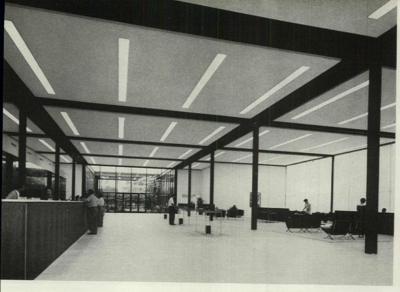
The McAllen State Bank in McAllen, Tex. stands serenely on a marble platform. Its big, high, single-story space is defined, inside and out, by the exposed welded steel frame, and is penetrated by a courtyard (above, right). Cowell & Neuhaus, architects.
