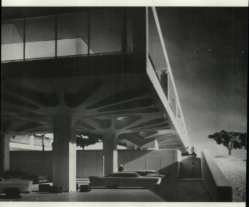
Treelike columns of concrete were redesigned after model (photo above) was built. Now four ribs in each capital support 42-foot-square floor sections (drawings, right). Fascias are white aggregate; fixed glass is gray. Retaining walls are granite aggregate.
