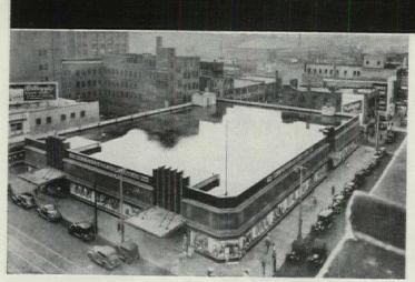
This 27 year old store of the J. C. Penney Company in Milwaukee has been given a million-dollar-plus remodeling job which involved everything but the water-cooled roof. Although the Koppers coal-tar pitch roof has been constantly under water for 27 summers, it is still in excellent condition, and should last many more years.
