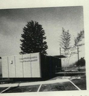
Seattle First National's Tukwila branch is one of four portable units called "interim banks" for locations where small buildings will soon be outgrown. Like the portable shown on page 106, this is a steel-framed box, in this case formed of rigid tubing except for the main girders. Panels are redwood, glass, and reinforced plastics. Steinhart, Theriault & Anderson, architects.
