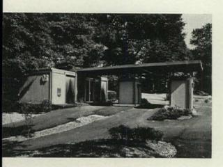
Brookwood Office of Citizens & Southern National Bank, Atlanta, called the "instant bank," is a portable building to which portable drive-in units are attached. The structure is a steel-framed box taking a system of panels. Toombs, Amisano & Wells, architects.
