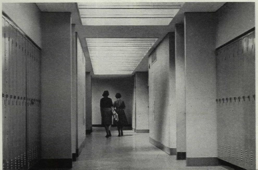
"Glass attic" scheme (see section, top) daylights classrooms (above), corridor (below).
