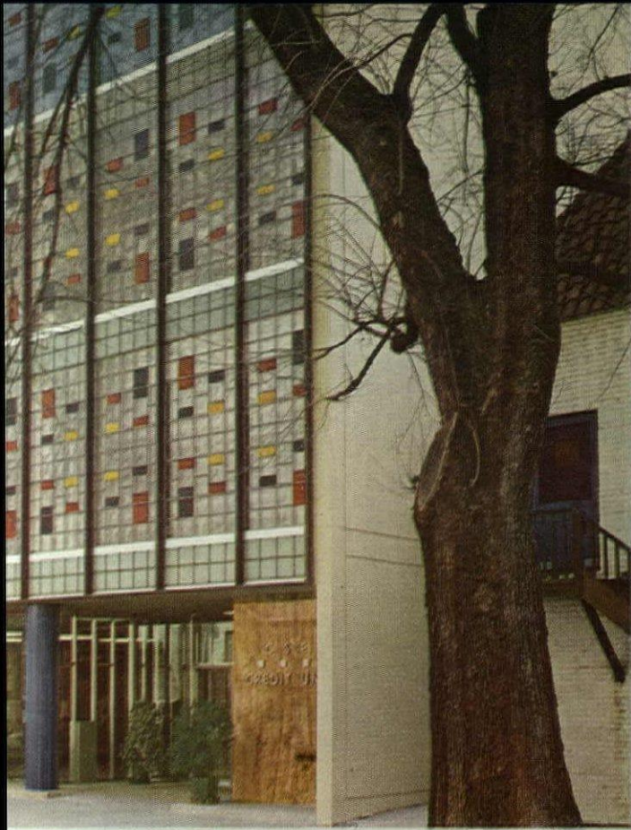
Thinlite panels of Clear Vista accented with ceramic colors, admit maximum light with low heat transmission in the new office building of the State Employees Building Corporation, Sacramento, Calif. West America Engineering Company, Inc., San Francisco, designed the structure.
