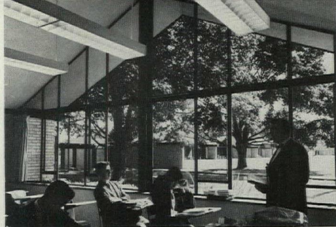
Typical classrooms have one full wall of glass rising to the gable roof, which is repeated over each pair of classrooms on a 24-foot module. Structure is of steel beams supporting wood rafters.
