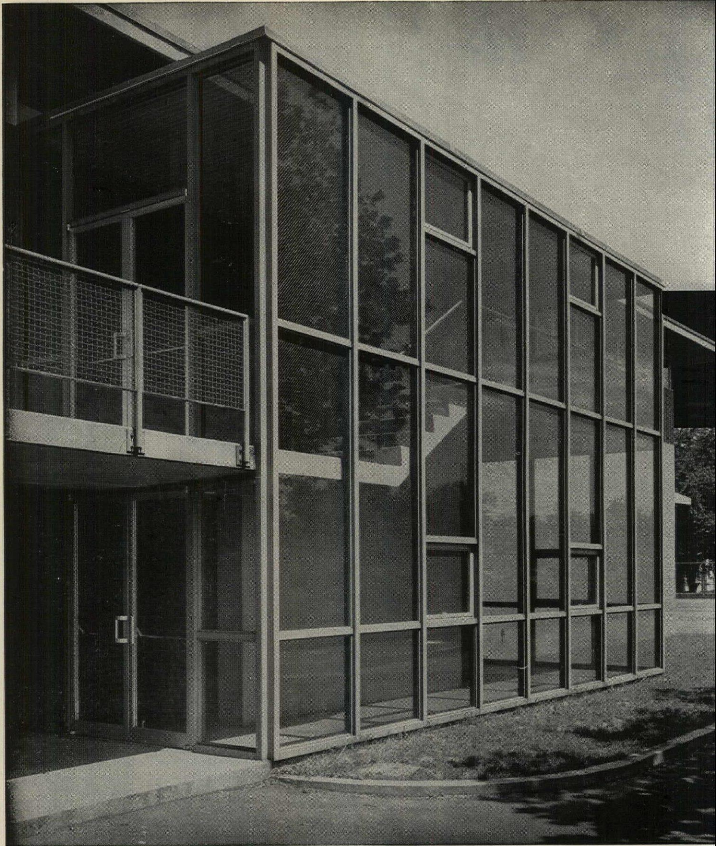
Stairwell of Polished Misco Wire Glass contributes to overall appearance as well as safety in the Fort Saunders Elementary School, Knoxville, Tenn. Architect—Painter, Weeks & McCarty, Knoxville, Tenn.
