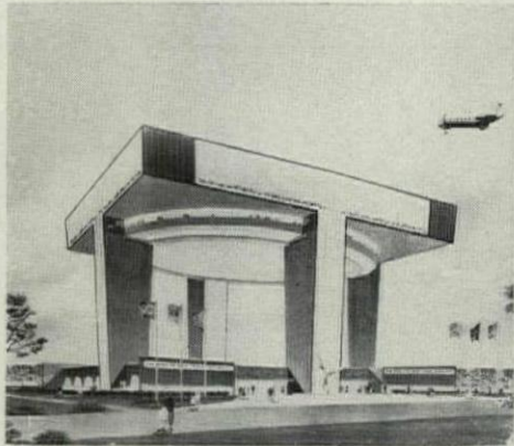
Port of New York Authority building, a heliport on four massive stilts, with a restaurant hung beneath landing platform.
