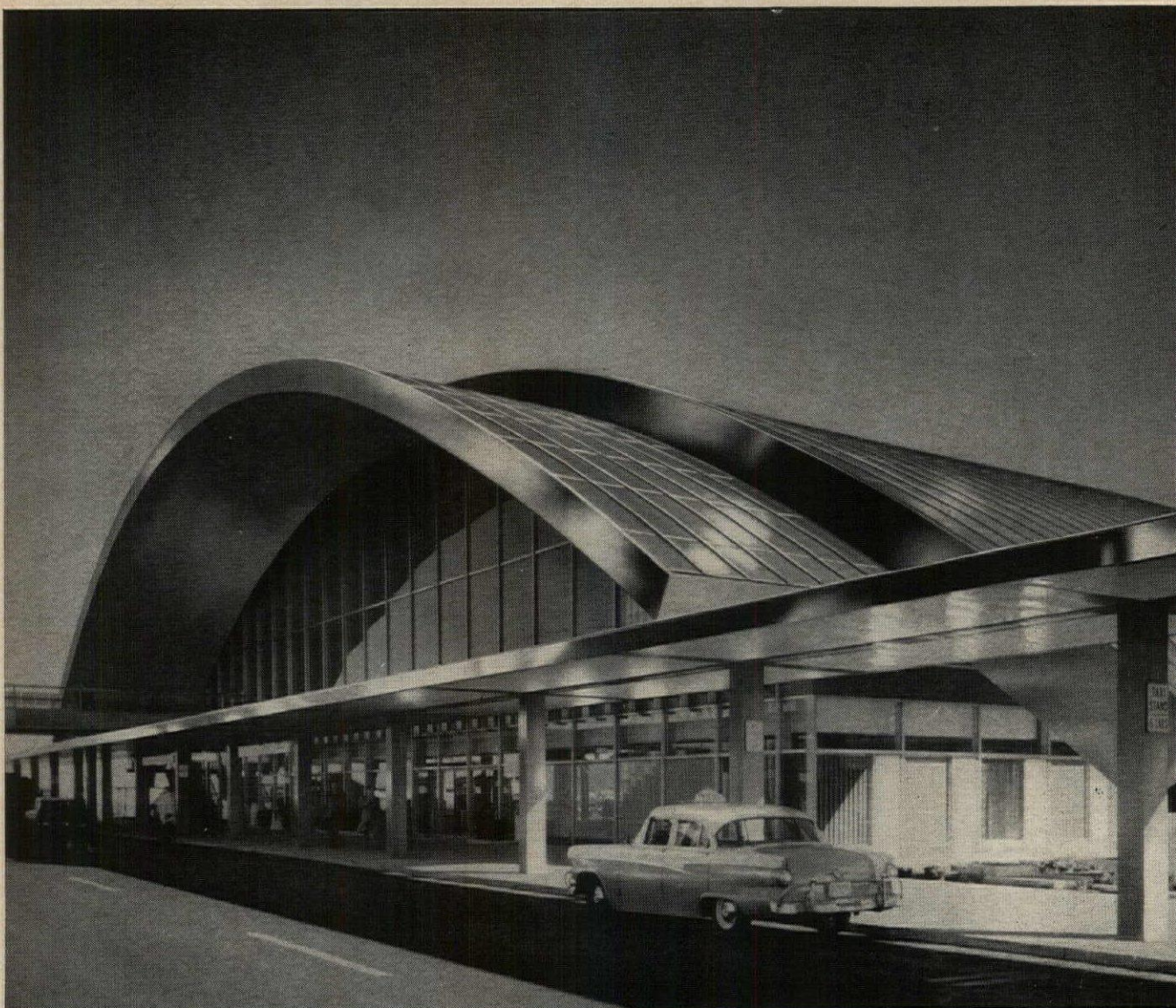
International Arrivals Building of New York International Airport. Arch is sheathed with 24-gauge, No. 2D special finish, Type 302 Nickel Stainless Steel. Architects: Skidmore, Owings
