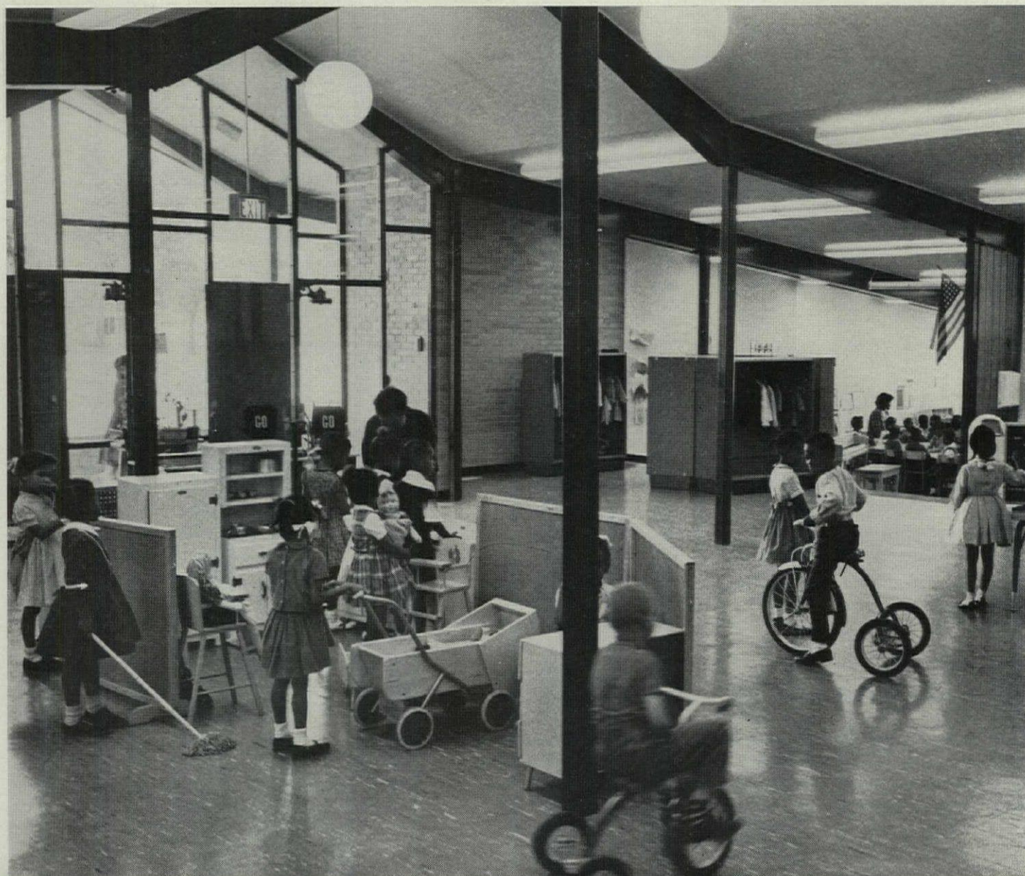
Kindergarten commons (below), used jointly by four classes, occupies a portion of the central "corridor" and corresponds to the library commons for older classes shown on the opposite page. The gable roof is formed of steel beams carrying wood joists.
