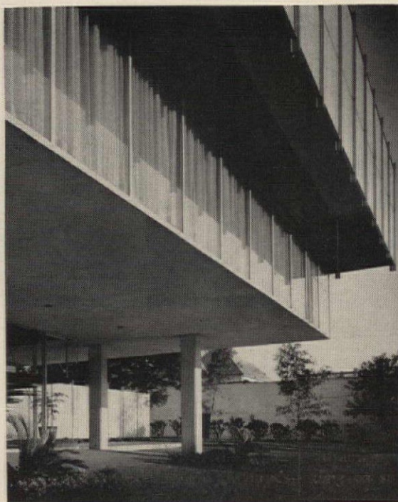
Building elevation will be symmetrical after expansion (see plan, page 90). Section (right) shows how glazing was pulled down to hide the floor slab. Gap measures 4½ inches, serves as pocket for curtains. Sun screen also screens out views of undistinguished surroundings.
