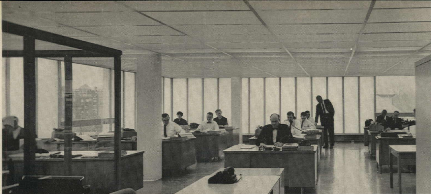
Luminous ceiling (above) draws exhaust air from the building through the fixtures, thus cooling the ballasts to prolong fixture life
