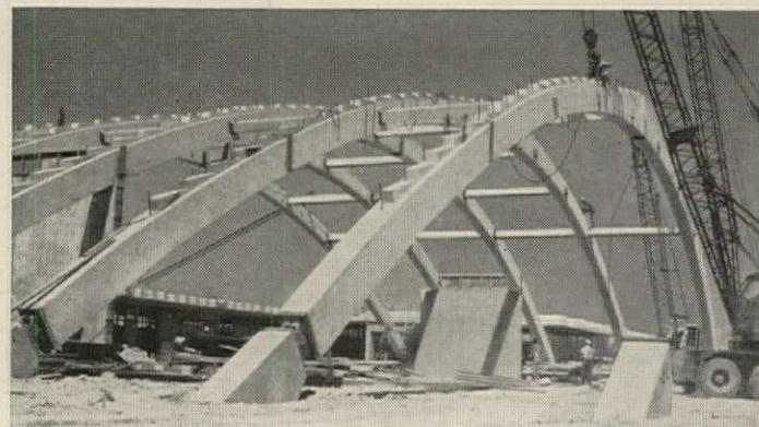
Each of the arches spans 160' and is spaced 16' center to center. The arch skeleton is braced by precast lateral members with welded connections. Gym floor space is 12,000 sq. ft., and there is a 10' wide covered walkway on each side. Note "steps" and projecting dowels cast into arches for securing roof panels.
