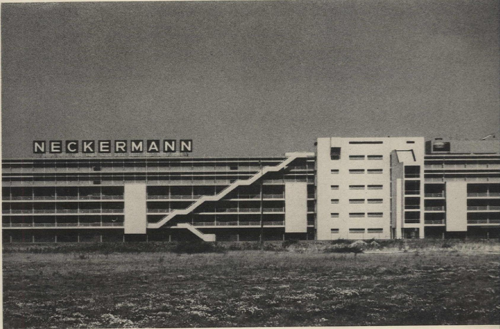
four service cores were too far apart to allow satisfactory emergency egress. The architect's solution, stamped clearly on the façades, was to rim the building with galleries which lead to free-hanging exterior stairs, two on each long side.
