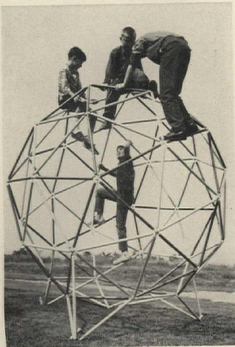
cartons ready for assembly, both versions require only pliers and a wrench to bolt the metal connectors together. Equal-sized struts are hardwood dowels with a red and yellow baked enamel finish.
