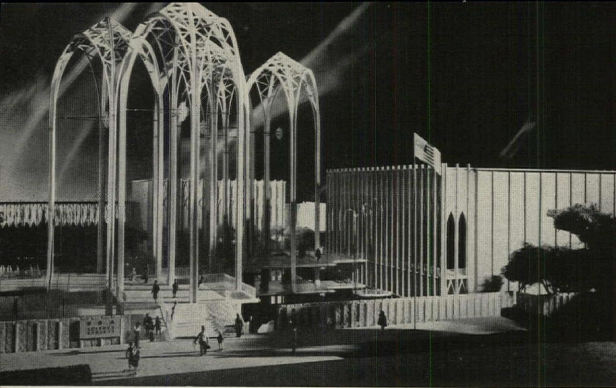
▲ **WORLD'S LARGEST SCIENCE EXHIBIT** is housed in Federal Science Pavilion constructed entirely of precast, prestressed concrete components made with 'Incor' 24-hour Cement.
