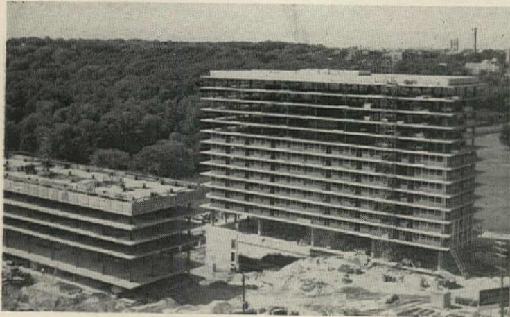
more stories were added to the columns' height and the process was repeated. A truck-mounted crane drove around the top slab during its slow ascent lifting steel for the columns and other building components. As each of the slabs reached position, it was welded and grouted to the columns in a permanent bond. Twenty weeks elapsed before the highest slab was in place, during which time other work was, of course, proceeding on lower floors.
