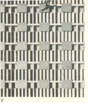
Klumb uses louvers and screens for sunshading (photos 1, 6), for security (photos 3, 5), to disguise unit air conditioners which will be inserted later (photo 2), and sometimes, side by side, for several reasons (photo 6). The climate frequently permits him the real architectural luxury of ending rooms without a wall, even a glass one (photo 4).
