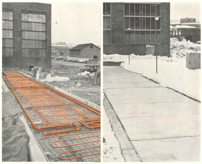
Anaconda Preformed Copper Tube Grids installed in sidewalk . . . and 6 months later a 10" snowfall is quickly melted.
