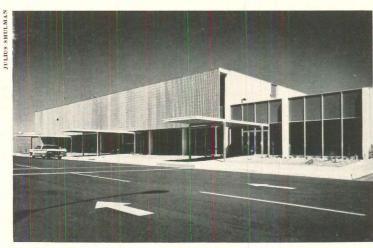
SYRACUSE TERMINAL (above), at a concrete deck, completes the Clarence E. Hancock Airport in structure, which is walled in brick upper New York State, was deand glass framed in aluminum. signed by Architects Ketcham-The terminal building is part of Miller-Arnold. The building sits a three-stage, \$5 million improvement program which includes under a big folded-plate concrete roof supported by exposed coneverything from approach roads crete columns. Steel skeletal framto new runways. General con-
