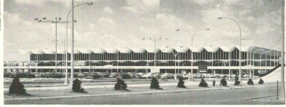
**MINNEAPOLIS-SAINT PAUL** International Airport Terminal at Wold Chamberlain Field, designed by Cerny Associates, Inc., is a 485 by 245-foot, two-story structure sheltered by an immense folded roof of thin shell, lightweight concrete. An important part of the design is a four-lane approach highway elevated to the secondstory concourse level and canopied by continuous umbrella shapes. Two elevated finger walkways lead to planes. General contractor, Foley Bros. Inc.
