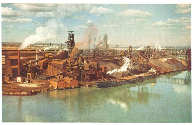
McLouth's Trenton, Michigan plant showing sintering plant, blast furnaces, ore docks and bridges.
