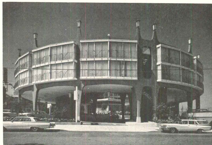
SAN FRANCISCO MOTEL. Floating on precast concrete stilts 20 feet aboveground, the new Columbus Avenue Motel has opened for business a few blocks from San Francisco's Fisherman's Wharf. Automobiles drive underneath to park around a central court, where there is a raised pavilion containing a bar and lounge. The 47 bedrooms and 12 living rooms have shallow bay windows with exterior railings and sliding glass doors. Perched atop the modern structure, somewhat incongruously, are old-fashioned carriage lamps. Cost: about $600,000. Architects: Anshen & Allen. Engineers: Robert D. Dewell (structural); K. T. Belotelkin & Associates (mechanical); Charles Krieger (electrical). Owner and builder: Stolte, Inc.
