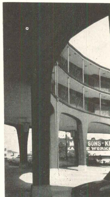
SAN FRANCISCO MOTEL. Floating on precast concrete stilts 20 feet aboveground, the new Columbus Avenue Motel has opened for business a few blocks from San Francisco's Fisherman's Wharf. Automobiles drive underneath to park around a central court, where there is a raised pavilion containing a bar and lounge. The 47 bedrooms and 12 living rooms have shallow bay windows with exterior railings and sliding glass doors. Perched atop the modern structure, somewhat incongruously, are old-fashioned carriage lamps. Cost: about $600,000. Architects: Anshen & Allen. Engineers: Robert D. Dewell (structural); K. T. Belotelkin & Associates (mechanical); Charles Krieger (electrical). Owner and builder: Stolte, Inc.
