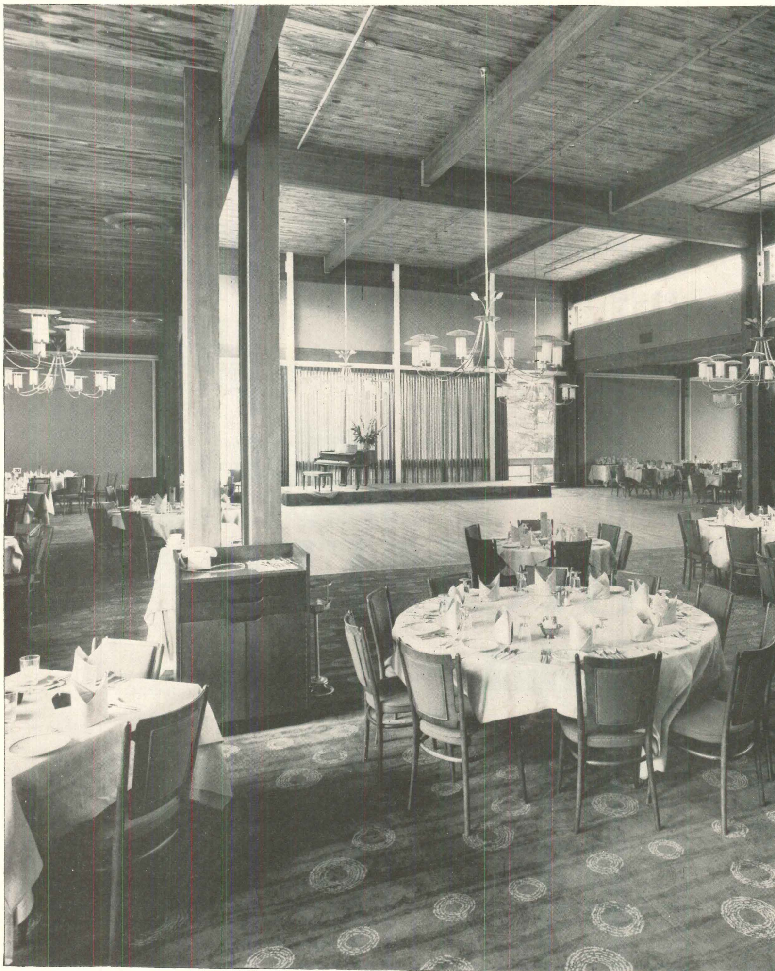
Lengthy laminated beams, dual-post supports, and a multi-toned planked ceiling create spacious luxury in the club's high clerestory-lighted room for dining and dancing. Wood's natural resiliency adds to dance floor pleasures, too. Interior Decoration; R. F. Associates.
