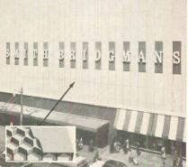
STORE FRONTS. Save on store front modernization and construction with UNION HONEY-COMB. Decorative lightweight panels are extremely durable. They can be faced with stainless steel, aluminum, porcelain enamel, etc. HONEYCOMB store fronts combat moisture, resist temperature extremes and weathering.
