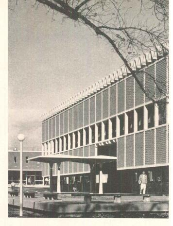
The attractive and unusual entryways are made of precast concrete elements manufactured at the job site, using Lone Star Portland Cement.
