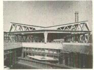
buses at the base and maximum bearing area for the four trusses which come together overhead. A single form was used for all six columns; it was made with thin boards lovingly tapered and fitted in a cabinet maker's shop.
