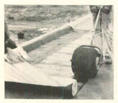
Bitumagic goes down quickly, then is rolled or brushed to assure uniform adhesion (see photo), and topped with a coat of cold-applied emulsion. It may be used as a continuous roofing-flashing system or as waterproofing for foundations.
