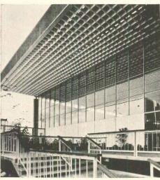
A chemical added during the papermaking process made the paper fire retardant, but, to make sure, the finished paperboard was treated again with fire-retardant paint. The double treatment paid off, and the ceiling passed all requirements, including a blowtorch test.
