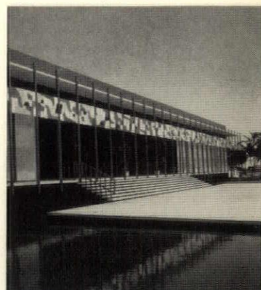
FLORIDA LIBRARY. The West Palm Beach Public Library is startlingly unlike most U.S. public libraries: it looks like a live building designed by a living architect. The concrete frame has a curtain wall of aluminum framing, porcelain enamel panels, and gray glass. Set behind a pool, it is ringed by a narrow gallery and a handsome mural designed by the architect, Norman N. Robson. Landscape architect: Robert L. Neal. Contractor: W. G. Lassiter, Inc. Cost: $350,045.
