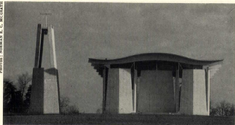
FLORIDA LIBRARY. The West Palm Beach Public Library is startlingly unlike most U.S. public libraries: it looks like a live building designed by a living architect. The concrete frame has a curtain wall of aluminum framing, porcelain enamel panels, and gray glass. Set behind a pool, it is ringed by a narrow gallery and a handsome mural designed by the architect, Norman N. Robson. Landscape architect: Robert L. Neal. Contractor: W. G. Lassiter, Inc. Cost: $350,045.
