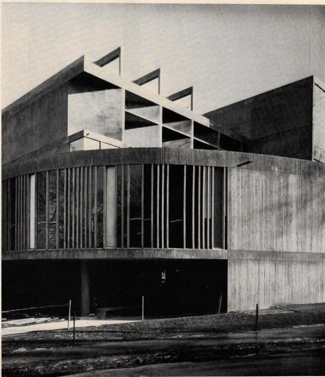
Three-dimensional studio-workshop on second floor has a curved glass wall divided by irregularly spaced mullions that follow Le Corbusier's Modulor scale. Below: same wall seen from outside.
