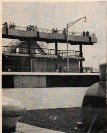
SEAWAY LOOKOUT. The shipshape look of this observation structure on the St. Lawrence Seaway at Massena, N. Y., results from a clean, straightforward use of steel. The three-level facility has a gift shop and snack counter at ground level, with a promenade deck on its roof overlooking the Eisenhower Lock. Twin stairs lead to the saw-toothed "flying bridge" (below), supported on six steel columns which form Y's. Architect: Daniel Chait & E. Slater. Contractor: John Rouse Construction Co. Cost: $203,780.
