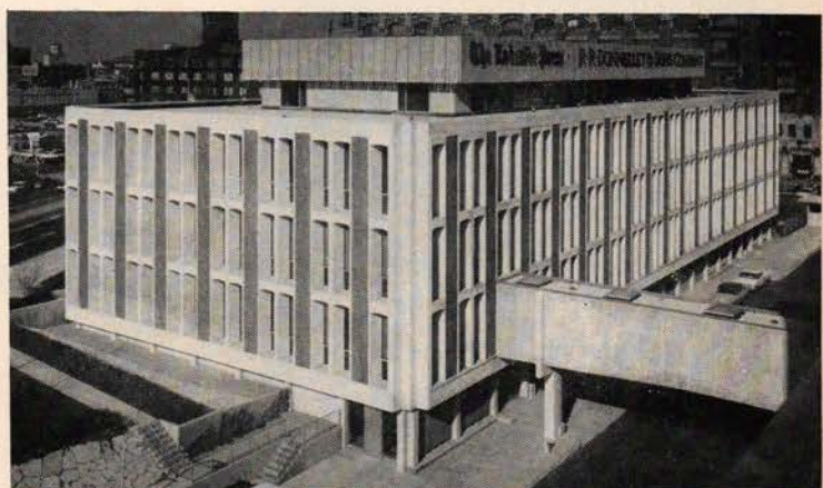
CHICAGO OFFICE. R. R. Donnelley & Sons' new publishing headquarters (above) was designed to harmonize with the firm's old buildings; it uses the same exterior brick, and windows are framed with precast concrete to recall nearby stone and terracotta trim. The deep windows control sun and leave space for riser ducts. Architects: Albert Kahn, Inc. Contractor: W. E. O'Neil Co. Cost: $2.5 million.
