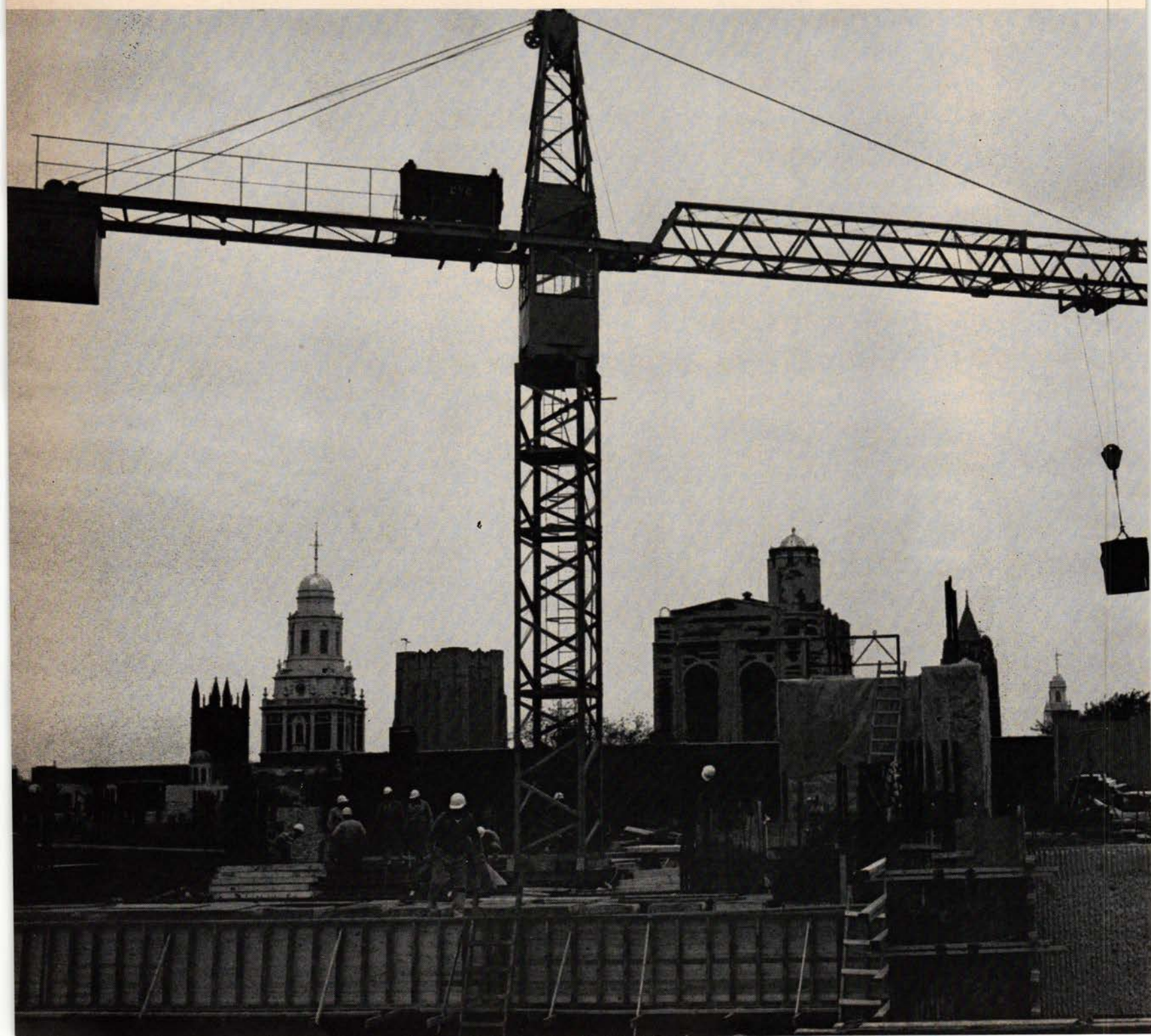
Below, a "hammerhead" tower crane atop the new Arts and Architecture Building at Yale swings a traveling bucket of concrete up to waiting workmen
